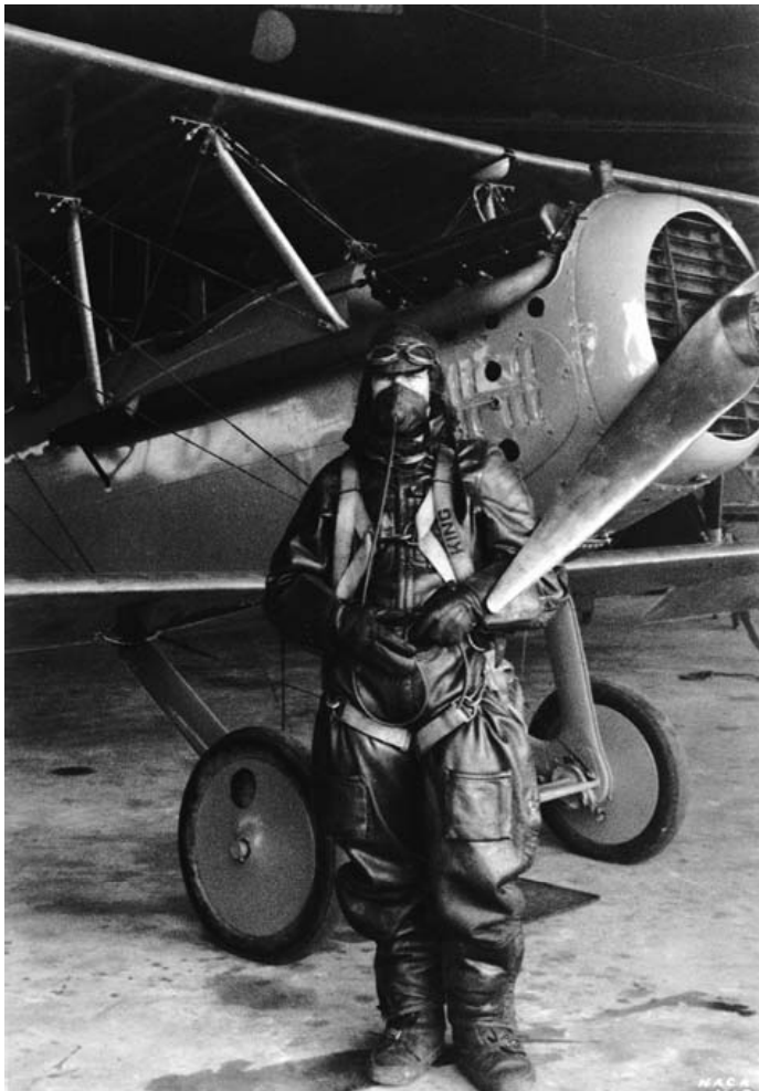
The higher one gets in the troposphere, the less dense the atmospheric gases, and the colder the air. This 1925 photograph shows a National Advisory Committee for Aeronautics pilot who is wearing a fur-lined leather flying suit with an oxygen facepiece for a test flight in this open-cockpit biplane. (Photograph GPN-2000-001380 courtesy of NASA.)
