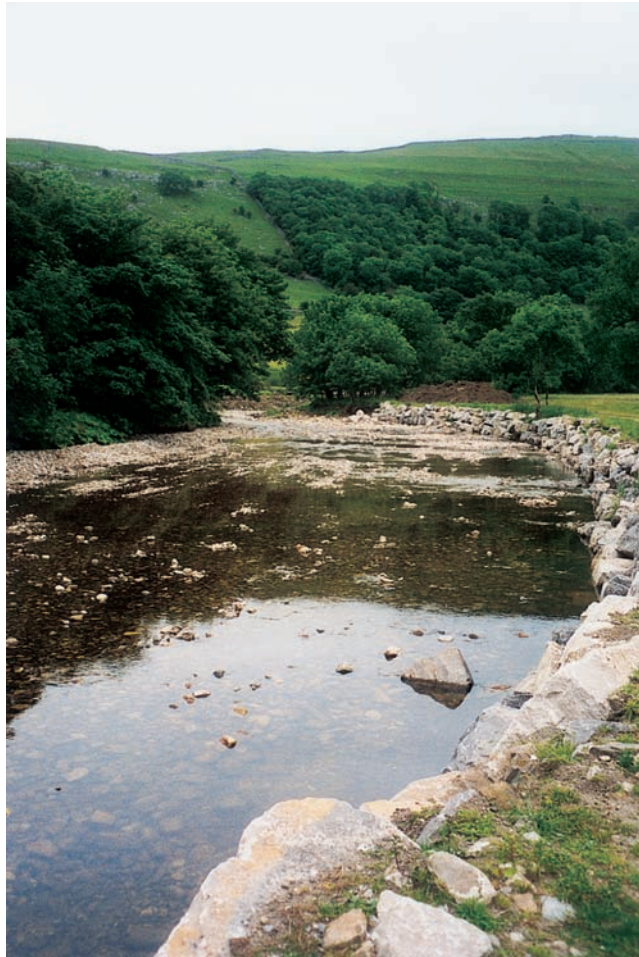
Figure 24.13 The gravel trap on the River Wharfe with bank protection.
