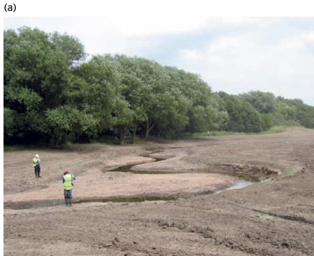
Figure 14.28 The re-meandered Sinderland Brook near Manchester, England, on the day after completion (a) and three months later (b). (Source: photo (b) courtesy of Charles Perfect)
