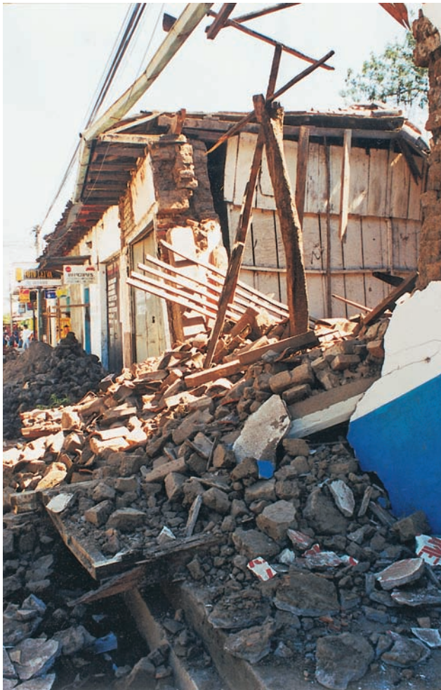
Figure 2.16 Photograph of the destruction of a building in El Salvador caused by an earthquake. (Source: photo courtesy of Dr W. Murphy)
