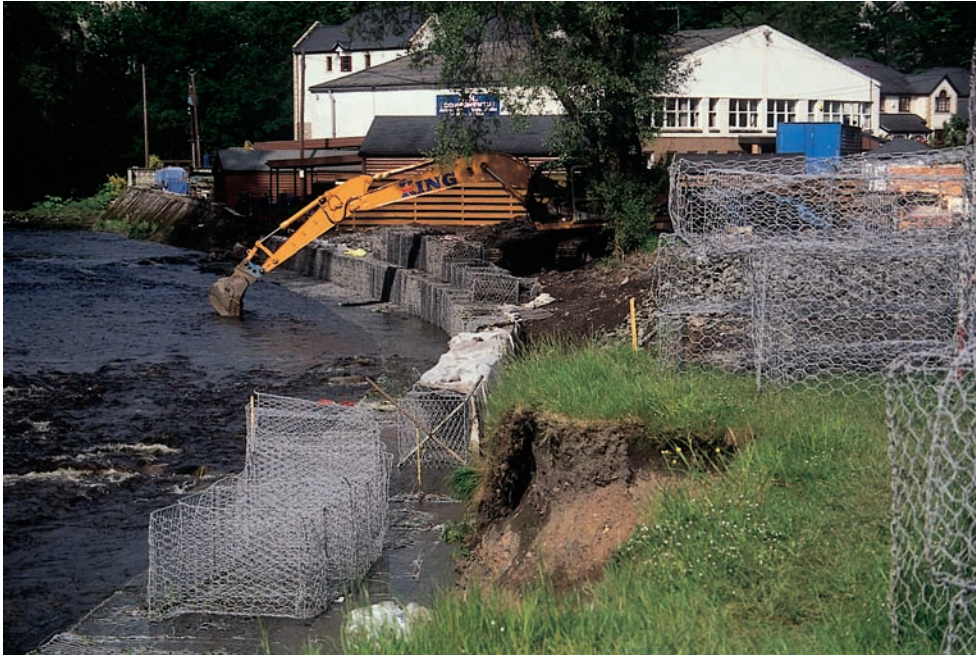
Figure 14.10 Gabion protection being used to stabilize a river bank adjacent to a new housing development aptly named 'Riverside' in Bridge of Allan on the Allan Water, Scotland.
