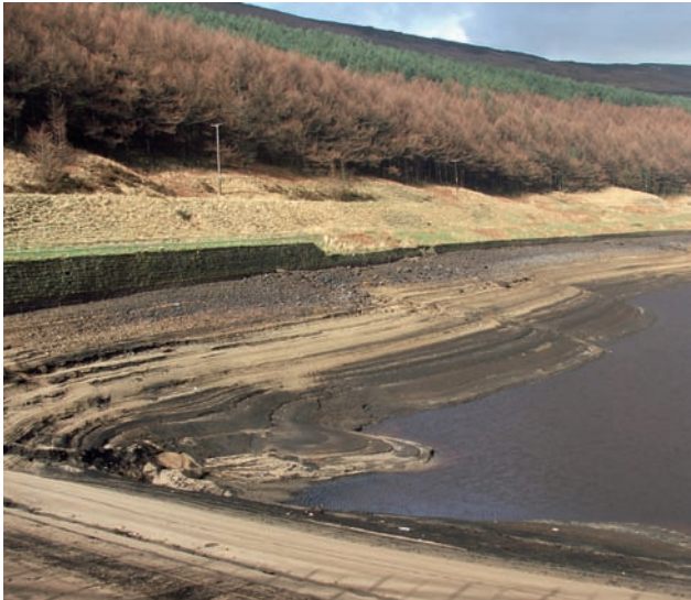
Figure 12.26 An upland water reservoir after drought conditions showing the layers of sediment that have built up. Such sedimentation reduces the capacity of these reservoirs.
