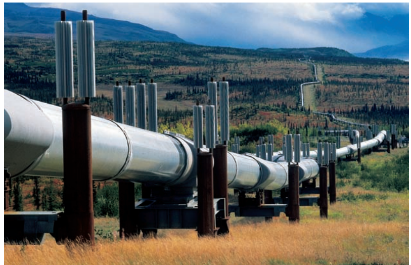
Figure 19.6 The trans-Alaska pipeline (heavy line): (a) the route of the trans-Alaska pipeline crosses both the continuous and discontinuous permafrost zones; (b) the design of the trans-Alaska pipeline allows it to move laterally and vertically with expansion and contraction. The supports are designed to prevent melting of the permafrost by the pipeline (source: T & P Leeson/Photo Researchers Inc./Science Photo Library).
