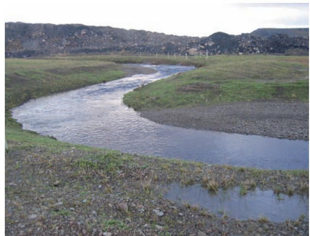
Figure 14.27 The River Nith diversion, south-west Scotland, showing its engineered morphology. The point bar features visible on inside of the meander bends were not engineered but developed over the first few flood events to flow through the diversion. The spoil behind is from a coal mine which lies beyond.
