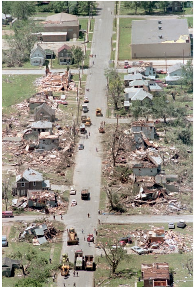
Figure 5.18 Damage to homes on the end of a cul-de-sac demolished by a tornado in Grandview, Missouri in 2003. (Source: Ron Kuntz/Corbis)
