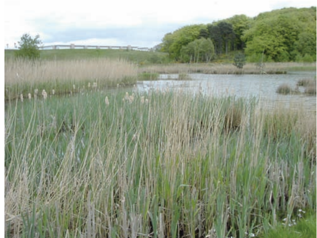
Figure 15.28 Example of a SUDS: a wetland and retention basin with a permanent water pool treating diffuse pollution from a residential and commercial development in central Scotland.
