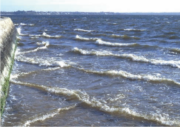
Figure 17.13 Reflection of breaking waves at the vertical face of a seawall giving rise to a criss-cross wave pattern.
