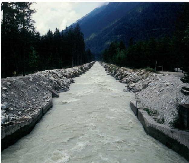
Figure 14.14 The Arve River between Argentiere and Chamonix in the French Alps following bulldozing and straightening.
