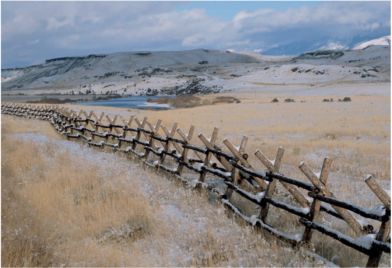
Figure 6.19 A snow fence acting as a shelter belt near a railway line across a grassland in the Rocky Mountains. (Source: National Geographic/Getty Images)
