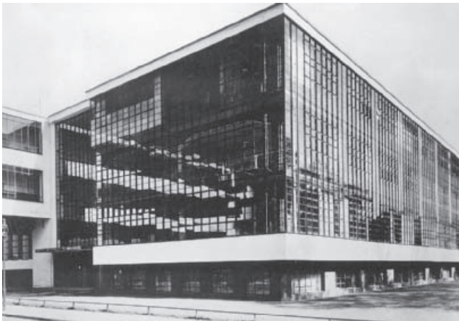
ARCHITECTURAL STYLE IN GERMANY BETWEEN THE WARS. The Bauhaus, by Walter Gropius (1883–1969). This school in Dessau, Germany, is a starkly functional prototype of the interwar “international style.”
