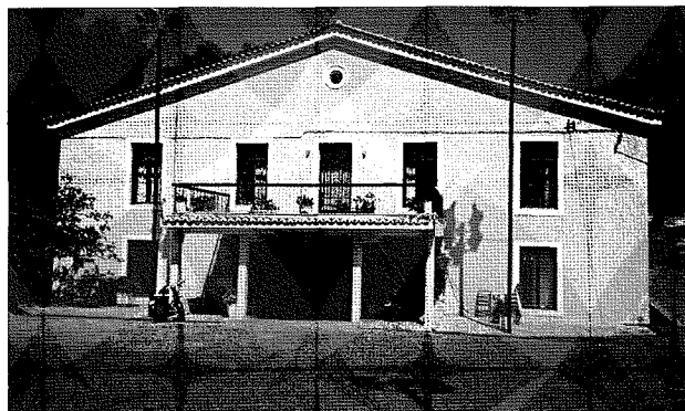
Fig. 221 The locker room for the first modern Olympics in 1896, constructed at the end of the tunnel entrance to the stadium, seen from the southeast (photo: author).
