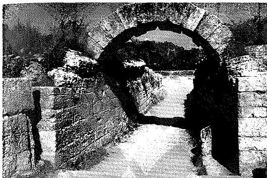
Fig. 175 The tunnel entrance (krypte esodos) to the stadium at Olympia. Originally constructed, with a narrower passage, in the 4th century B.C., the modern reconstruction of a small part of the vault is based on an ancient reconstruction of Roman times. The end of the Treasury Terrace wall appears at the extreme left (photo: author).
