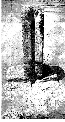
Fig. 59 Detail of the back of a half-column from the hysplex III system at Epidauros, viewed from the east. The vertical groove and its answering slot in the base held the hidden cords that released the barrier of the mechanism (photo: author).
