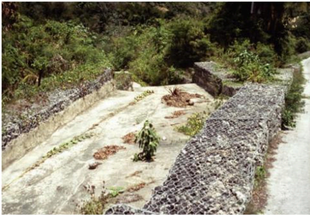
Figure 13.27 Gabions in Barbados
