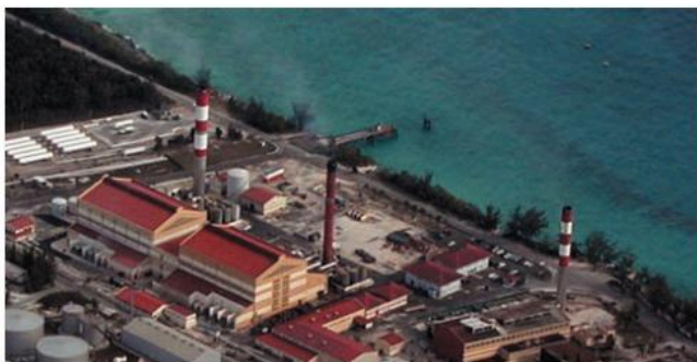
Figure 14.2 Clifton Pier diesel power station in the Bahamas
