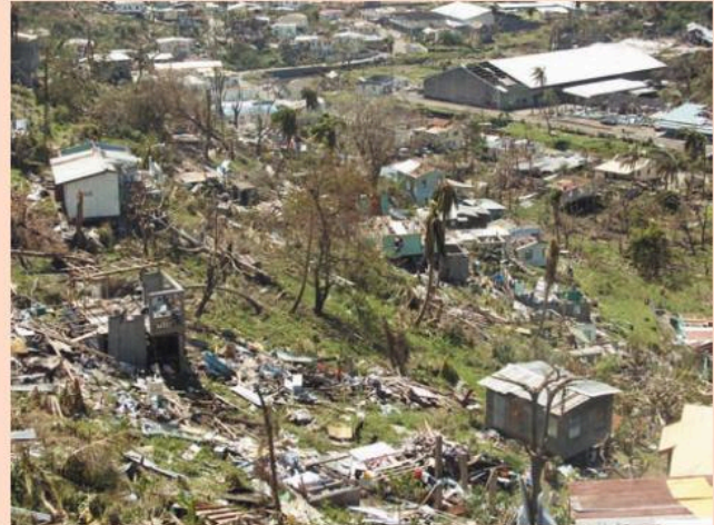
Figure 7.26 Destruction caused by Ivan
