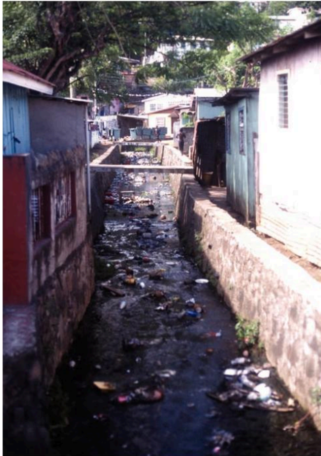
Figure 14.4 Open sewer in a shanty town outside Castries in St Lucia
