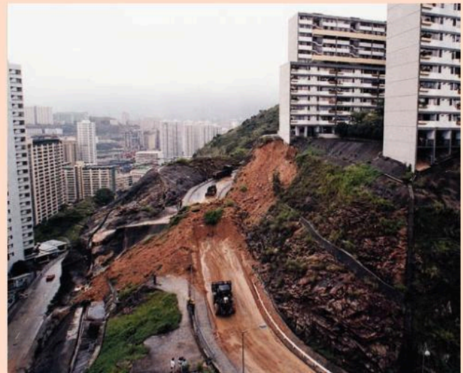
Figure 2.20 Consequences of a landslide in Hong Kong
