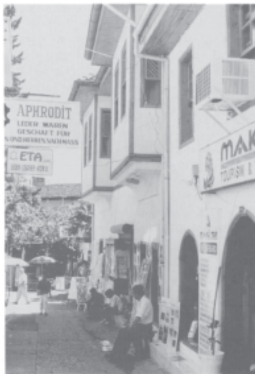
Fig. 6.7 (a) (right) Every piece of spare space is used for commercial activity in Antalya. (b) (overleaf) High ground-floor walls and small openings indicate 'privacy' in residential neighbourhoods, Bergama, Turkey.
