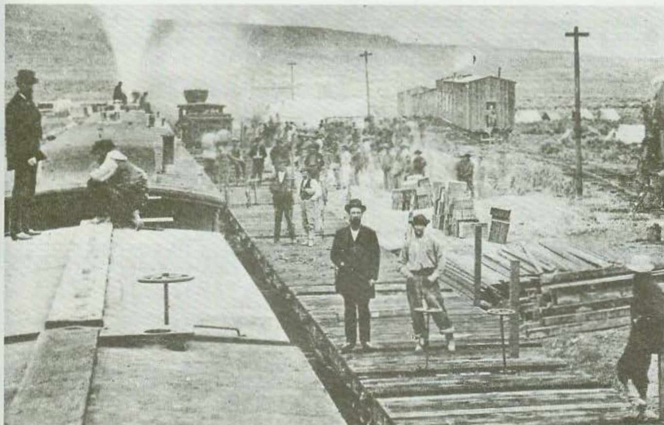
An all-time record for track construction in one day, April 28, 1863.
