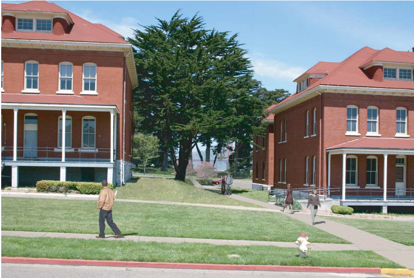
FIGURE 2: VIEW BETWEEN BUILDINGS 103 AND 104 FROM THE MAIN PARADE GROUND
