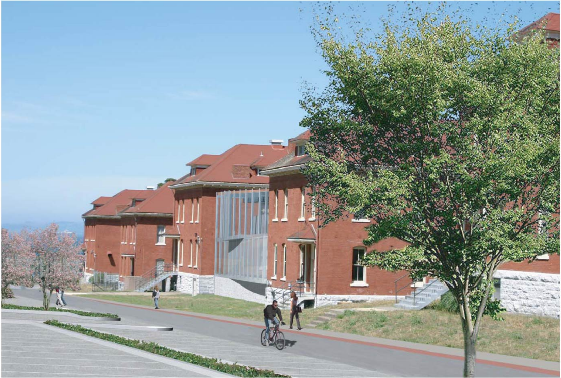
FIGURE 3: VIEW OF BUILDING 122 FROM TAYLOR STREET
