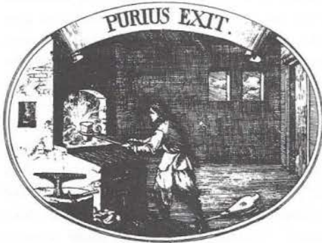
Gold purified in a smelting furnace. Hohberg, 1675
