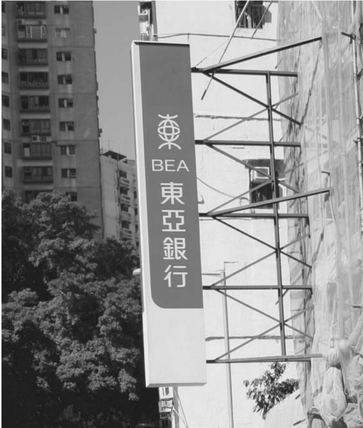
Figure C10.3 Bank of East Asia street sign
