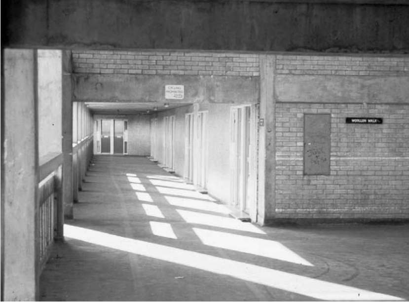
7.4 The so-called 'streets in the air' of the famous Sheffield housing schemes of Park Hill, Hyde Park and Kelvin. In reality they contain few of the social features of a real street in terms of the relationship of territories and defensible spaces. In practice they thus failed to offer the behavioural setting clearly in the minds of the architects
