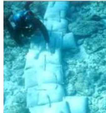
Application of cement bags
