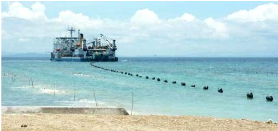
Figure II.2: Cable floated from the cable-ship to shore
