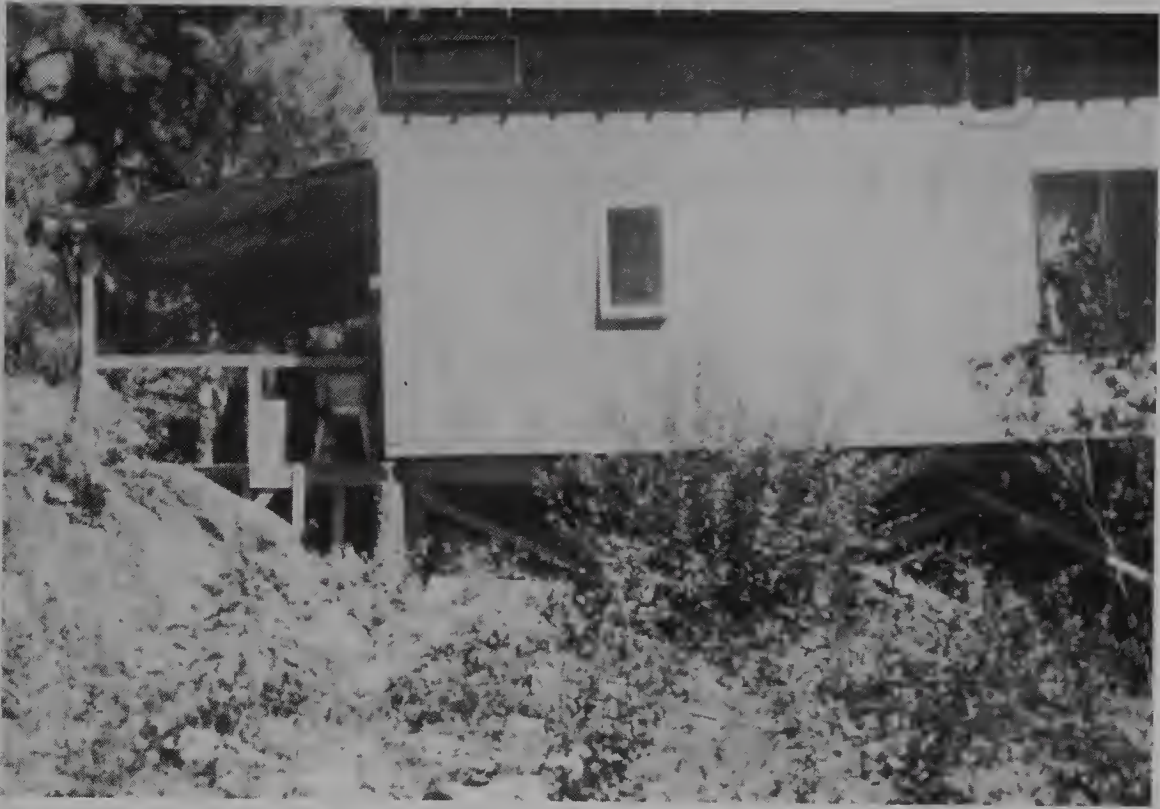
The Weaver cabin in the mountains of North Idaho in the summer of 1984, when it was completed. The cabin was built by Vicki and Randy with two-by-fours, plywood, and scraps from a nearby sawmill.
