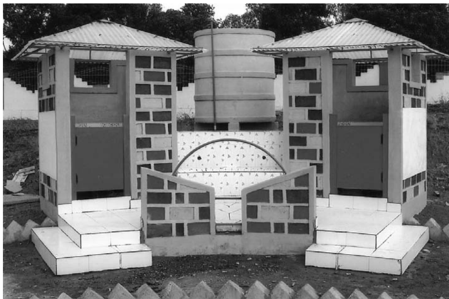
Figure 2.5 Child-friendly, barrier-free, cost-effective toilets at a children's park in Koraput
