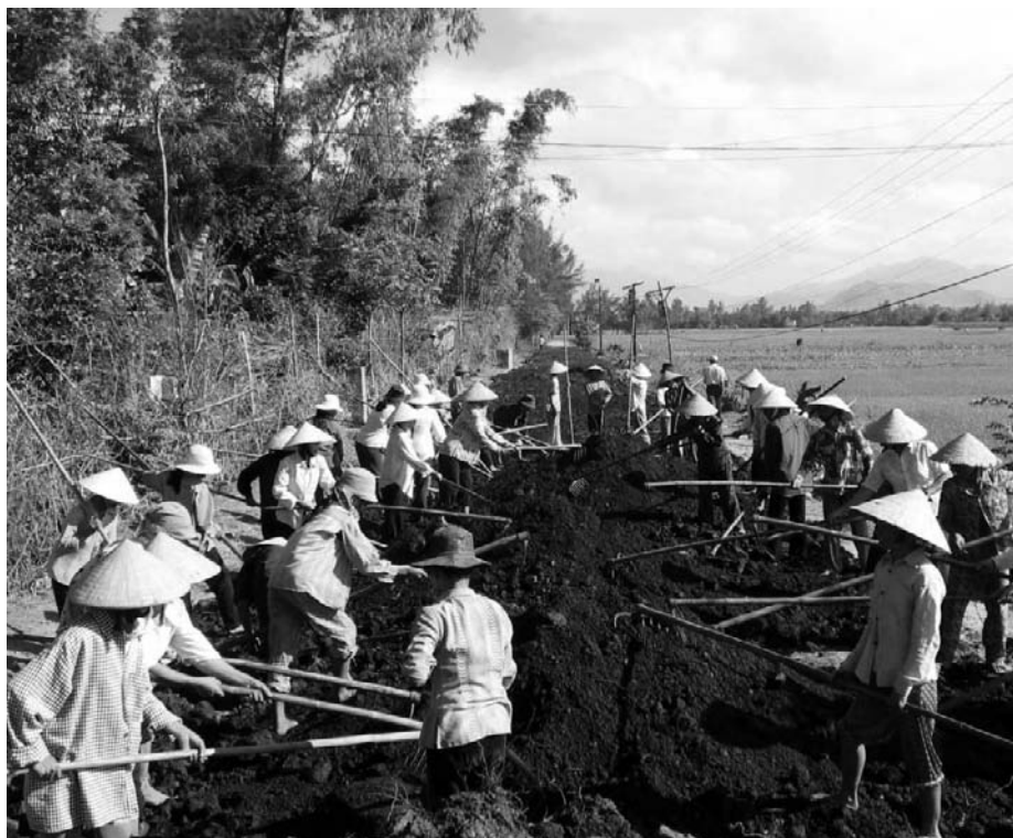
Figure 10.2 A road being built by commune members
