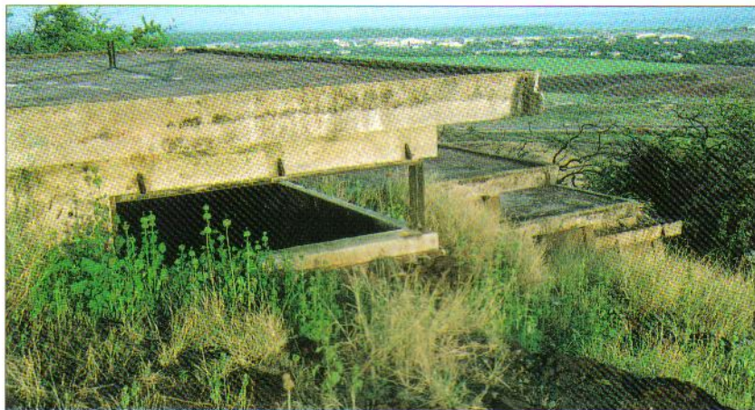
Fire control station "B" on the summit of Puu Palailai. This was a four-tiered building with stations staggered in echelon. The top station was the Battle Command Station; the others were secondary stations for batteries Williston, Closson, and Hatch. The first three stations were constructed in 1929, and the fourth (for Hatch) added in 1934. The site served through World War II, but is now abandoned. (TM)
