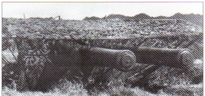
One of the mounts of Battery Kirkpatrick at Wiliwilinui Ridge. This is one of the few known photographs showing the dual 8in. gun mounts emplaced on Oahu in 1942. The mounts (strictly speaking they were not turrets, though the Army used the term interchangeably with "mount") were pretty much the only above-ground part of the structure: the other important rooms and magazines were underground. (NARA)
