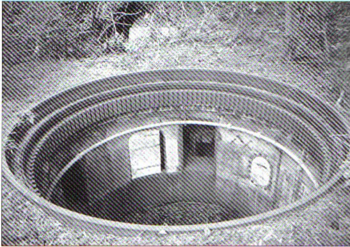
A 1994 photograph of one of the gun positions of Battery Kirkpatrick. The dual 8in./55cal. naval gun mount would have been emplaced on this base ring. (TM)
