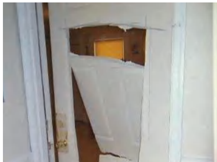
FBI agents used a chainsaw to enter a Fitchburg apartment.
