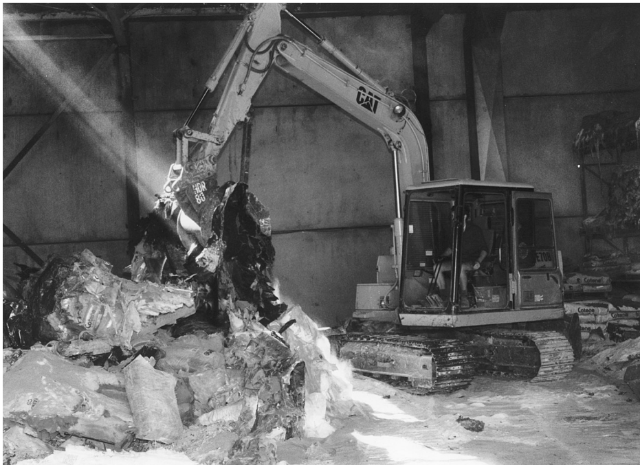
Figure 15.1 The clearing and searching of fire and/or explosion scenes requires individual assessment and appropriate action. However, in each situation, the potential for contamination and disturbance must be carefully considered. In this particular instance, the potential for sample contamination with petroleum products was high but unavoidable given the amount and nature of the materials which needed removal prior to the examination of the diagnosed fire starting point
