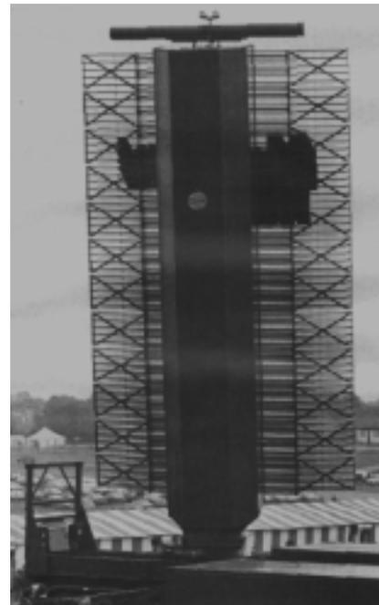
**Figure R65** Martello stacked-beam 3D radar. In this design, each row of elements has its own receiver front end, and an IF beam-forming matrix is used to generate the multiple elevation beams (Marconi Co. photograph).
