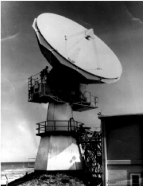
**Figure R34** AN/FPQ-6 instrumentation radar (RCA photo).
