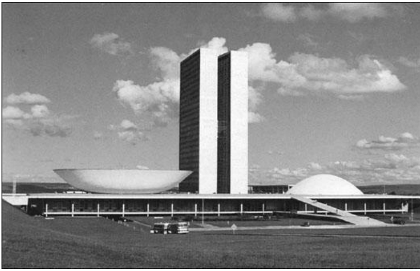
The Secretariat Building (c. 1956), Brasilia, Brazil, is a visually dramatic representation of the “two pillars,” Jachin and Boaz, attained by traversing the bridge entrance. On one side is the vessel or grail of enlightenment, on the other is the dome, sign of fertility of the goddess.
