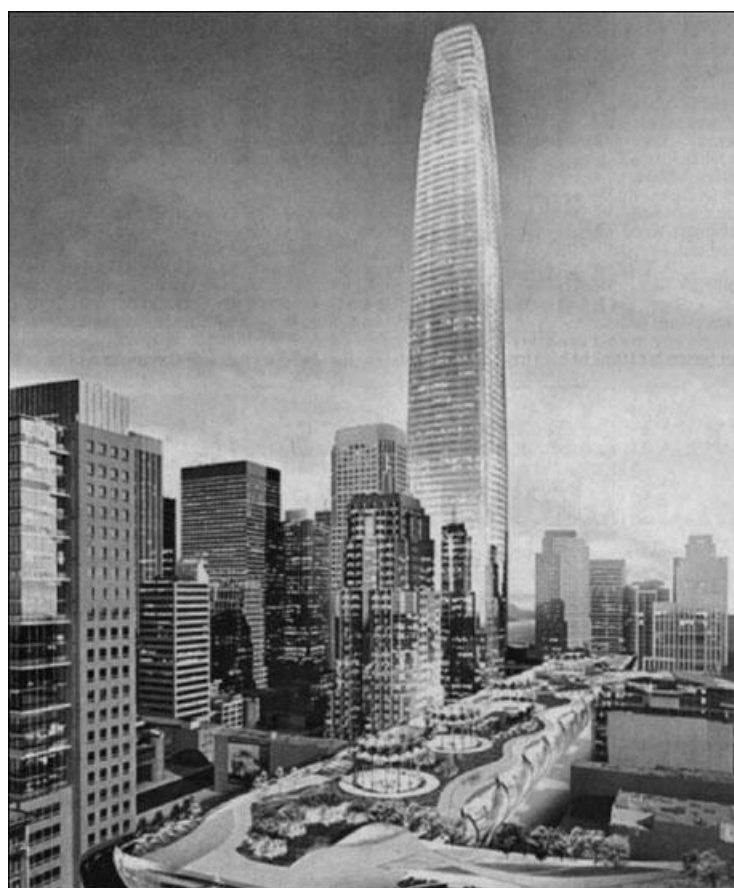
The billion dollar, Transbay Transit Center tower planned for San Francisco, California. When finished, the massive structure will be 400-feet higher than the Trans America Pyramid, which is now the city's highest.
