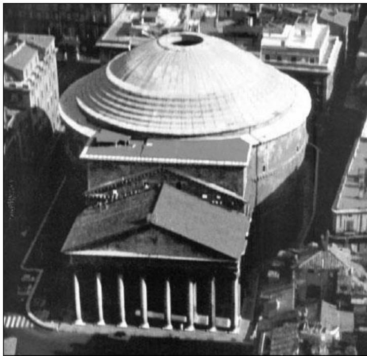
This view of the Pantheon in Rome reveals the huge opening in the middle of the dome through which sunlight streams into the circular-shaped sanctuary.
