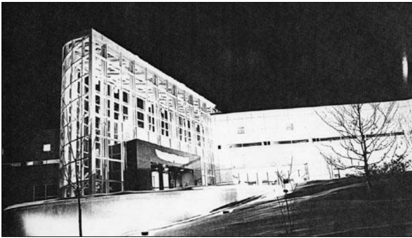
Exterior of main building, Fetzer Foundation World Headquarters.
