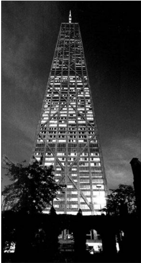
The John Hancock Center (c. 1969) in Chicago incorporated the “X” and Diamond repeatedly in its 1,127 foot tall structure.
