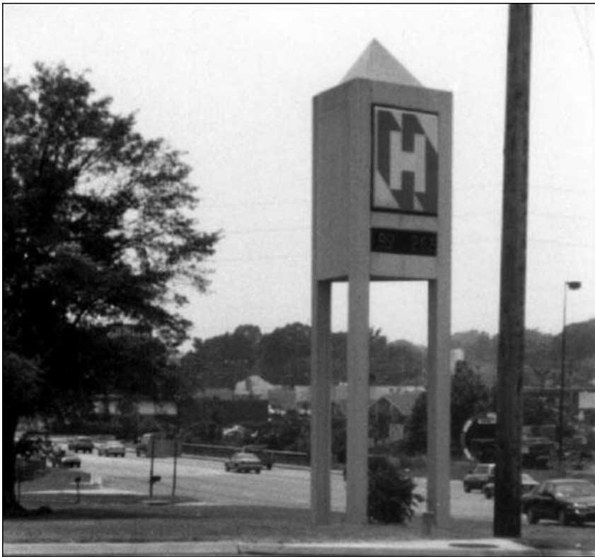
Hardwick Bank and Trust in Dalton, Georgia placed a pyramid atop its time and temperature sign. Why, no-one seems to know.
