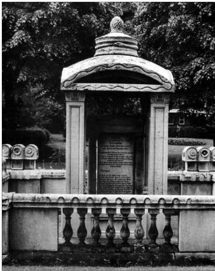
Mausoleum for Sir John Soane in St. Giles-in-the-Fields cemetery in London, near Old St. Pancras Churchyard. Note the acorn mounted on top, the oroboros serpent wrapped around the circular dome, and the bow or arch of Diana (Isis) with wavy lines engraved symbolic of the goddess' role of Aquarian age water-bearer and generatrix.
