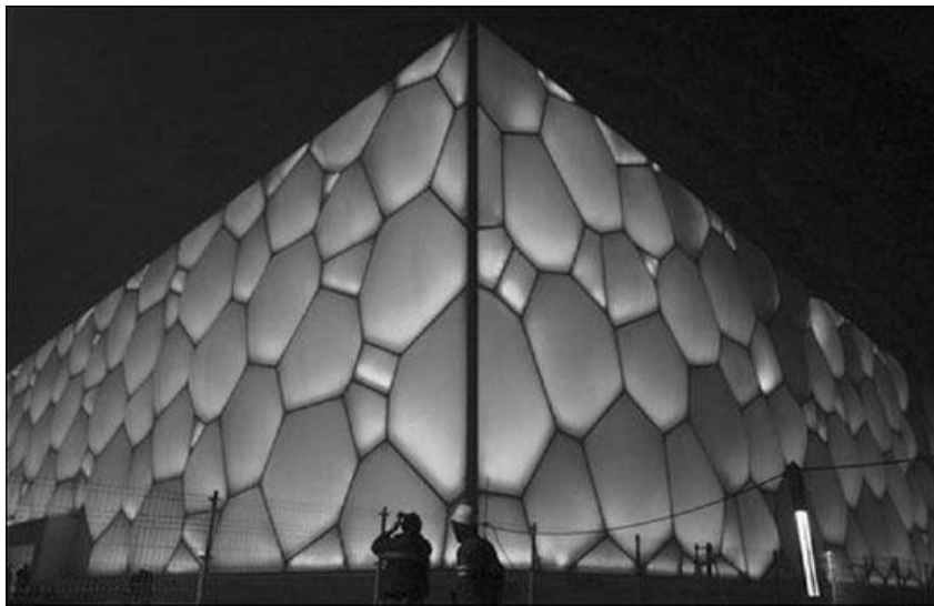
The much anticipated Olympic swim facility at the Beijing National Aquatics Center was built for the 2008 Olympic Games. Appearing to be a pyramid, the facility is actually shaped in the form of a cube.
