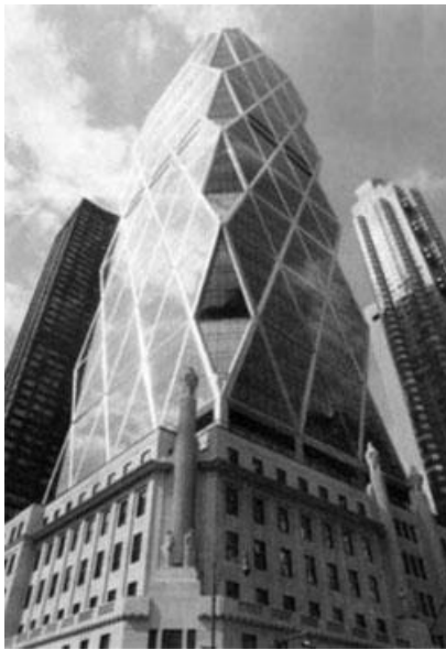
Hearst Corporation's new headquarters in downtown Manhattan (New York City) features an extension of glass diamonds and triangles atop a traditional base with statues and pillars.
