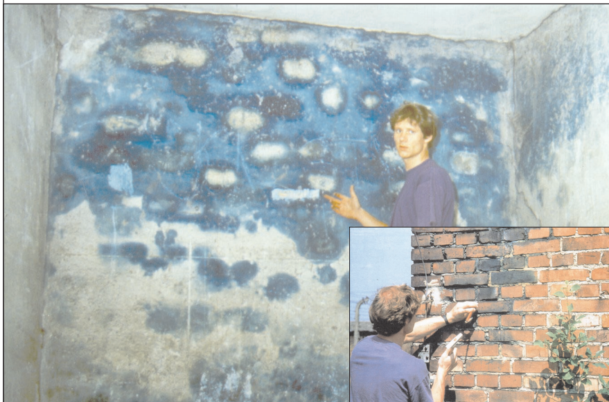
Color Illustration 3: Interior room of the delousing facility in the north-west part of Building 5a in concentration camp Auschwitz-Birkenau. Background and at right, the exterior wall is stained a deep blue by iron blue, caused by exposure to Zyklon B (HCN): At left, the wall (a later addition) is white and free of cyanide residue. Color Illustration 4 (inset): External wall of the delousing facility of Building 5a.
