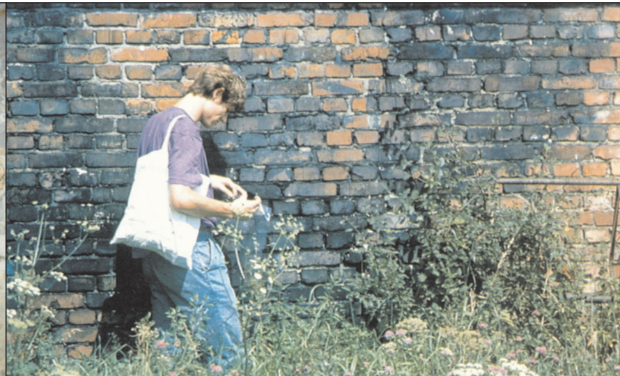
Color Illustration 2: Outside wall of the Zyklon B delousing facilities of Building 5b in concentration camp Auschwitz-Birkenau: discolored a deep blue by hydrocyanic acid that penetrated through the wall over time and reacted with iron to form the pigment. It has survived 50 years of weathering unscathed. Photos 1-4: © Rüdiger Kammerer
