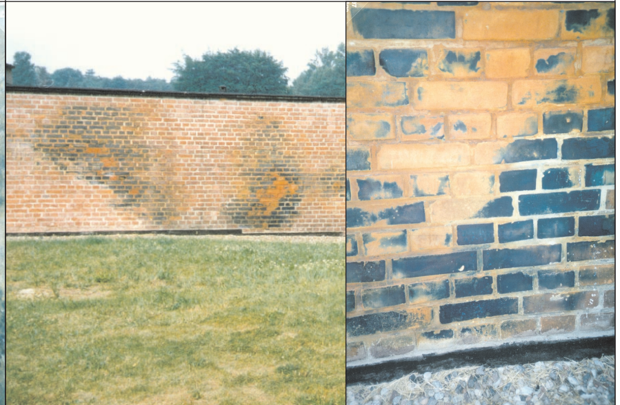
Color Illustration 9 (left): Blue staining on the exterior walls of the delousing gas chamber in concentration camp Stutthof. Color Illustration 10 (right): detail enlargement. © C. Mattogno
