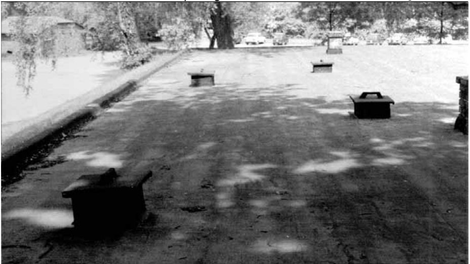
Document 23: Photo of the roof of the morgue. All four shafts constructed by the Poles after the war. © Carlo Mattogno
