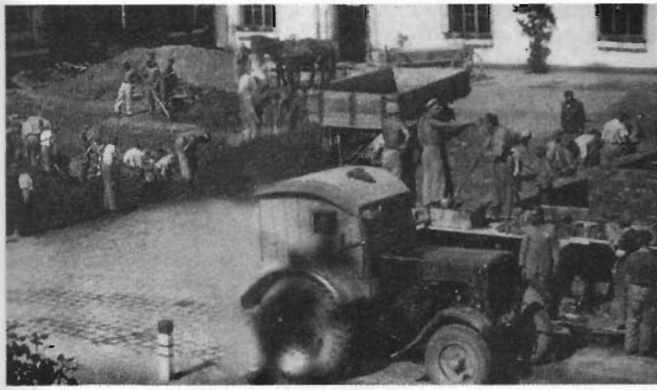
Photo 8 - 1943: (below) Workers doing renovations at the kitchen during early 1943. (Ref.: Auschwitz archives, Oswiecim, Poland).
