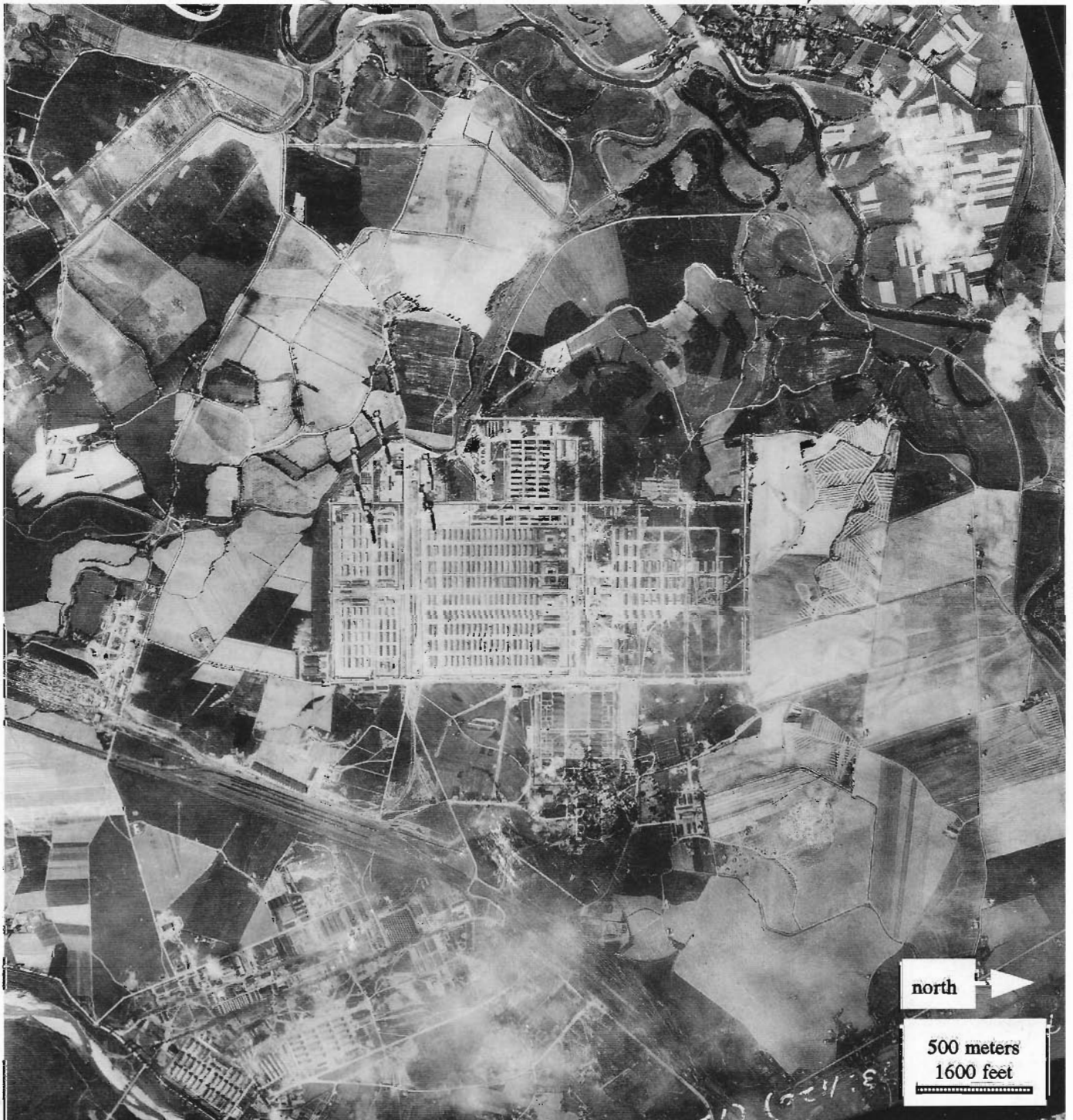
Photo 1 - September 13, '44 . (For now please discount the bombs falling directly over the camp) From the surrounding flat farmland, nine roads enter the Birkenau camp. There are no visible gatehouses, gates, or guardhouses on any of the many roads surrounding the camp. In the upper right corner across the Vistula River is the large village of Jedlina.
