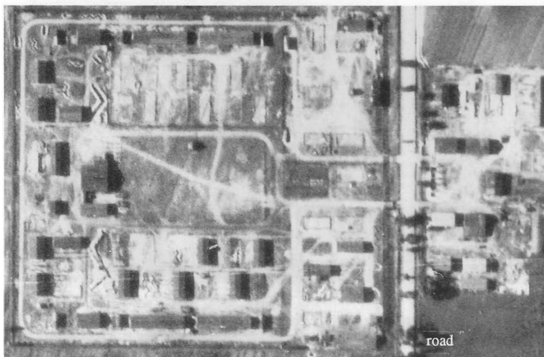
Photo 13 - Fall, '44: In the camp 26 buildings have been dismantled and 29 remain. The foundations of the dismantled buildings are visible. Scale: 2 Centimeters = 170 Meters or 1 inch = 700 Feet
