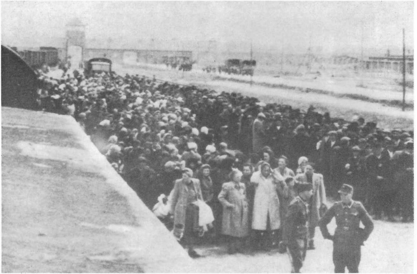
Photo 1 - Spring or summer, 1944: (above) Looking east from the unloading ramp towards the entrance gate in left background. (Ref.: Klarsfeld, S. Auschwitz Album).
