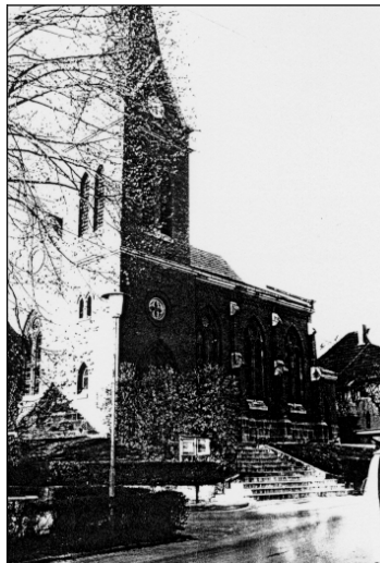
In August 1976, the Protestant church at D-96484 Meeder-Wiesefeld was fumigated with Zyklon B. Subsequently, blue-colored stains appeared all over the plaster.
