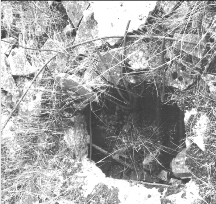
III. 26: Concrete roof of morgue 1 of crematorium II in Birkenau. Provan's opening 7 in July 1992. © Carlo Mattogno
