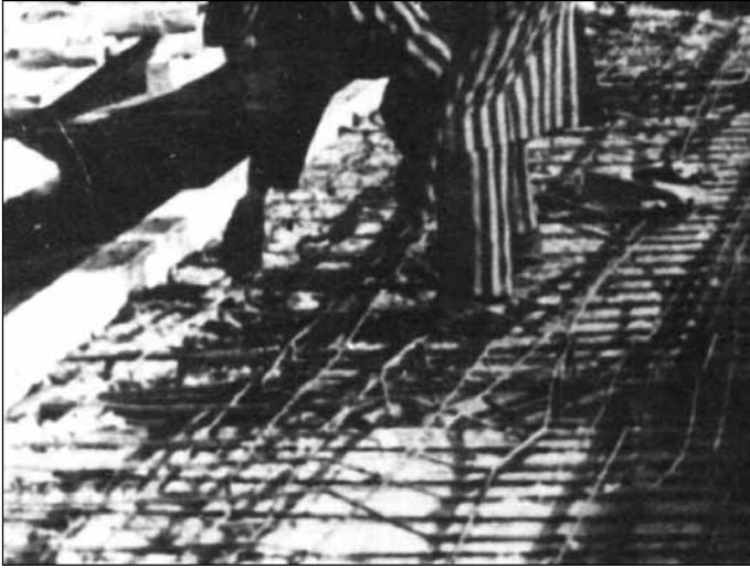
III. 15: Part of the reinforcement bars of the concrete roof of underground morgue 2 of crematorium II during construction. Photo published by J.-C. Pressac.
