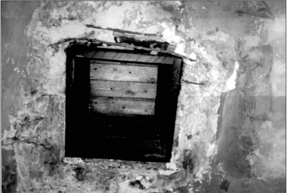
III. 13: Photo of the ceiling of the morgue. One of the four shafts constructed by the Poles after the war. © Carlo Mattogno.
