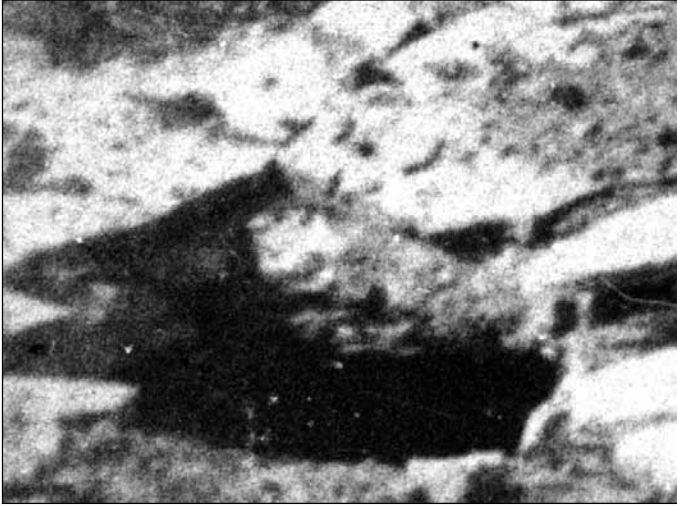
III. 19: Concrete roof of morgue 1 of crematorium II. Provan's opening 2 in June-July 1945. Section enlargement of photo 5.
