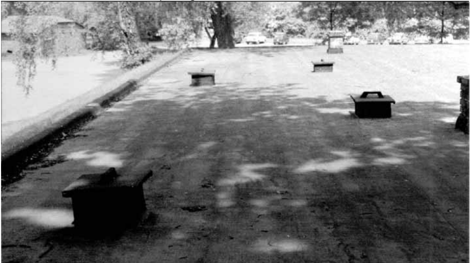
III. 11: Photo of the roof of the morgue. All four shafts constructed by the Poles after the war. © Carlo Mattogno.
