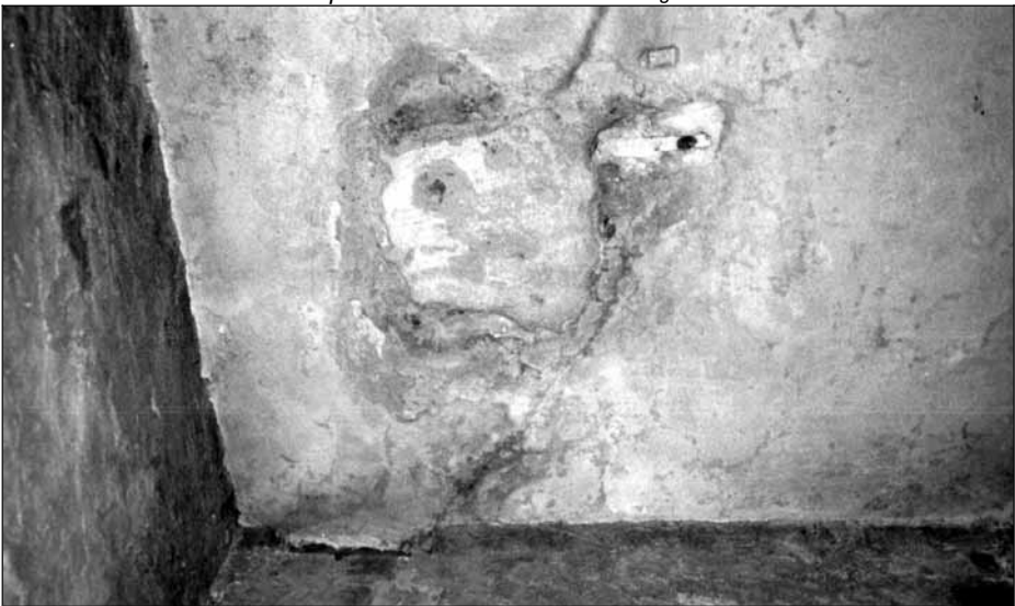
III. 7: Photo of opening no. 1 in the roof of the vestibule, part of the former morgue. © Carlo Mattogno.
