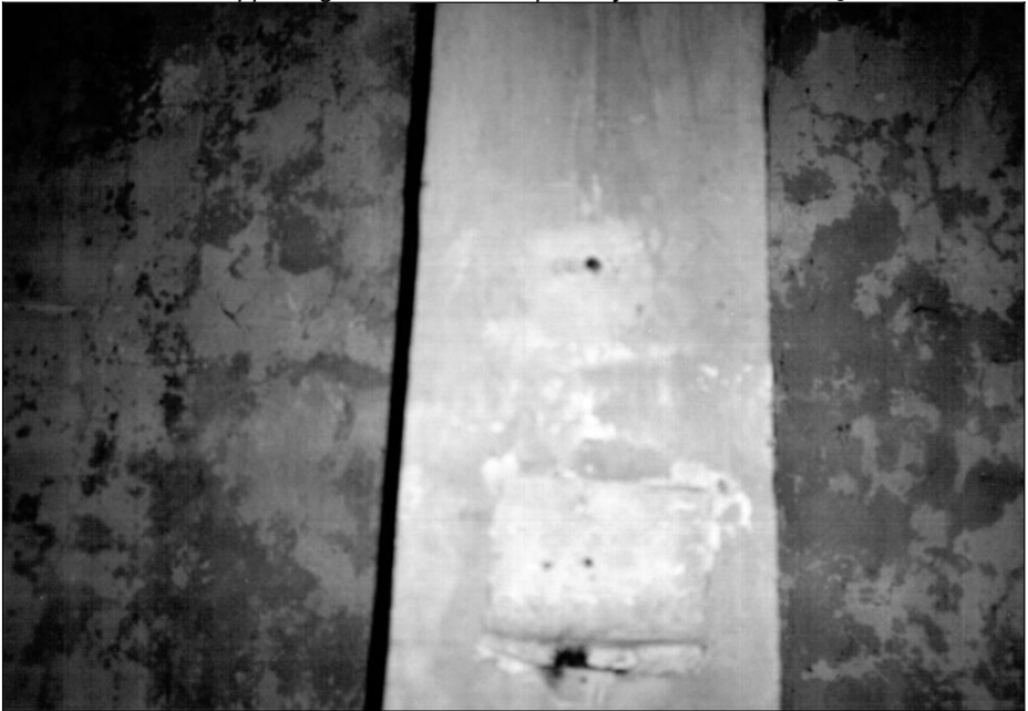
III. 12: Morgue of crematorium I at Auschwitz. One of the blocks set into the center of the supporting beam of the ceiling. October 1991. © Carlo Mattogno.
