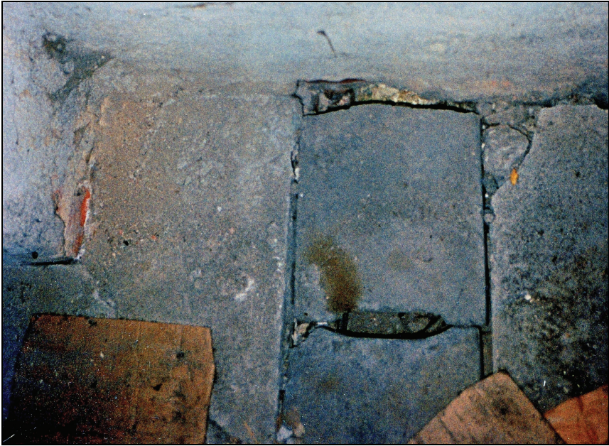
Document 16: Water run-off in floor of gas disinfestation chamber in BW 5a at Birkenau. © Carlo Mattogno.
