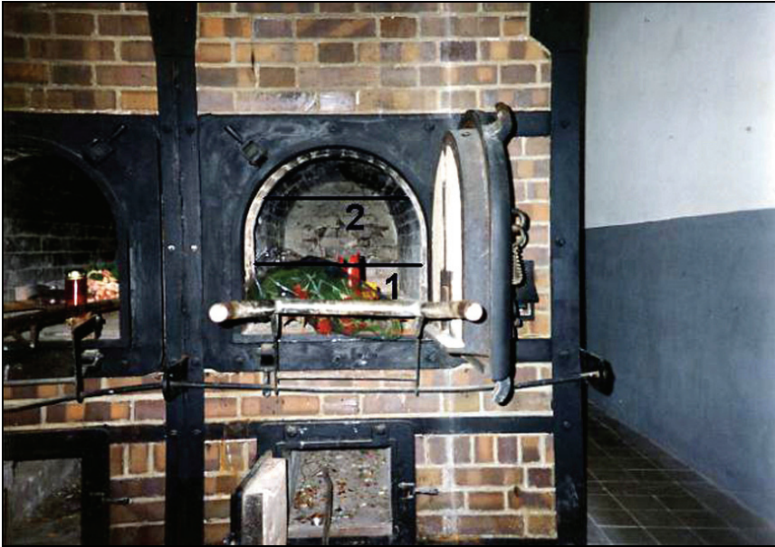
Document 46: Crematorium of Mauthausen. Topf coke-fired double-muffle oven Auschwitz type. (Cf. document 43). The two horizontal lines represent the height of two superimposed normal corpses on the muffle grid.
