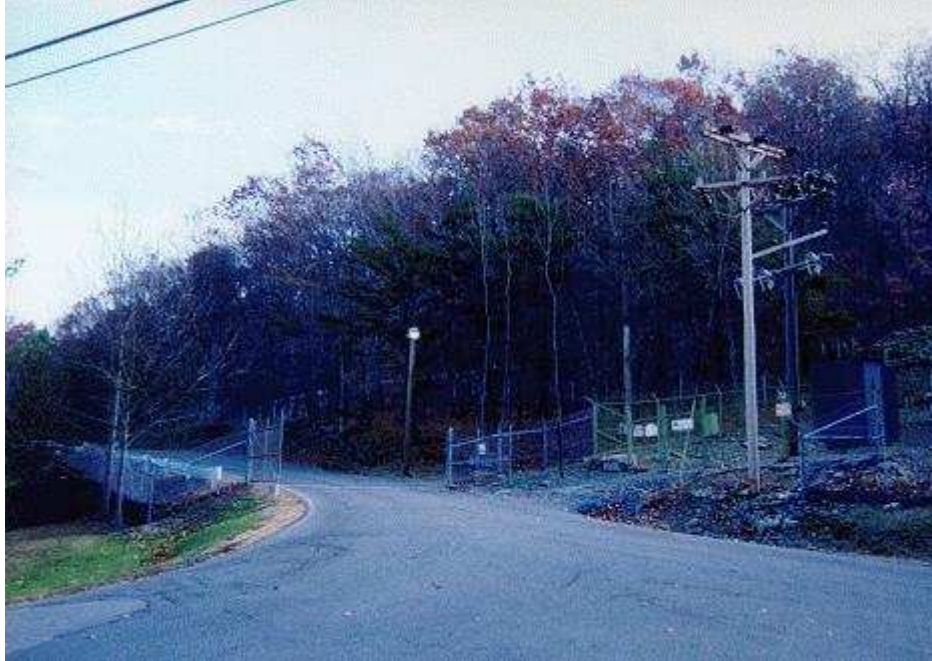
Main entrance to Raven Rock
