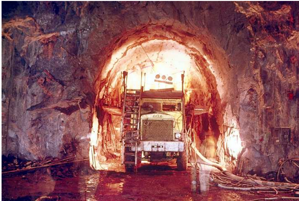
Cheyenne Mountain construction
