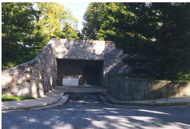
Entrance to bunker at Stephen P. Mather Training Center
