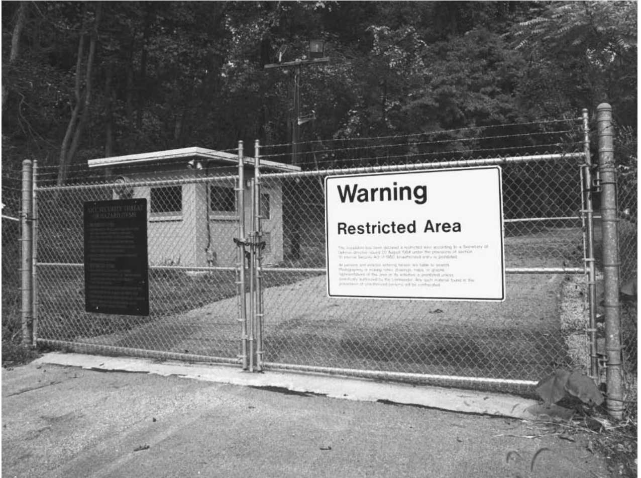
A view of chain-locked gates leading to an area of critical infrastructure, the underground Pentagon near Founatin Dale, Pennsylvania. The facility was built inside a mountain as a second central command structure if needed during wartime. AP/WIDE WORLD PHOTOS.
