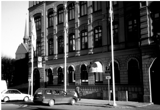
Seven floors under Johannes fire station is the SOS-centre
