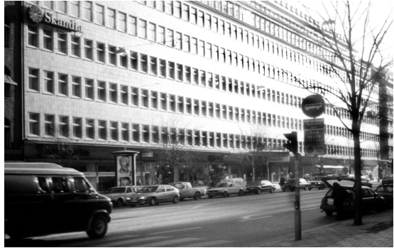
The Skandia building – secret HQ of Stay Behind
