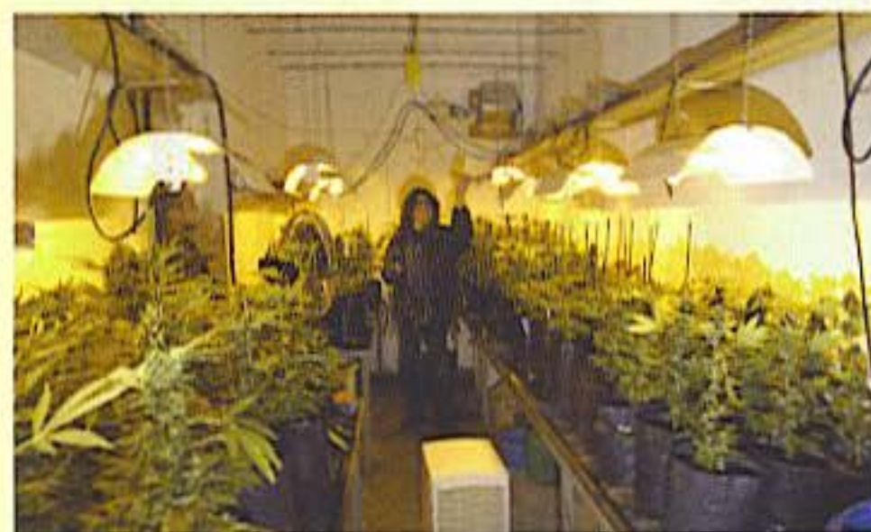
Place ballasts up on shelves so they stay out of the way and out of the splash-range of water.
