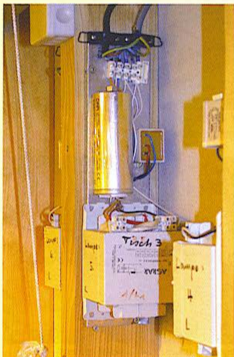
Attach ballasts to the wall so they are out of the way in the garden.
