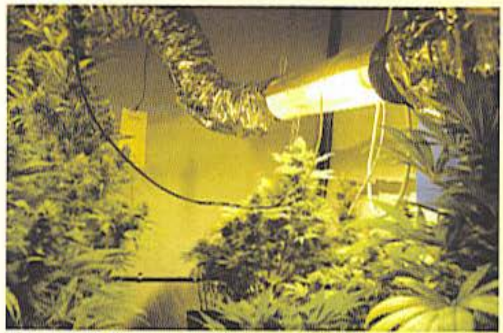
Air-cooled fixtures use blowers to direct heat generated by the bulb out ducting.
