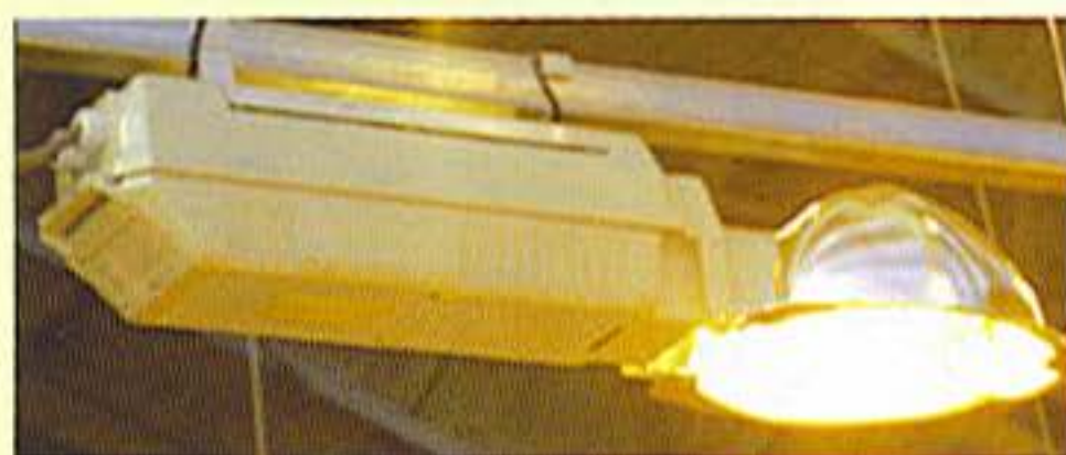
The ballast is attached to the bulb and reflective hood in this greenhouse fixture.
