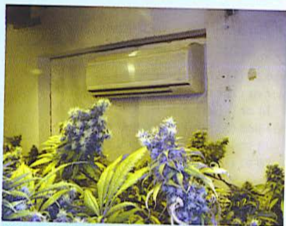
Air conditioners cool and dehumidify grow rooms. Growers must weigh the benefits against the extra electricity they use.
