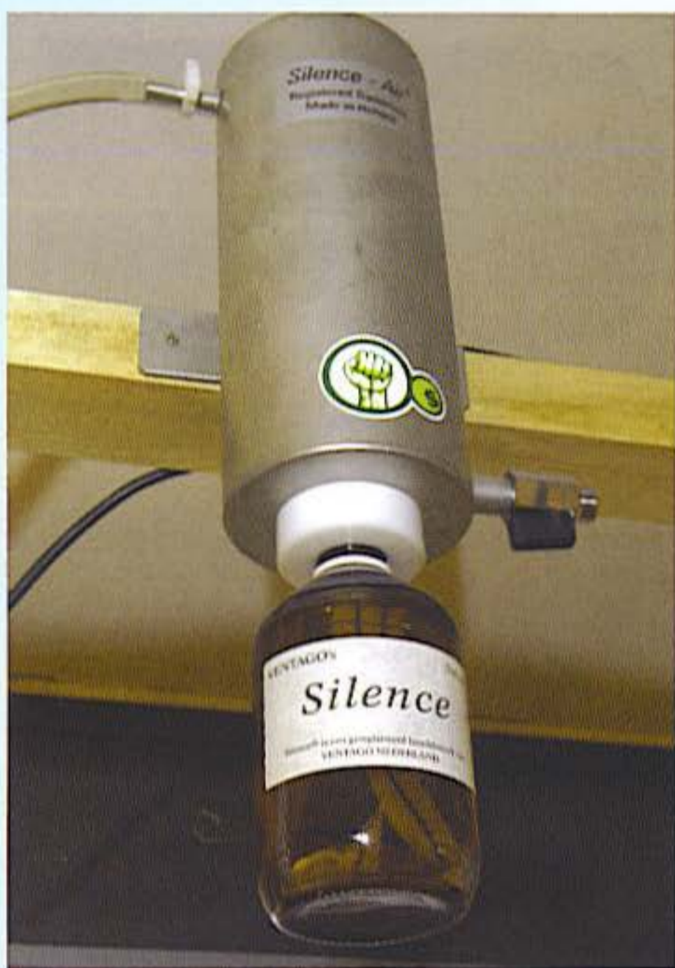
A vent-fan duct hooks to each tube, and the air-cleansing agent is imparted before air is evacuated.
