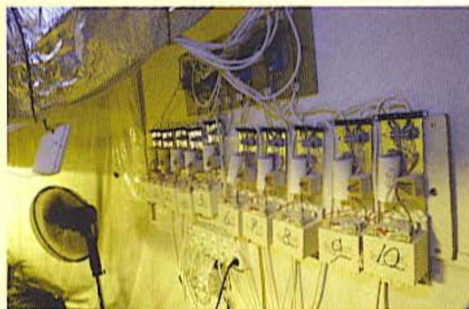
Attach ballasts to the wall on a plank for easy inspection and troubleshooting.
