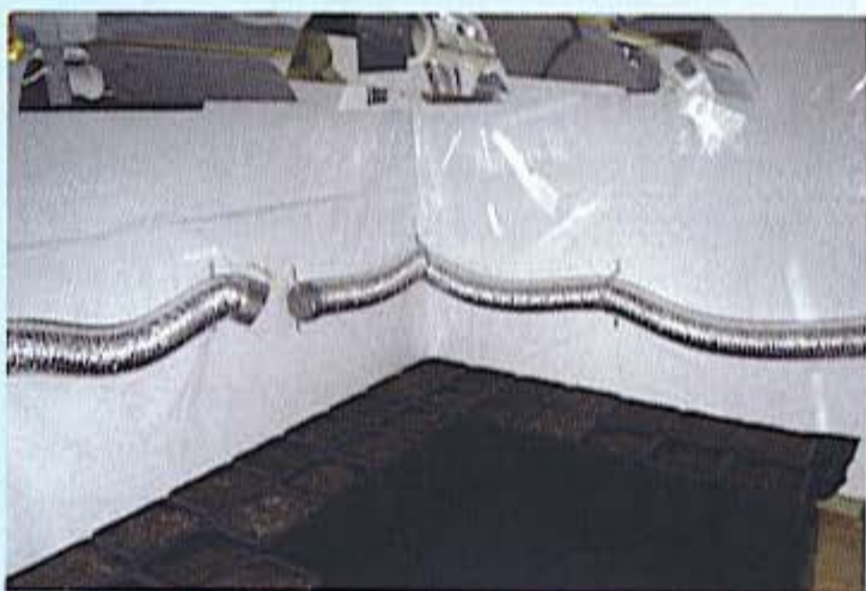
Fresh air in this room is piped in directly where plants need it.
