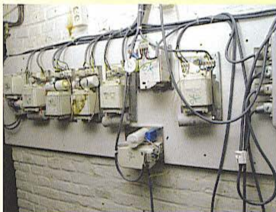
The timer on the right controls the entire lighting system in the grow room.
