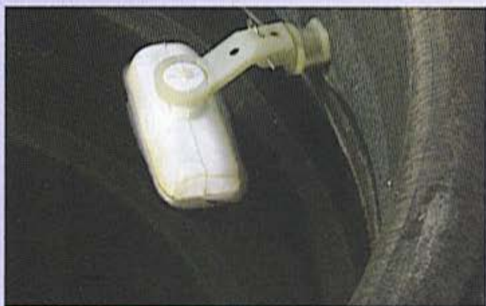
A float valve will turn water on to fill the reservoir when the level drops.
