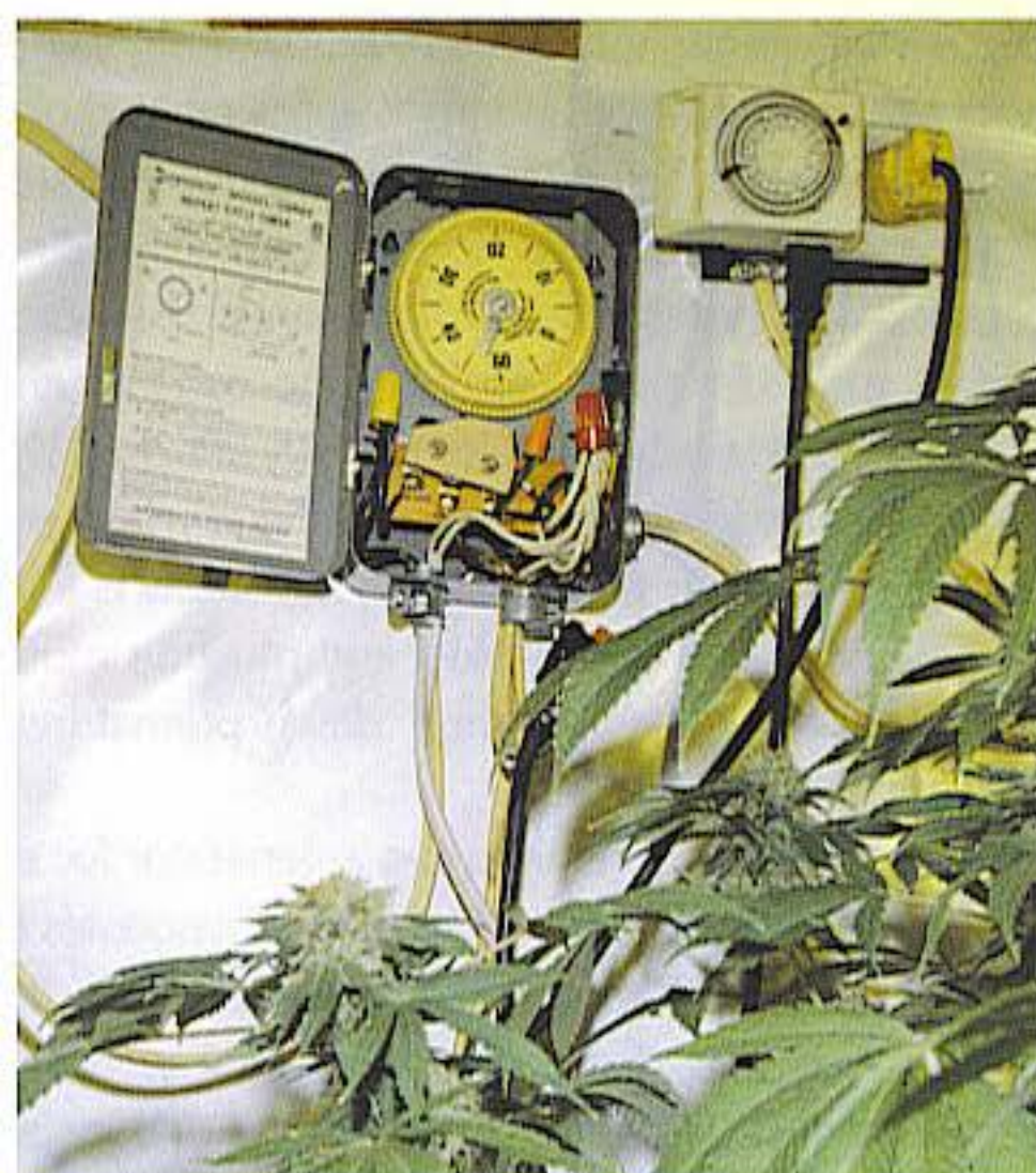
The mechanical timer on the left will operate several lamps at the same time. The digital timer on the right operates a single 1000-watt HID.
