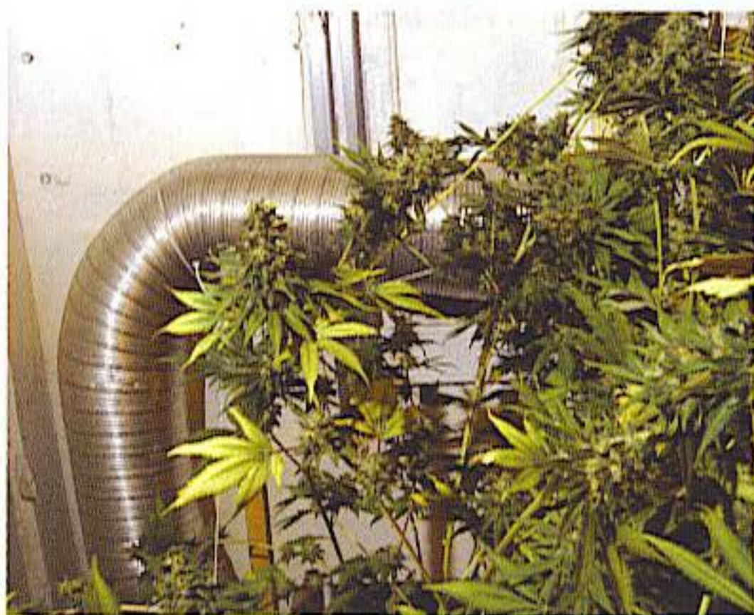
Air flow and volume are diminished when they turn corners.
