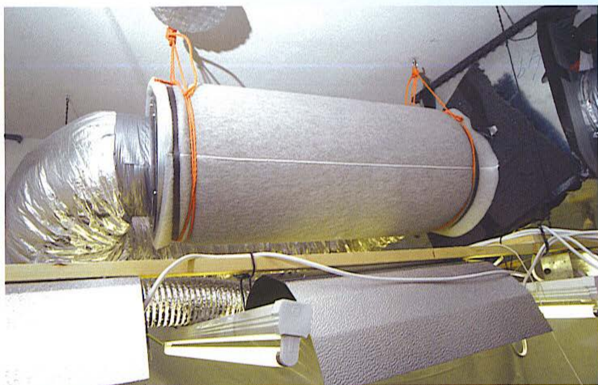
Charcoal filters remove fragrance and pollen from the air. The model shown above has a half-inch outer filter that encases porous ducting surrounded by activated charcoal. These filters are efficient until humidity climbs beyond 60 percent, at which point moisture-filled charcoal fails to absorb.
