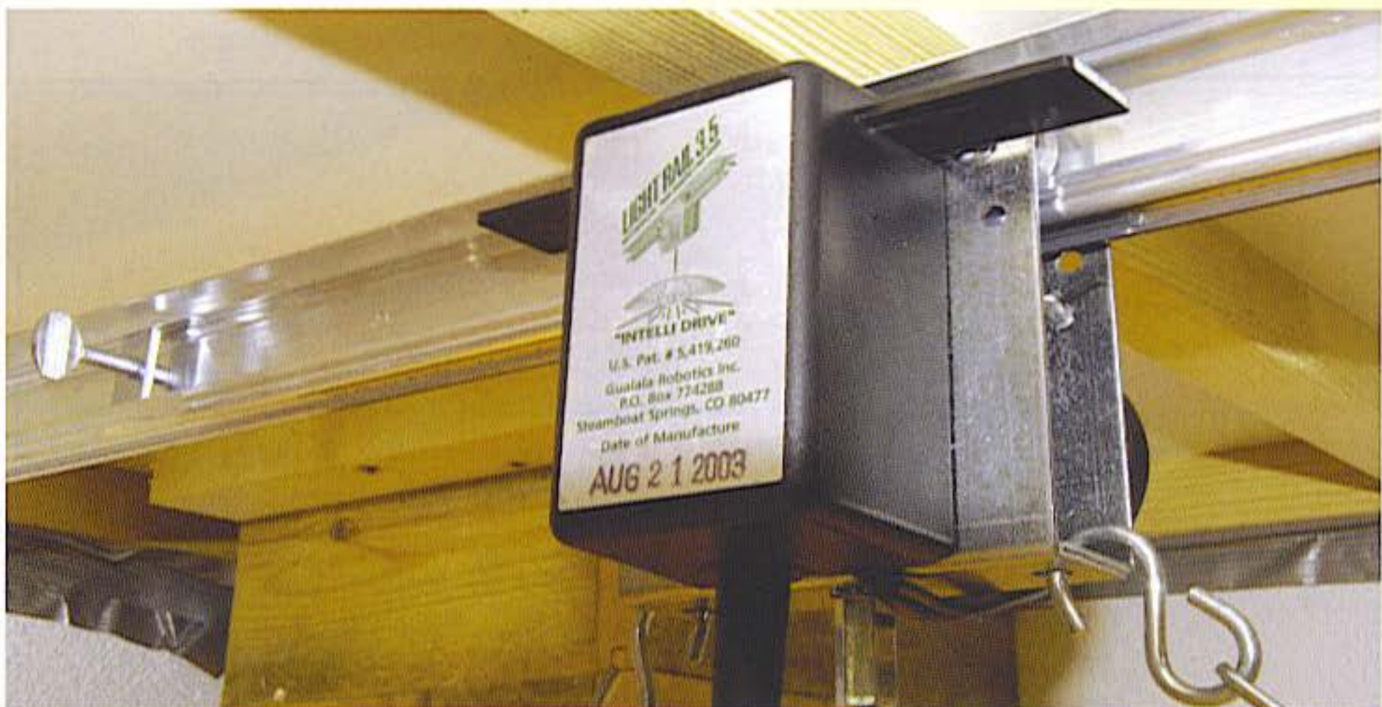
Reliable linear light movers offer an exceptional value to indoor growers. Light intensity increases exponentially when bulbs are moved closer to the garden using a light mover.
