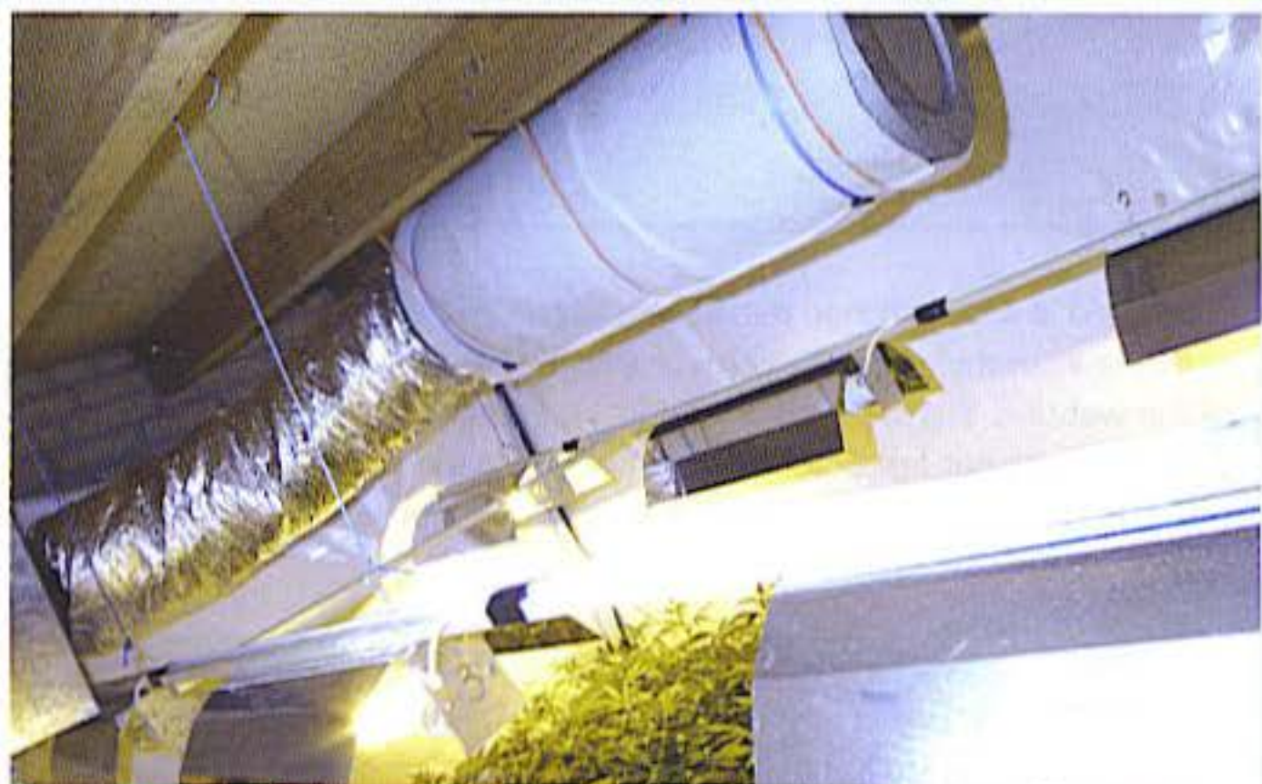
A carbon filter will remove the fragrance of cannabis before expelling grow room air.
