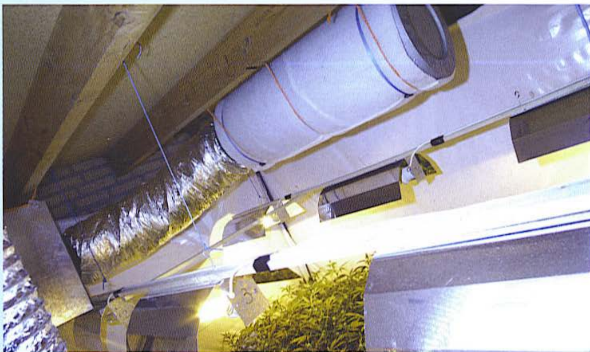
An activated charcoal filter is attached to a vent fan. The air is cleaned before leaving the grow room.
