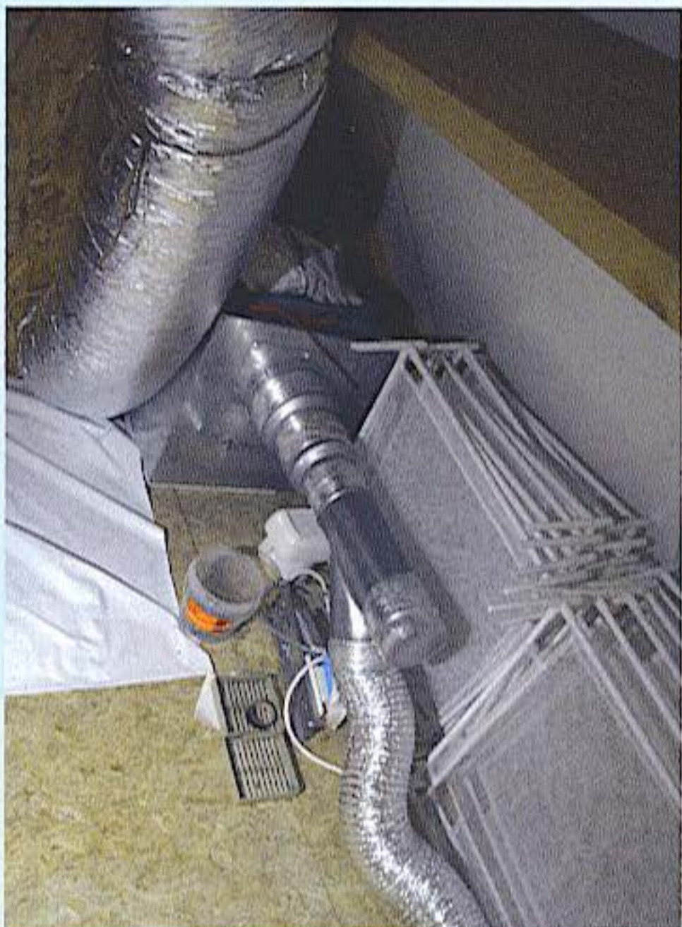
This grower treats the air with ozone and deodorizes air again just before it is expelled.
