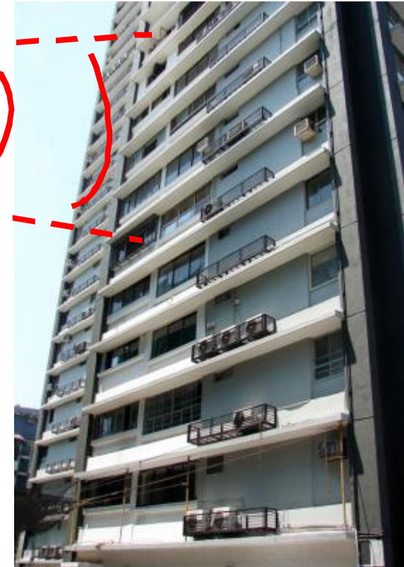
Usha Kiran Building
