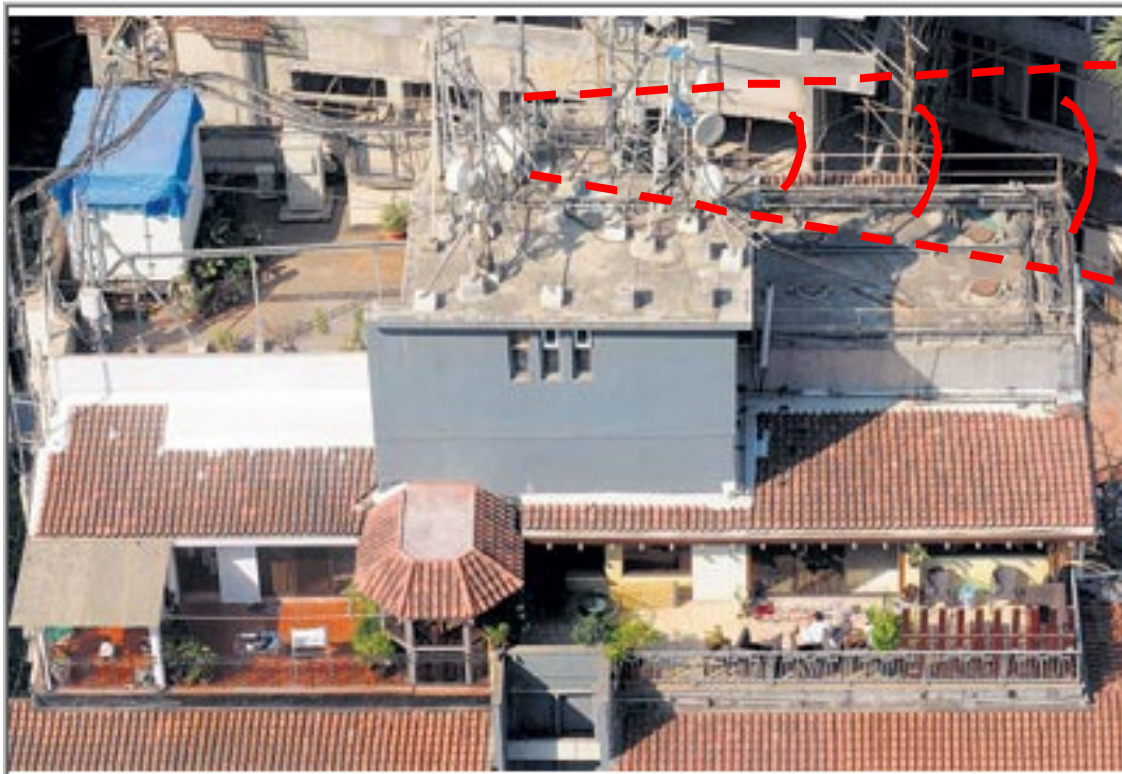
The cell phone towers installed on the Vijay Apartments terrace at Carmichael Road pic/Bipin Kokate
