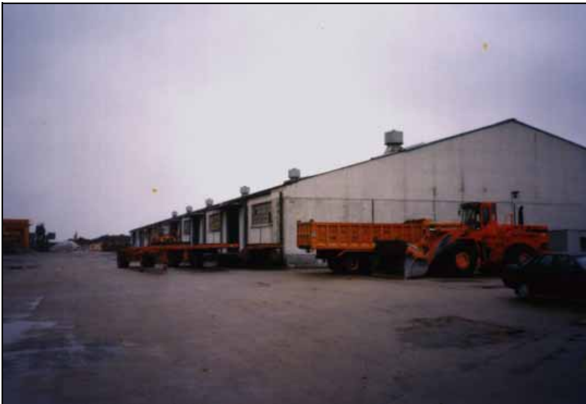
Warehouse Inland of Pier 1
