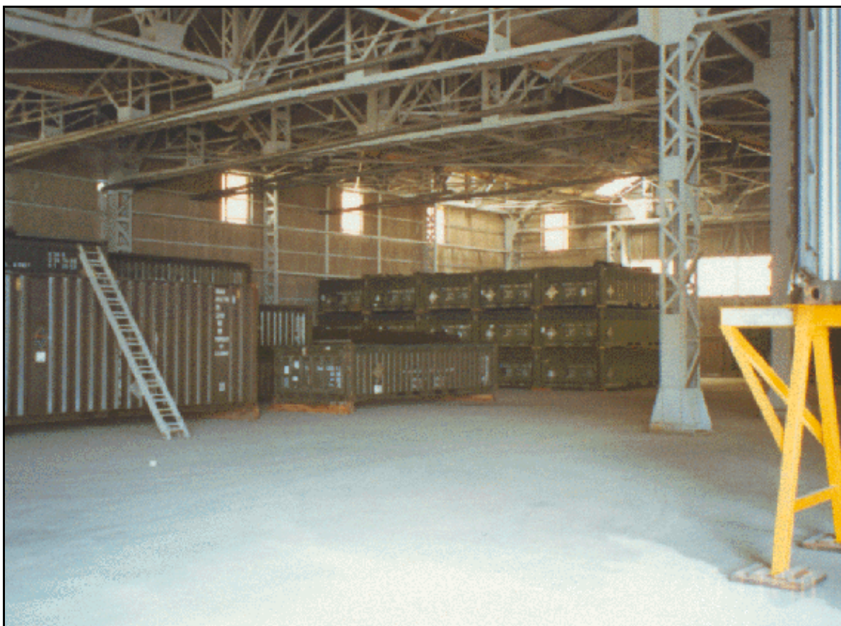
Hiro Container Repair Facility
