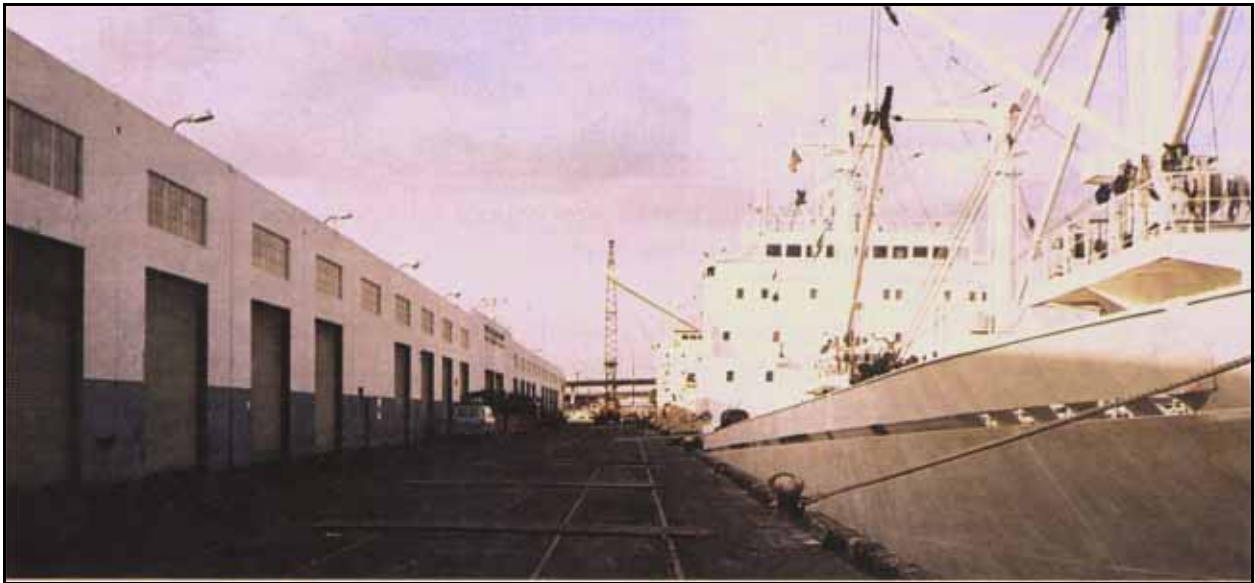
Covered Storage at Piers D and E; California United Terminal, Berths 12-13 (Northward View)
