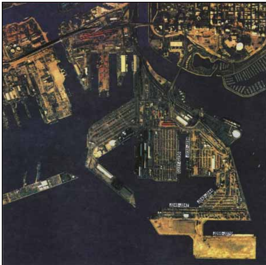
Piers G and J; New Pier J Under Construction
