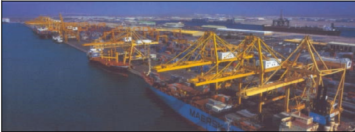
Container Cranes at Berth 14-17 (eastward view)
