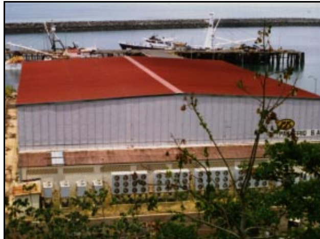
Covered Staging Area
