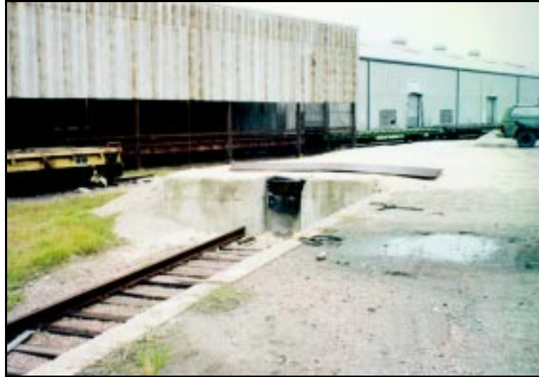
Fixed End Ramp at the Port of Beaumont
