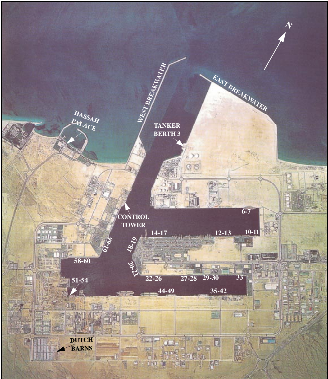
Aerial View of the Port of Jebel Ali (Photo circa 1996)
