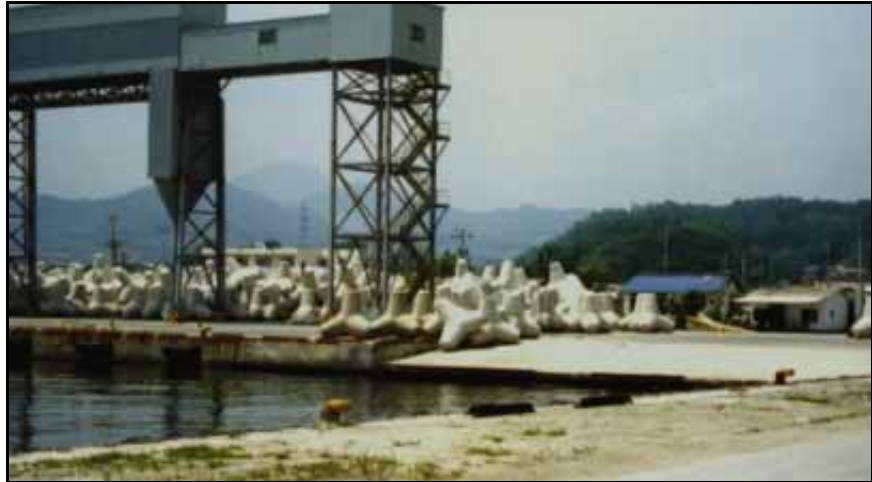
LST-Capable Ramps at Port of Samchok
