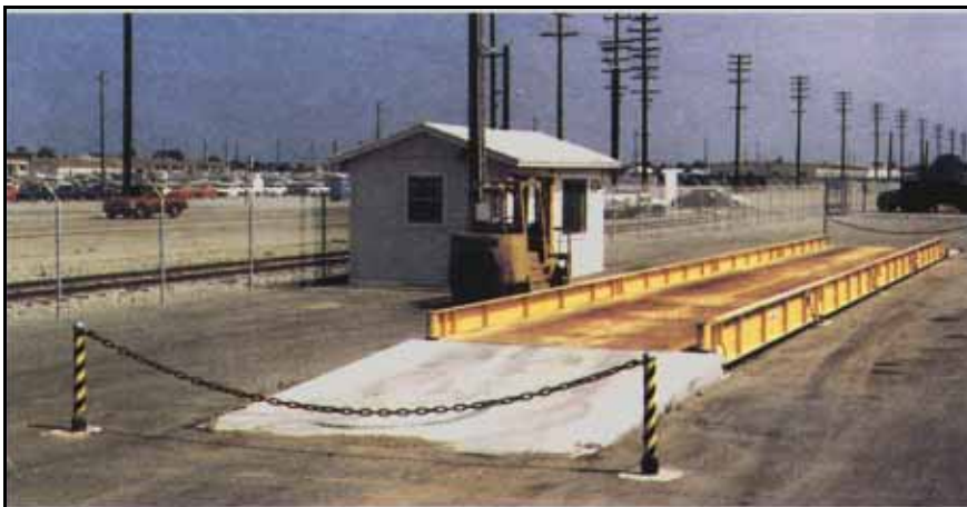
Truck Scales, Building 801 Compound
