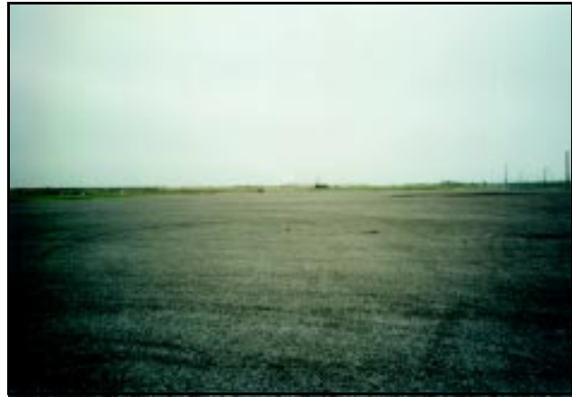
Paved Open Storage, Northside Terminal
