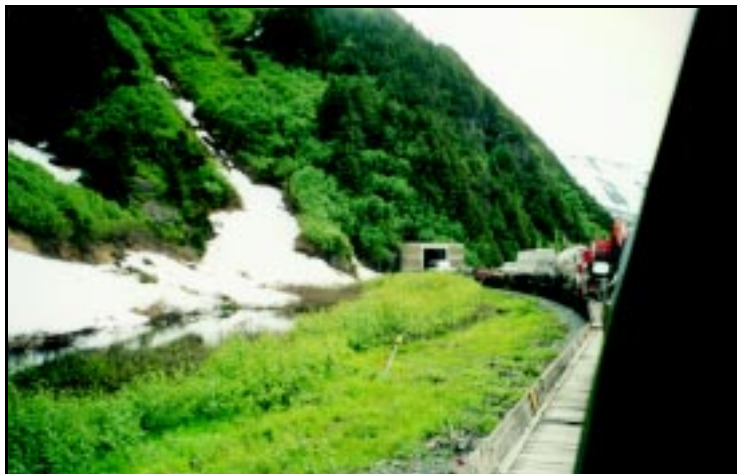
Rail Tunnel Near Portage
