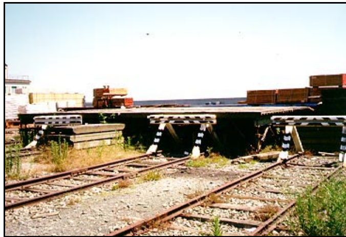
Rail End Ramp, Genova Terminal
