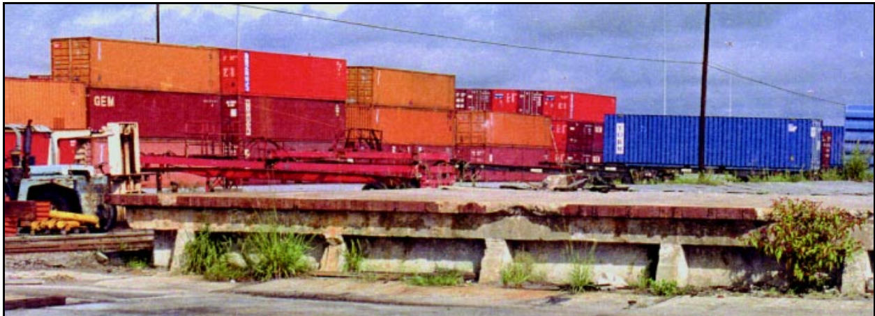
Fixed-Truck Ramp at Garden City Terminal
