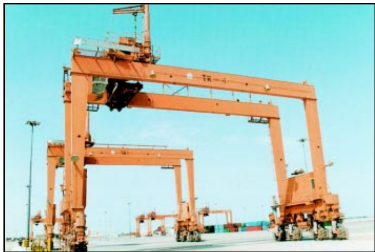
Container Gantry Cranes at the Port of Jubail
