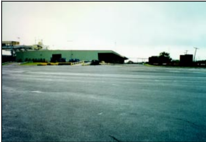
Open Staging Area
