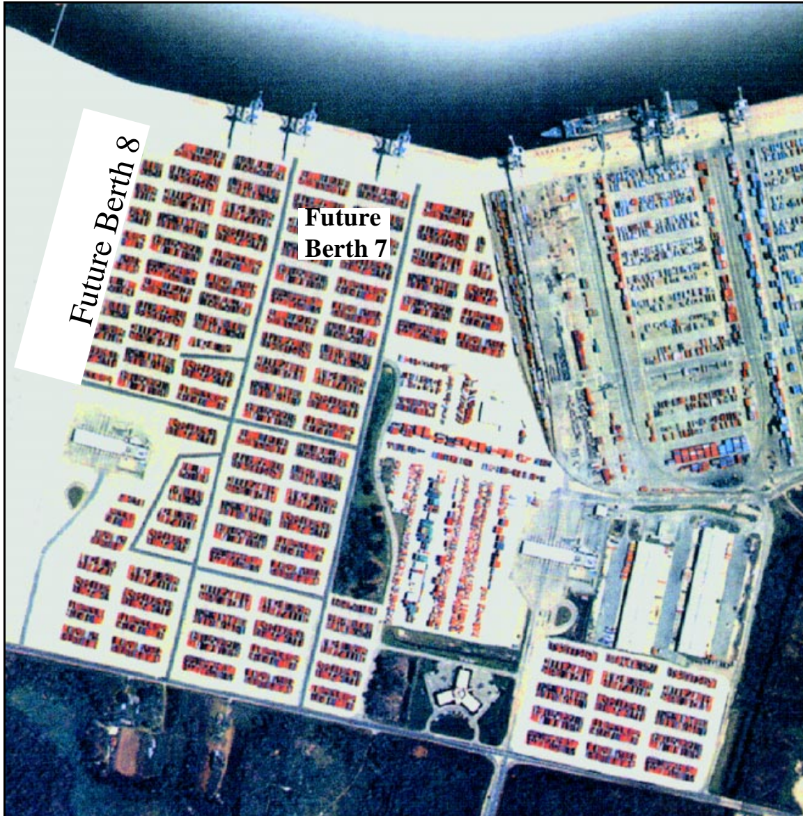
Future Berth 7 at Garden City Terminal
