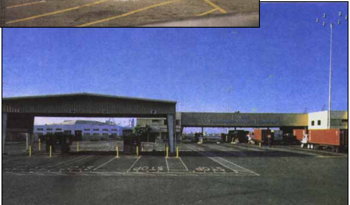
Gate to California United Terminal (Piers D and E)
