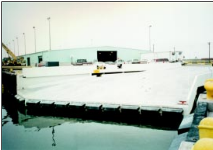
RORO Ramp at Cargo Dock (CD) 9
