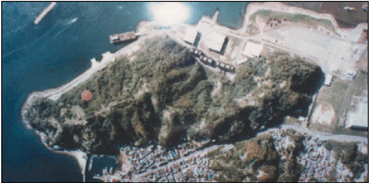
HIRO AMMUNITION STORAGE AREA
