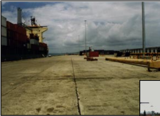
Pier 7 - Open Staging
