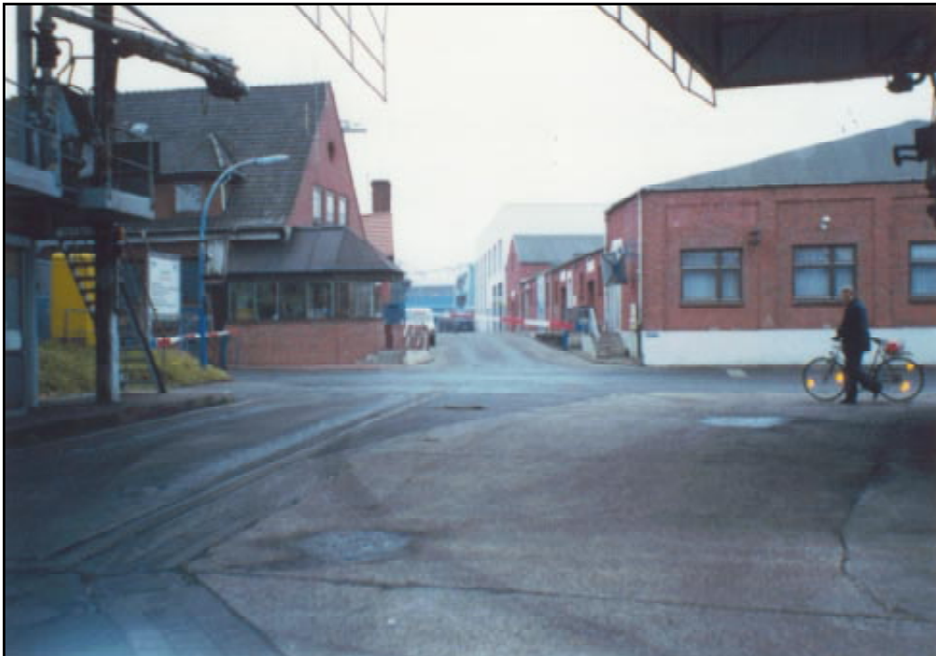
Main Gate to the Port of Nordenham
