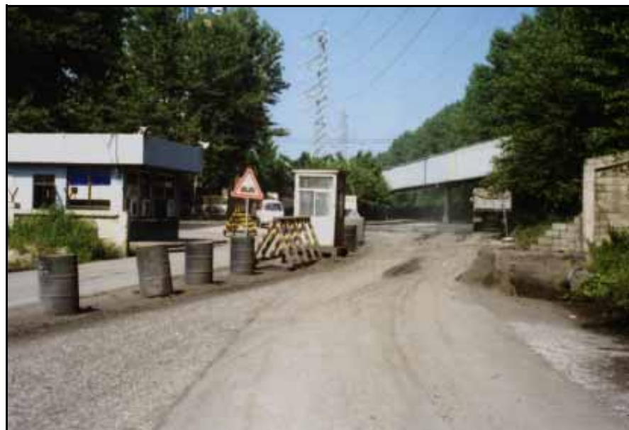
Gate to South Pier
