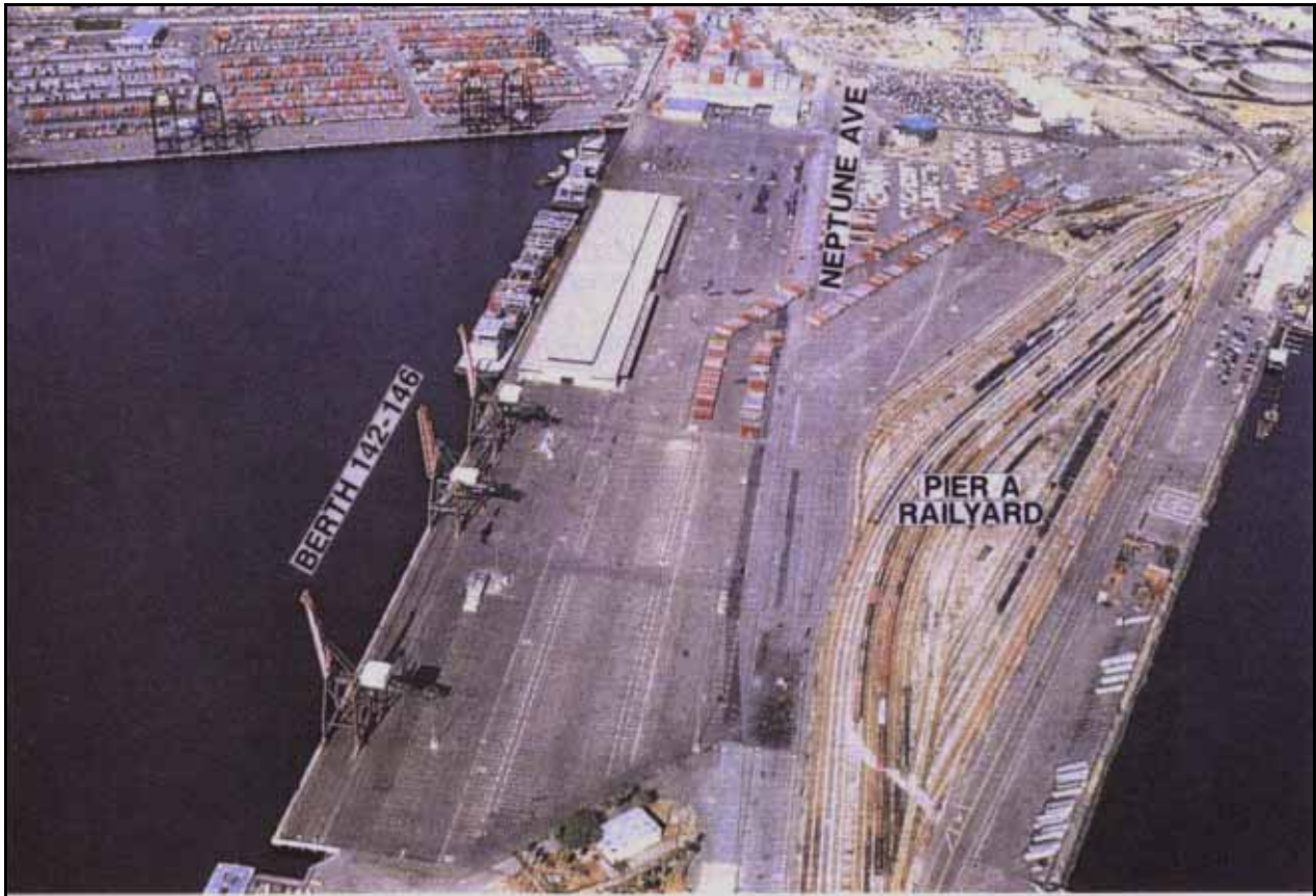
Berth 142-146 Terminal (Northward View)
