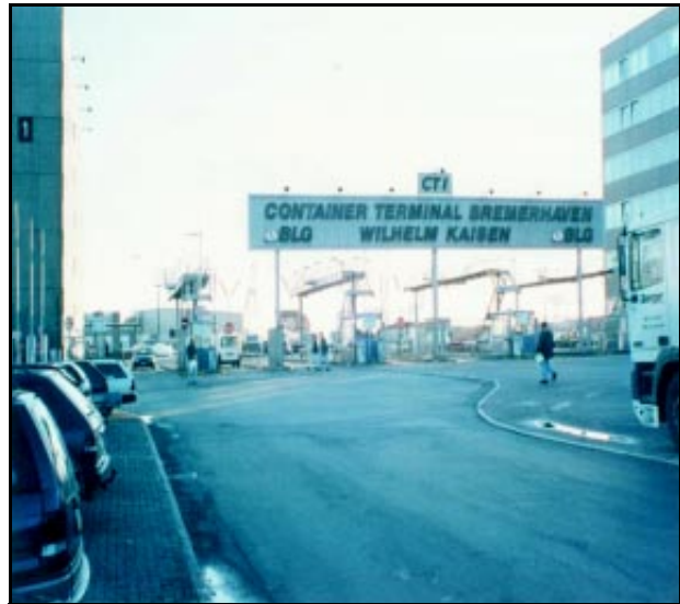
Container Gate to the Port of Bremerhaven
