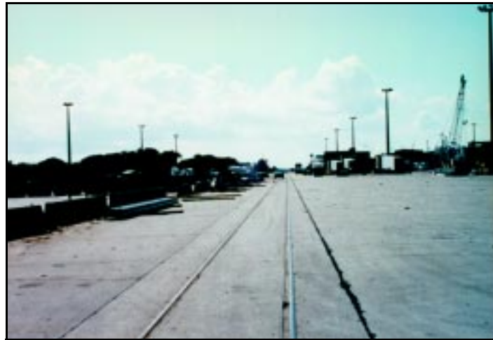
Spur Serving Fixed End Ramp at Barbours Cut
