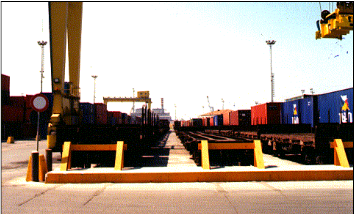
Rail Loading and Unloading Spurs at Tuscany Docks Terminal
