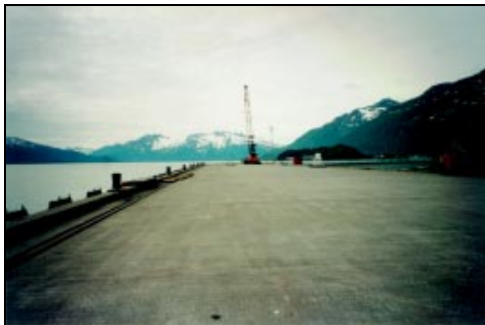
Ground-Level View of Container Terminal Wharf
