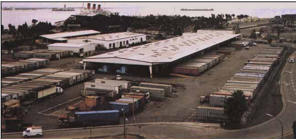
Covered Storage at Piers G and J Terminal; Sea-Land CFS near Berth G230 (Southeastward View)
