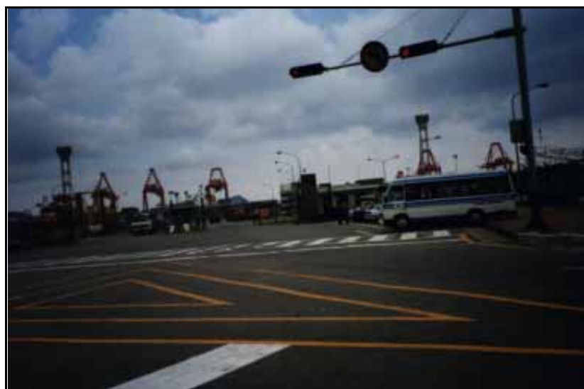
Access to Jasungdae Container Terminal
