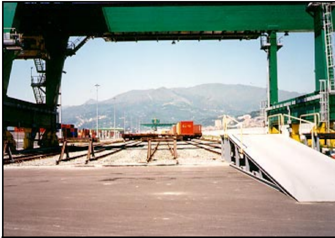
End Ramp and Rail Storage Yard, Voltri Terminal
