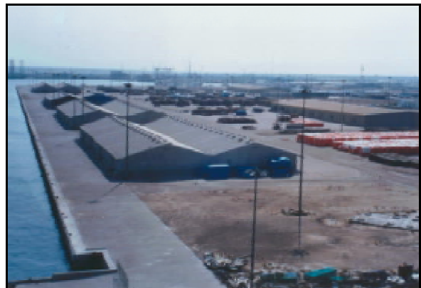
Transit Sheds at Berths 61-66 (southward view)
