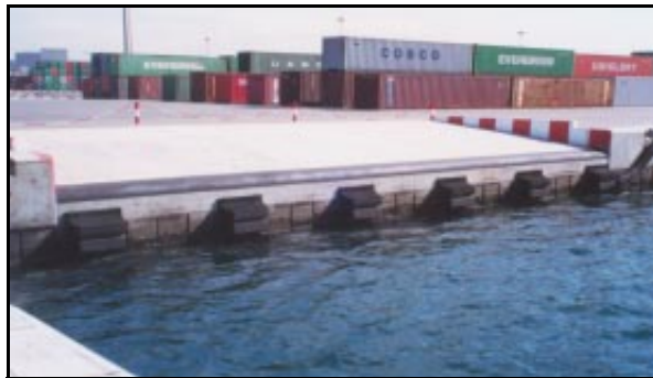
RORO Ramp at Berth 17
