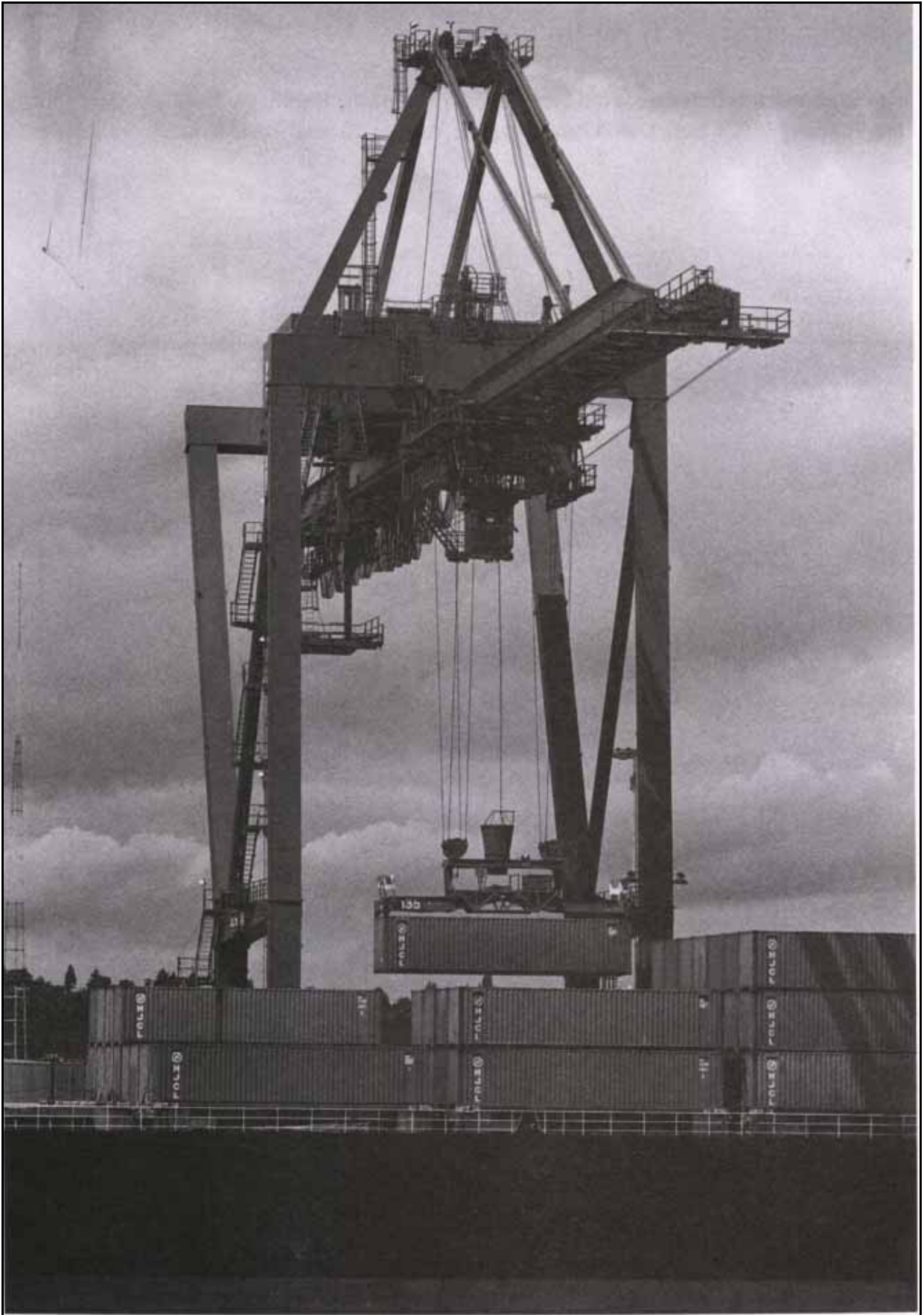
Container Crane at Terminal 18
