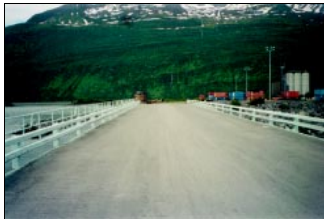
Access Way to Container Staging Area
