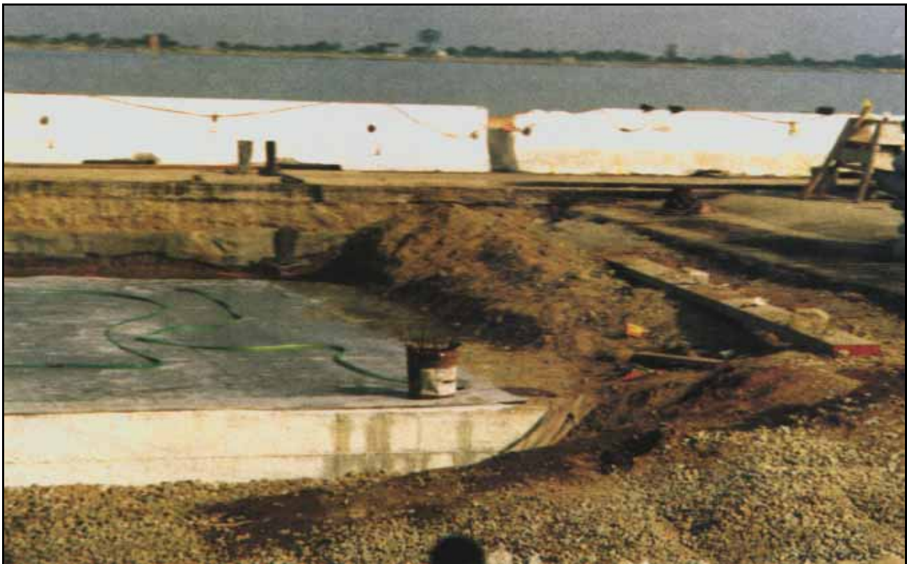
Shock Dissipation Improvements at Matson Terminal
