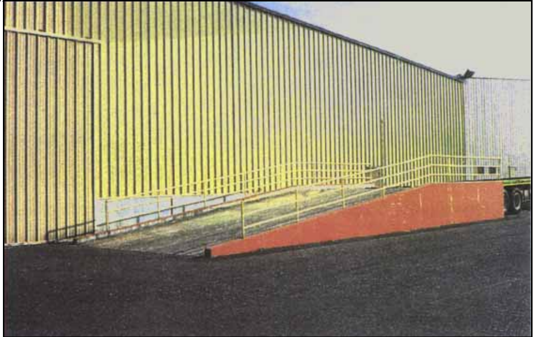
Truck Ramp at Terminal 2
