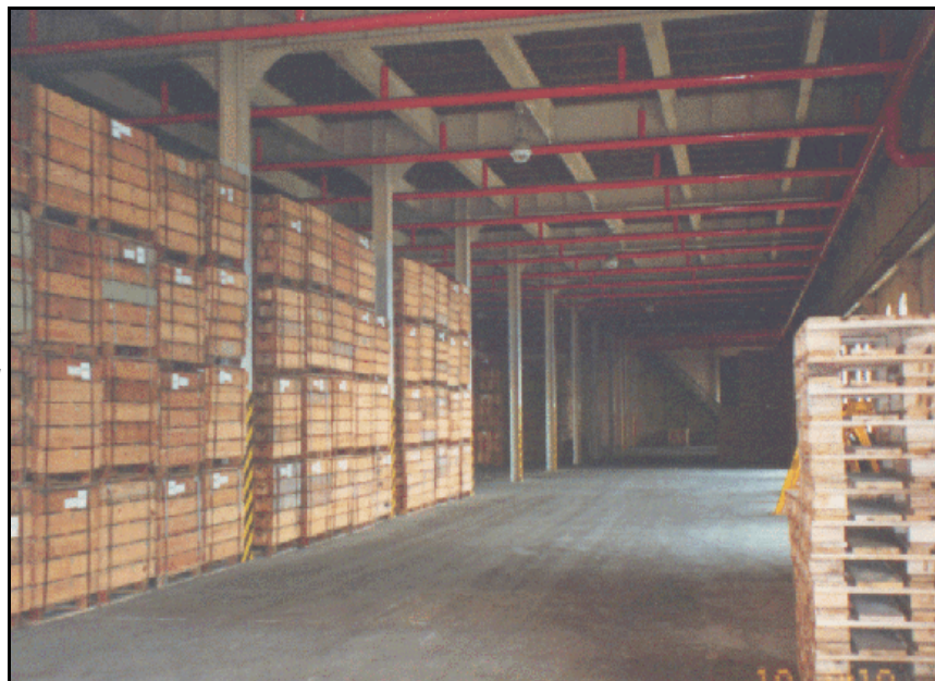
Covered Storage Building
