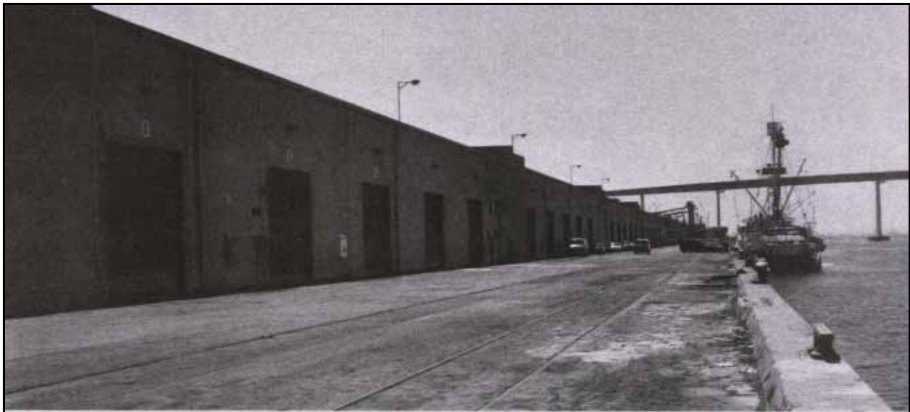
Covered Storage at 10th Avenue Terminal Berth 3-6 (Southeastward View)
