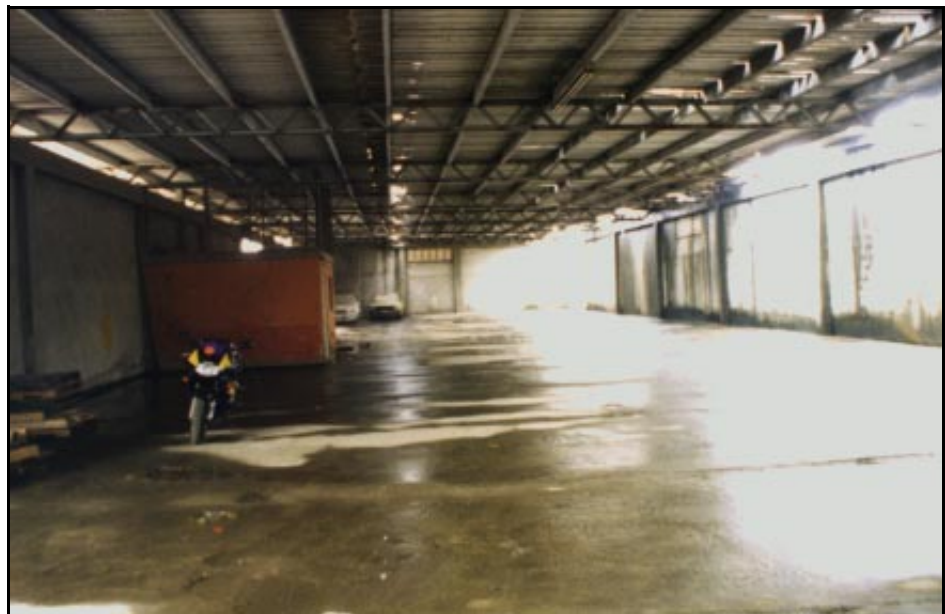
Container Freight Station
