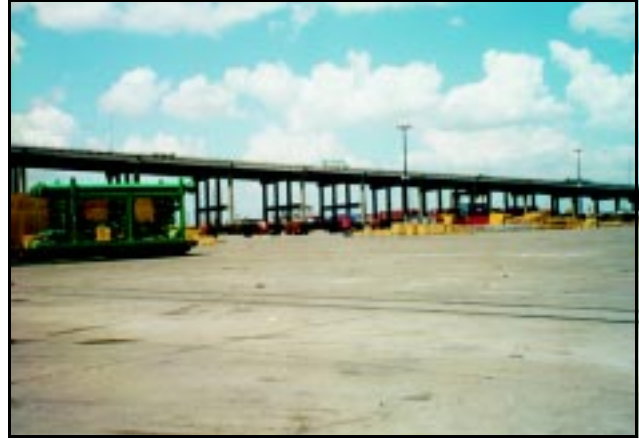
Portion of Open Staging at Berth 32
