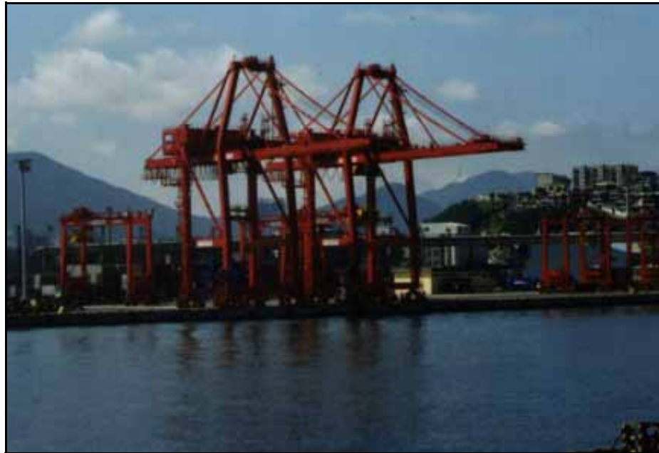
Southeastern portion of Pier 7
