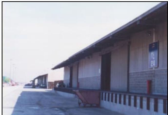
Truck Docks Near Berth 24 (northeastward view)
