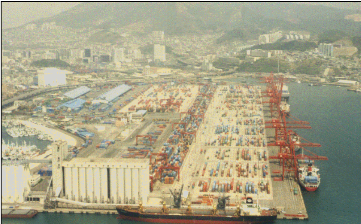
Jasungdae Intermodal Facilities
