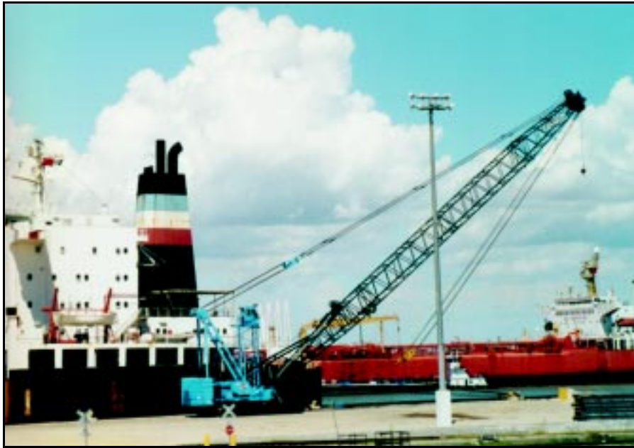
Manitowac 250 Crawler Crane at Cargo Dock 8
