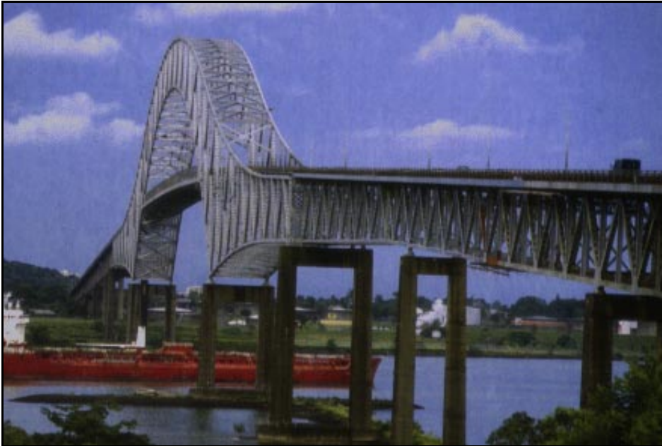
Bridge of the Americans along the Inter-American Highway
