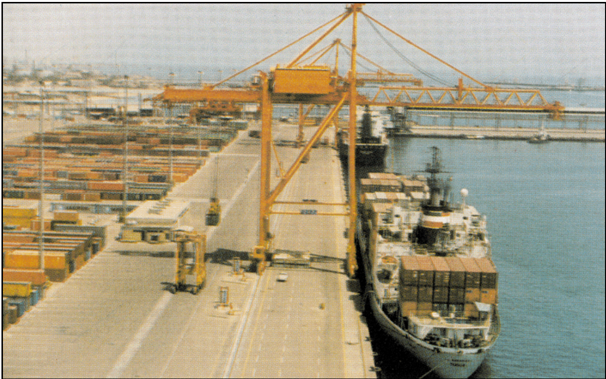
Container Staging at Berths 15 and 16 at Port of Shuaiba (northward view)
