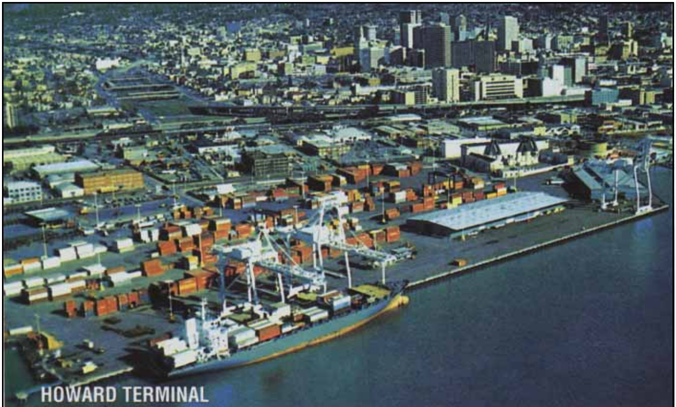
Figure 6. Howard port facilities.
