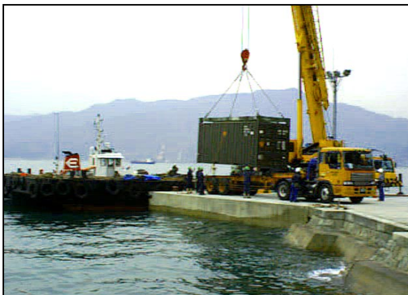
Terminal Handling at Akizuki Barge Pier
