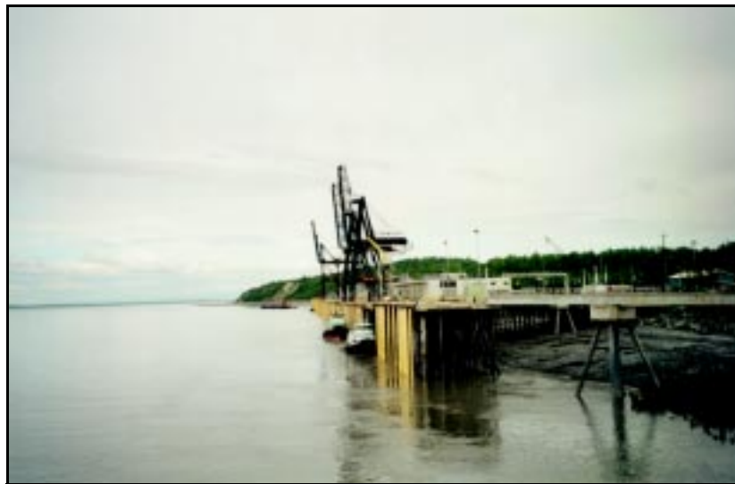
Port of Anchorage Wharf (Terminals 1-3) at Low Tide
