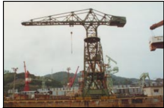
Ship Yard Crane
