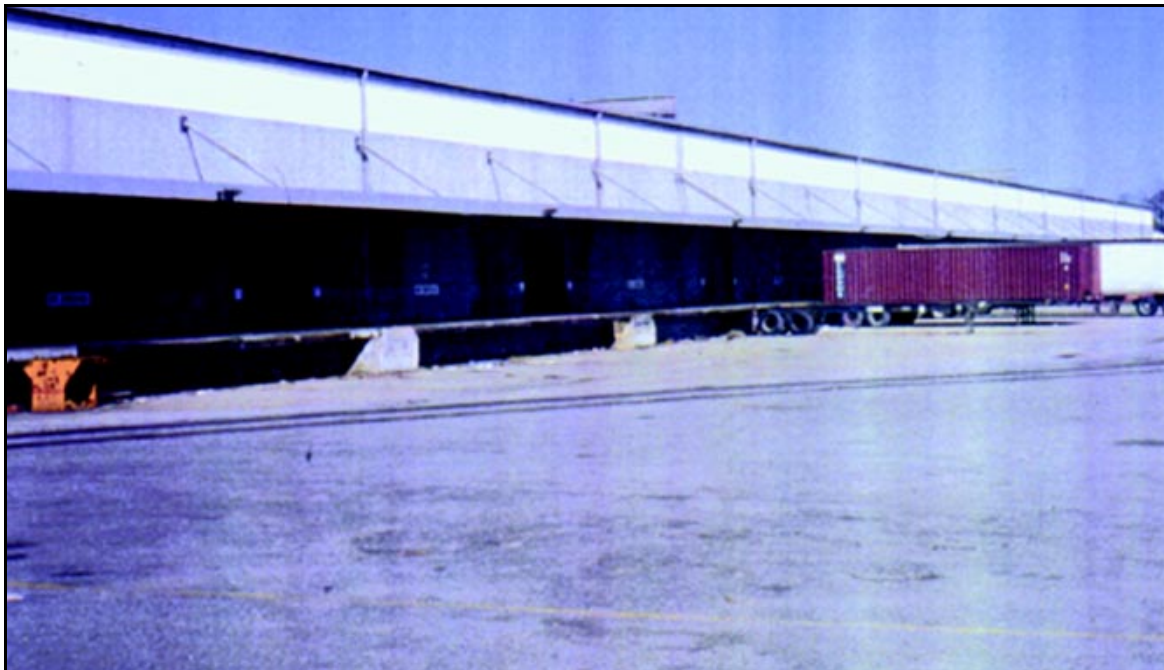
Covered Staging at Lamberts Point Docks (eastward view)
