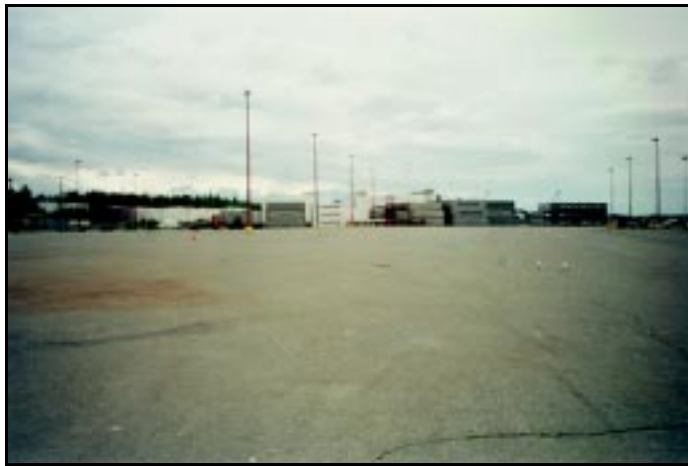
Open Staging Area (South Transit Area)
