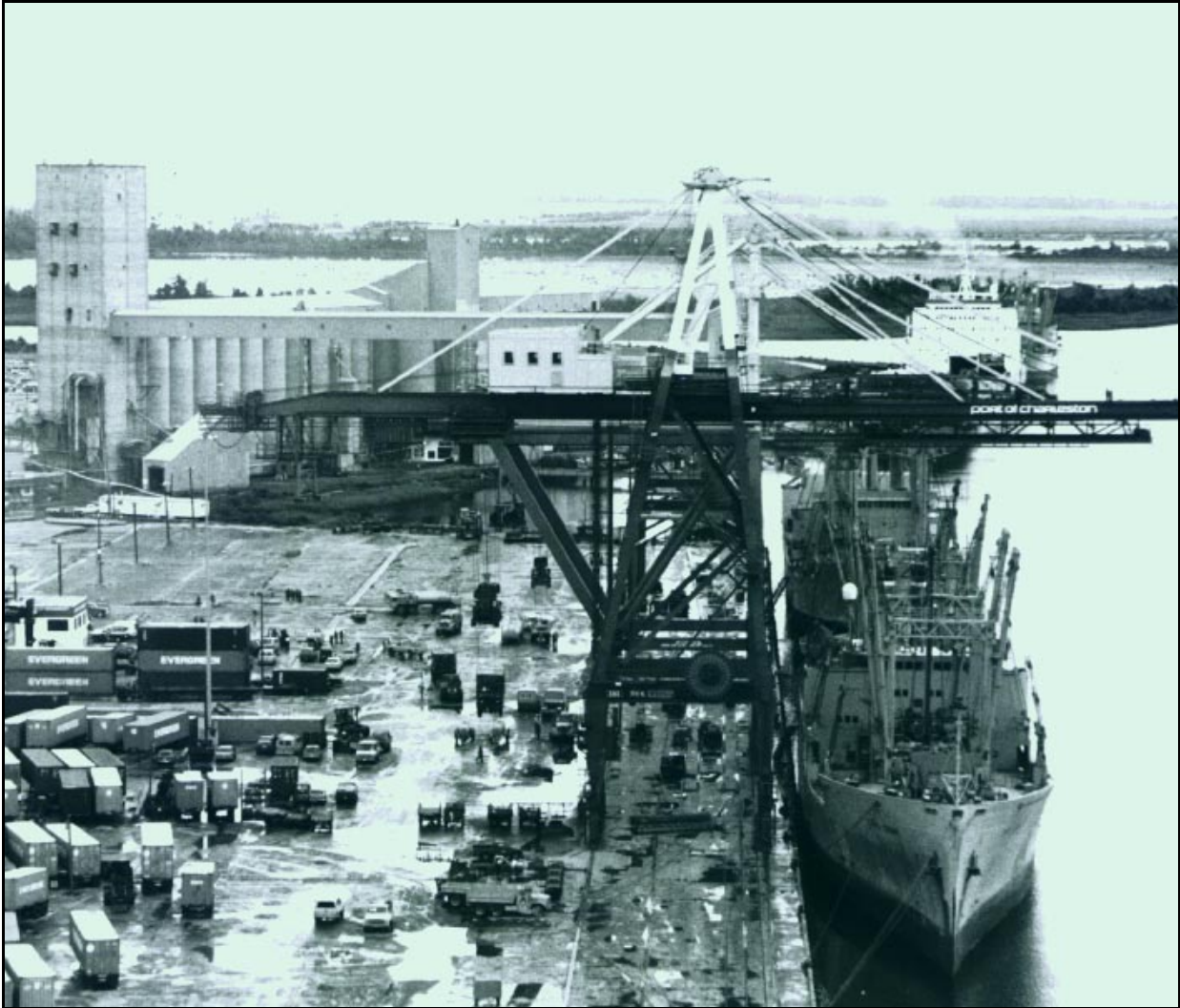
Open Staging at Berth 3 of the North Charleston Terminal (Northeastward view)
