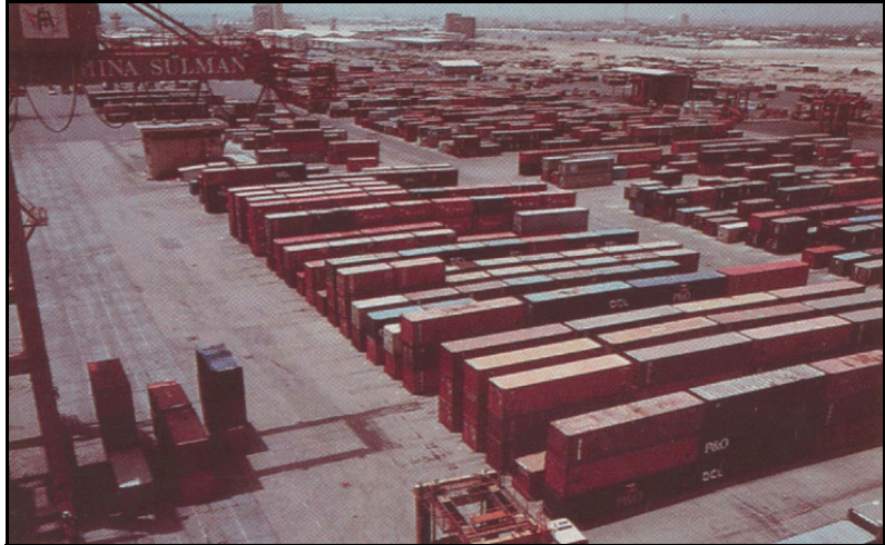
Westward View of Container Staging at the Container Terminal (Berth 15-16) of the Port of Mina Sulman
