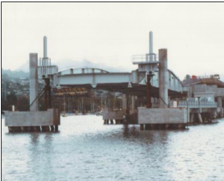
Ford Island Bridge under construction
