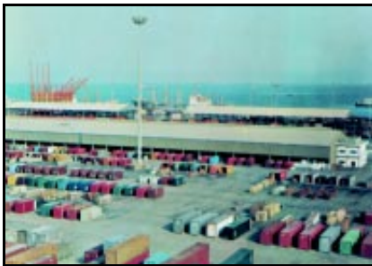
Container Staging at Container Terminal at Port of Ad Dammam (eastward view)
