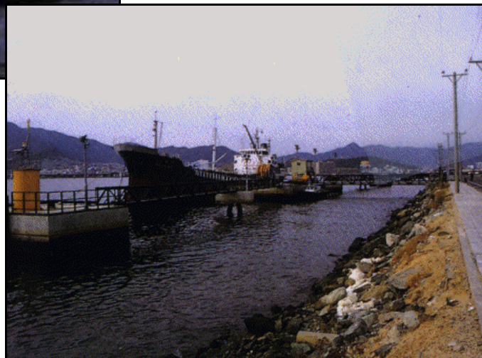
Dolphin Wharf Honam Oil Refinery
