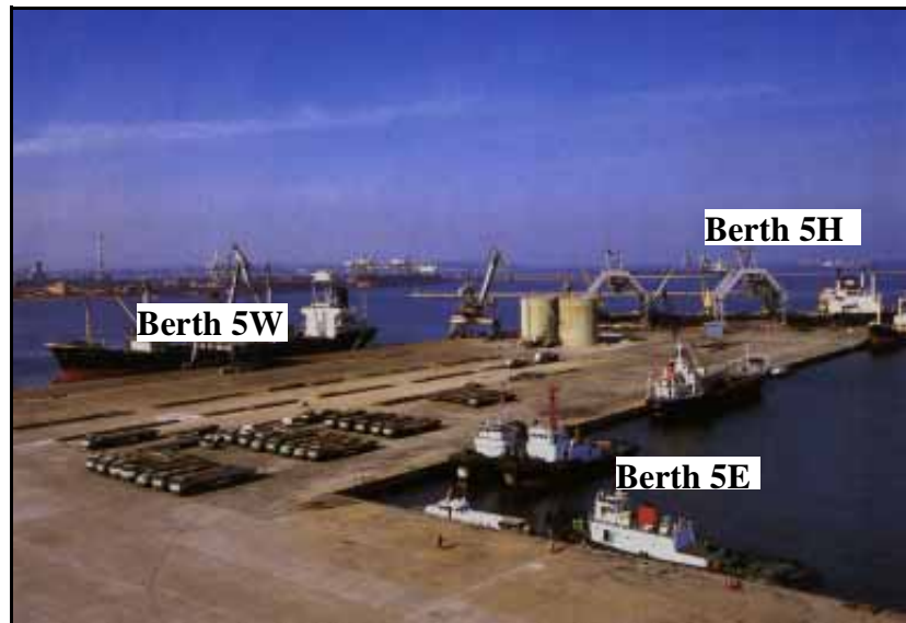
Pier 5 of Port of Pohang (Prior to shed construction)
