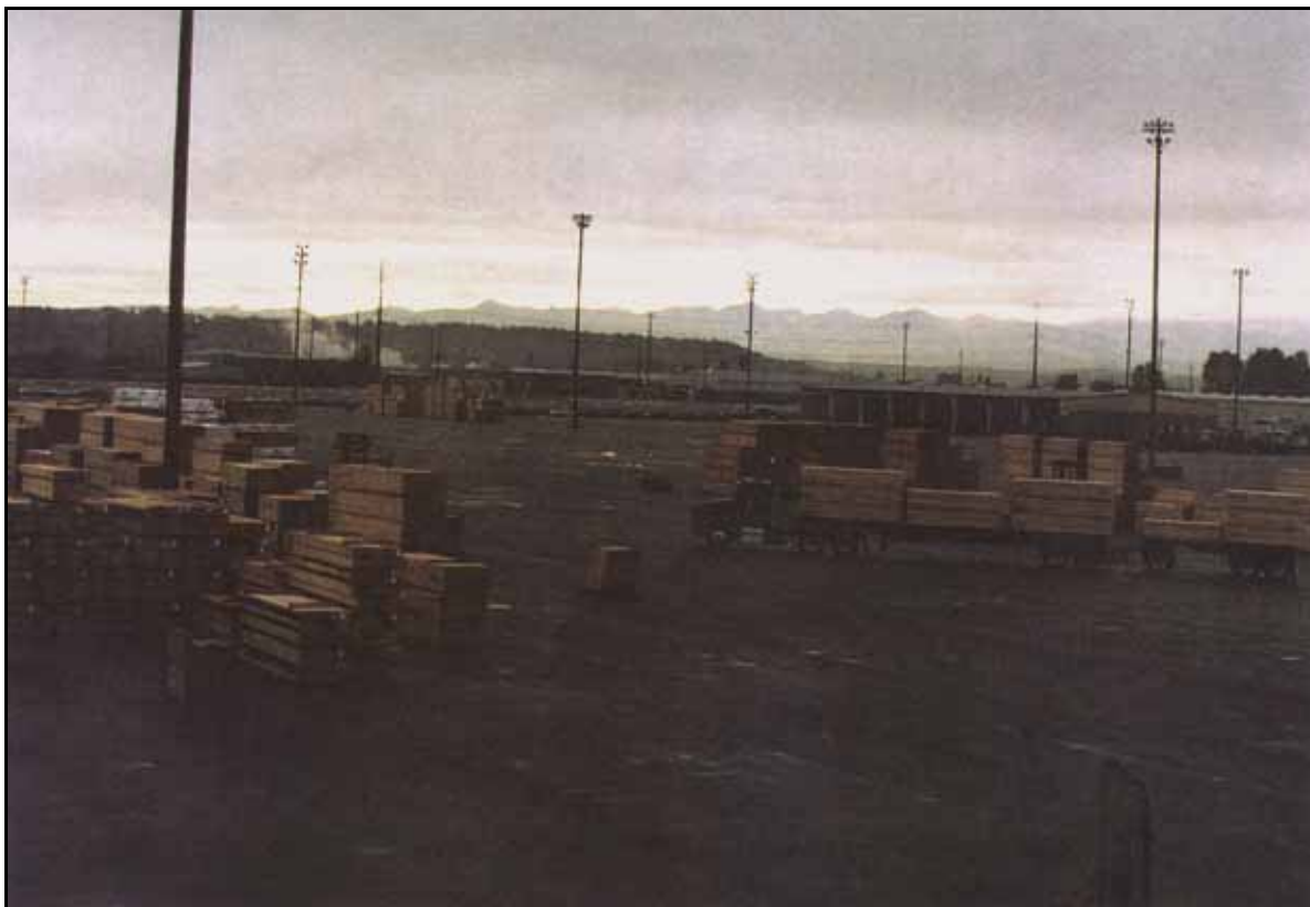
Open Staging Area at Pierce County Terminal (southeastward view)
