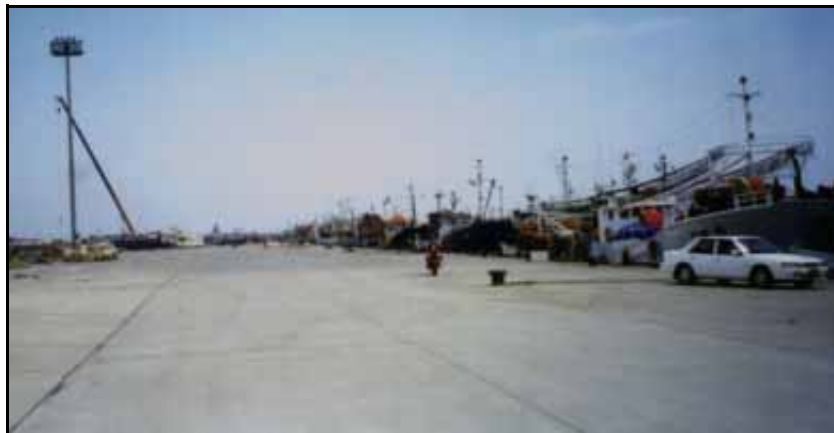
New Wharf (looking east)
