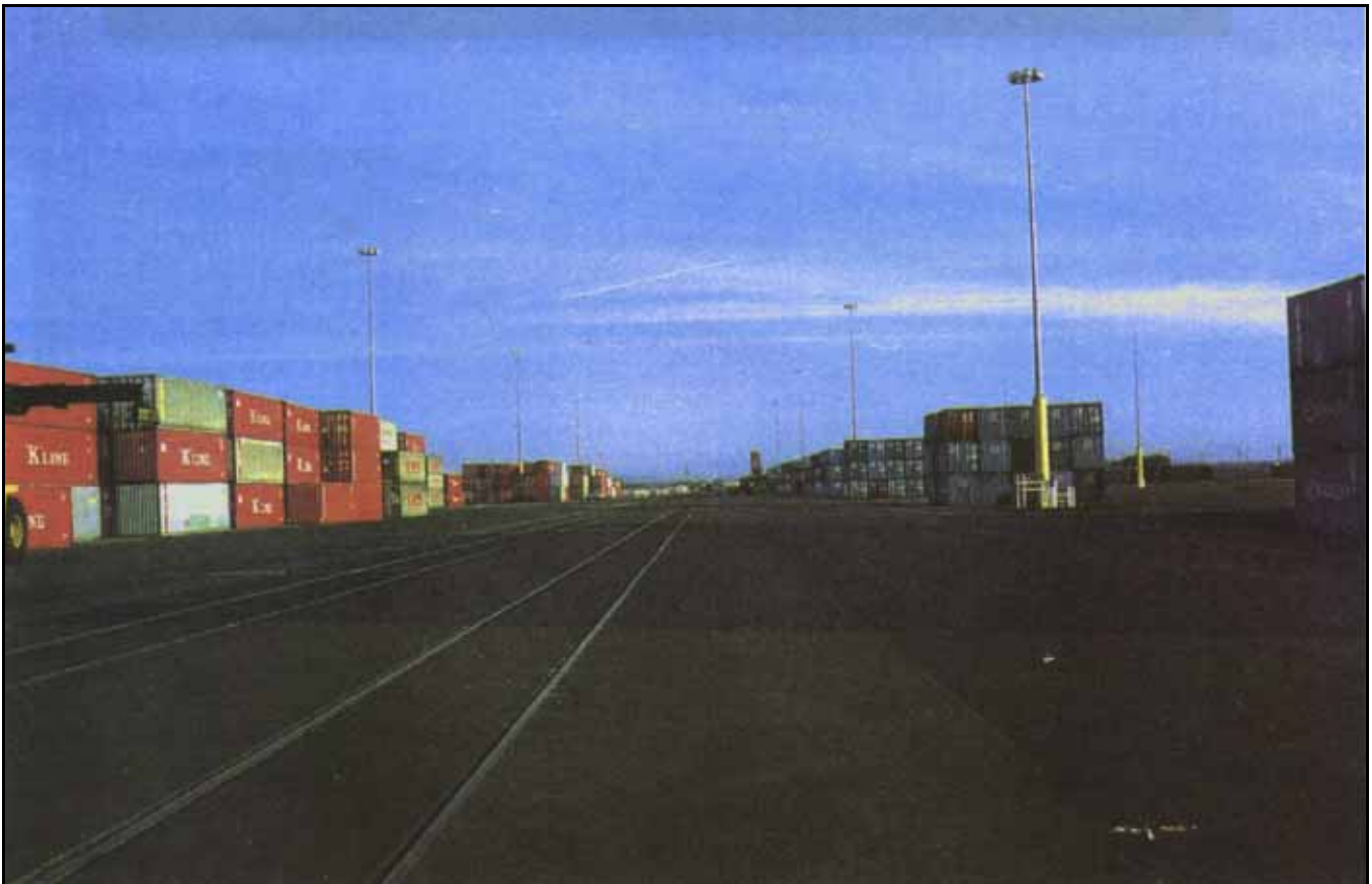
New Intermodal Railyard, Terminal 6
