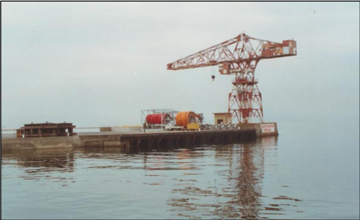
Barge Berth at Iwakuni
