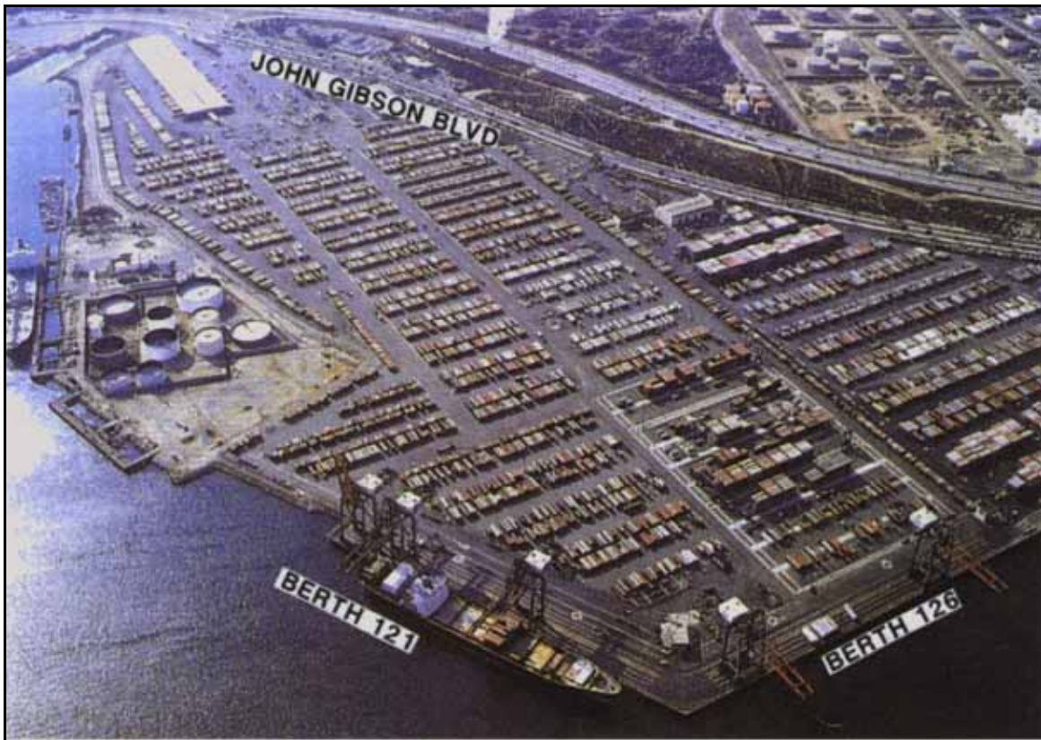
APL Terminal (Westward View)
