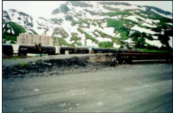
Fixed Rail End Ramp at the Port of Whittier
