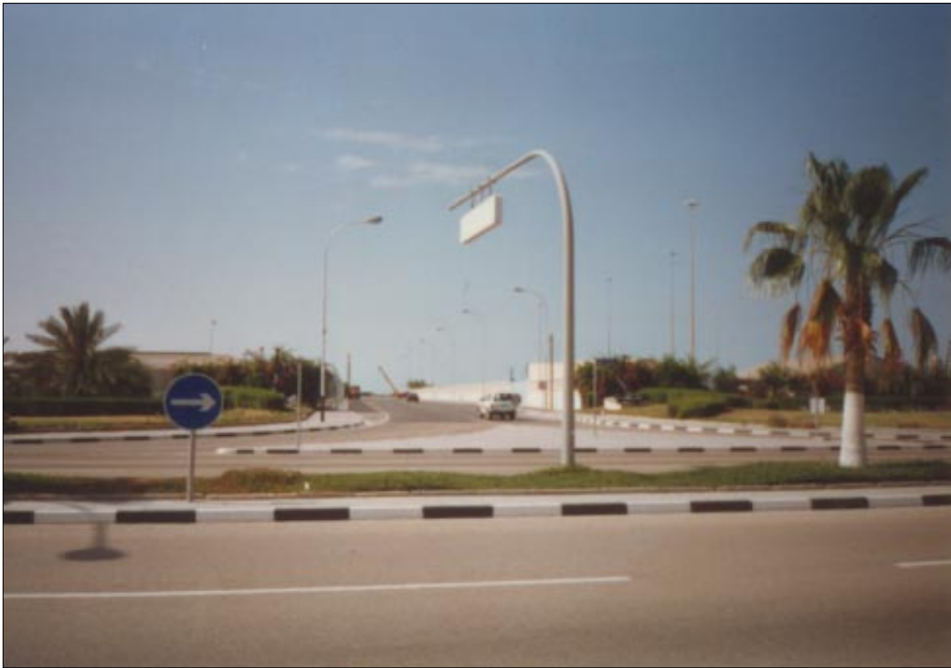
Driveway into the Port of Doha (northeast view)
