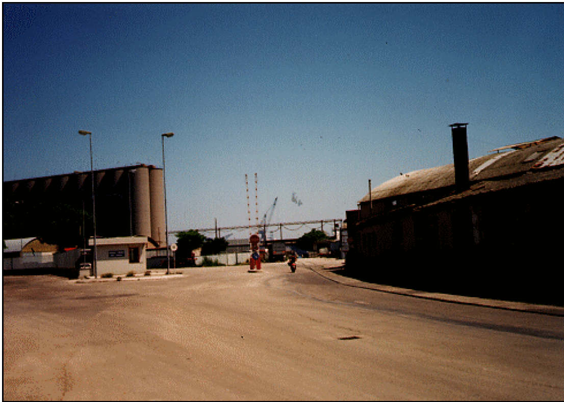
Via Marconi Gate
