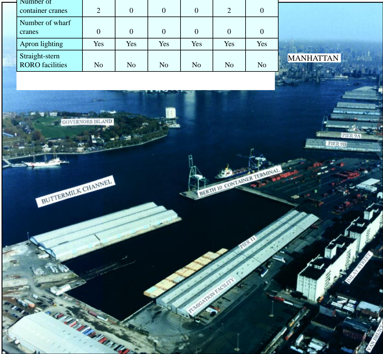
Red Hook Terminal (Northward view)
