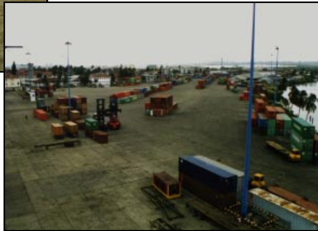
Open Staging - Pier 9 and 10
