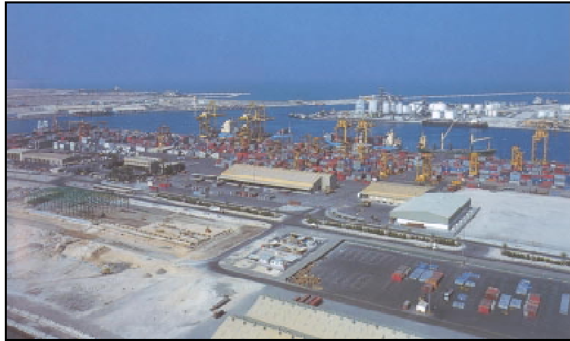
Container Storage Area at Berth 14-17 (northwestward view)
