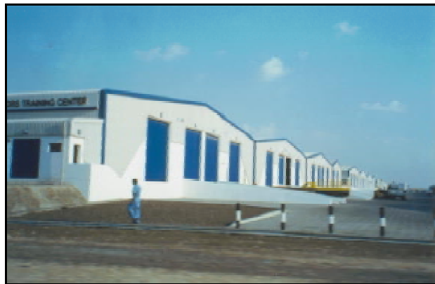
Dutch Barn Warehouses Inland of Berth 54 (westward view)
