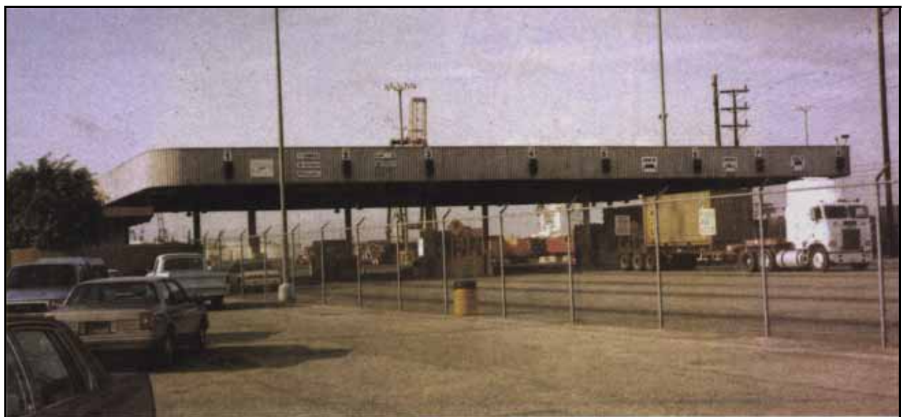
Gate to Los Angeles Indies Terminal
