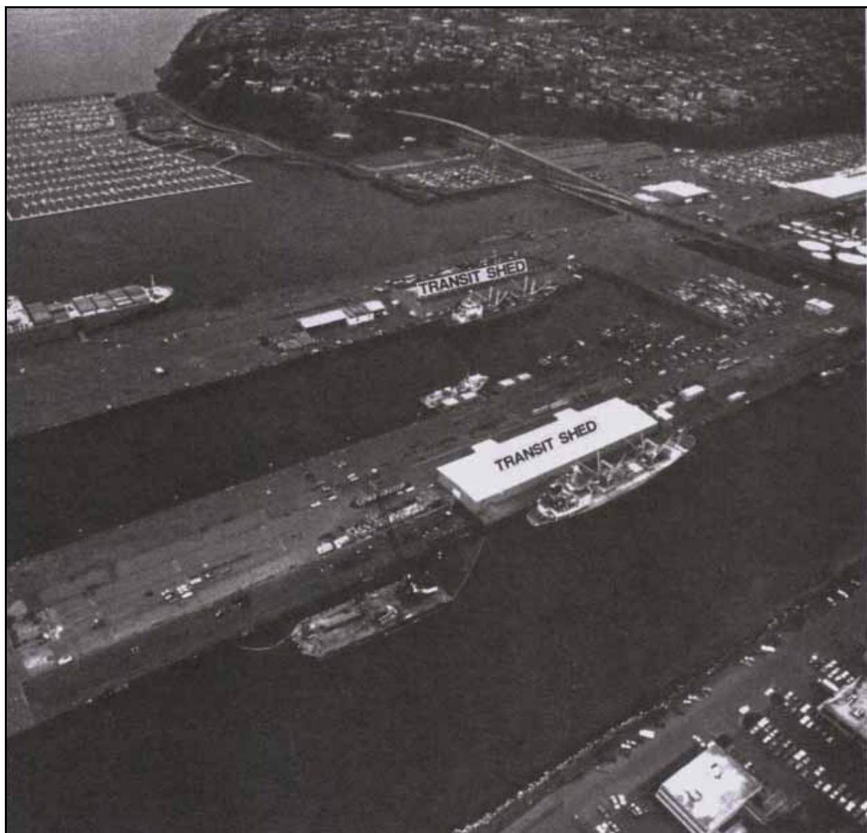
Covered Storage Facilities, Terminal 91
