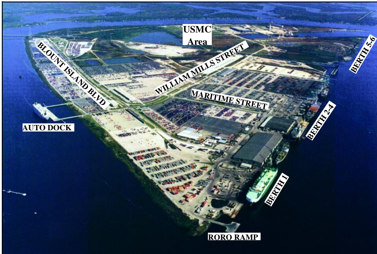
Blount Island Terminal (Northeastward view)
