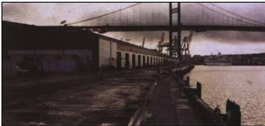
Covered Storage and Apron Track at Indies Terminal Berth 222 (Southward View)
