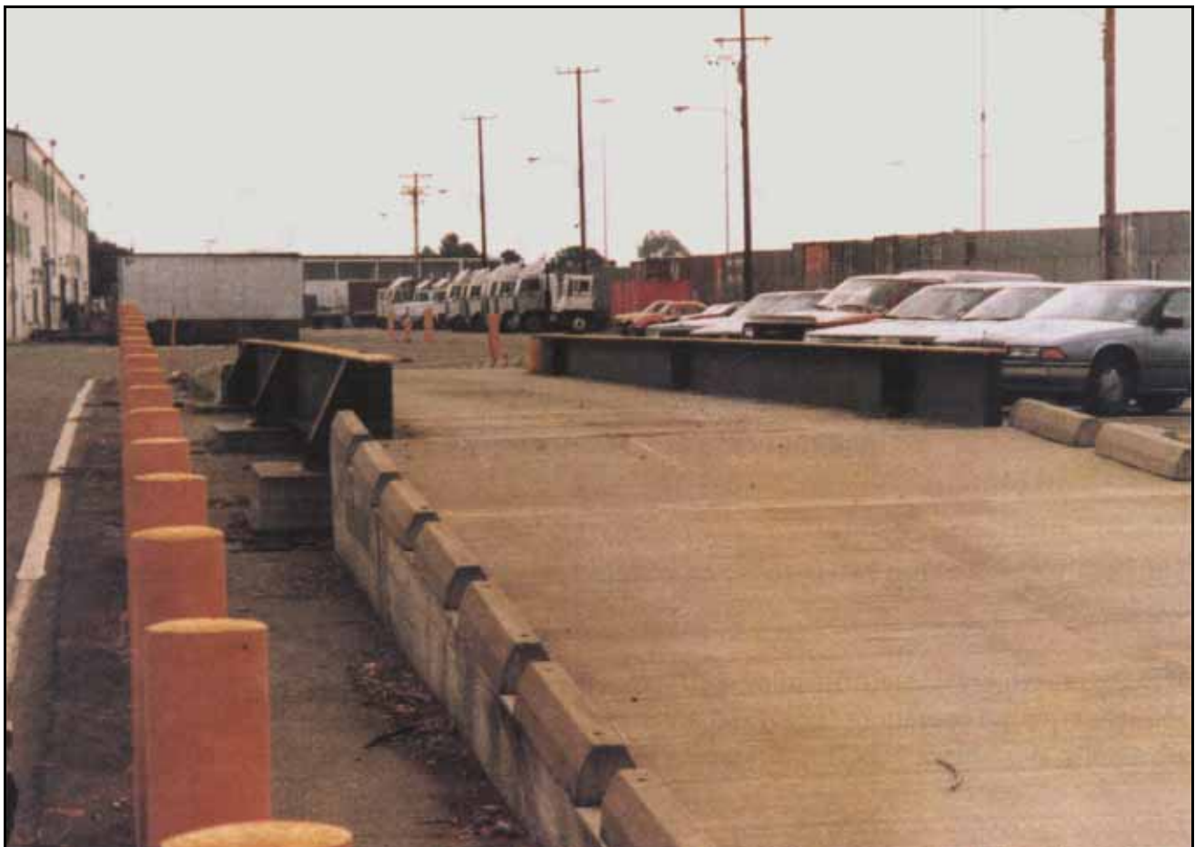
Truck Scales at the 1302d Major Port Command
