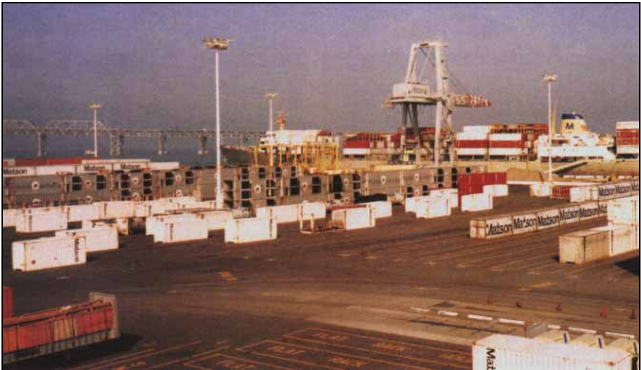
Matson Terminal Open Staging Area
