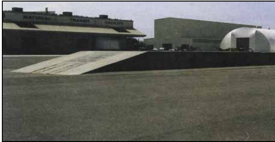
Fixed Concrete Ramp Near Building 801
