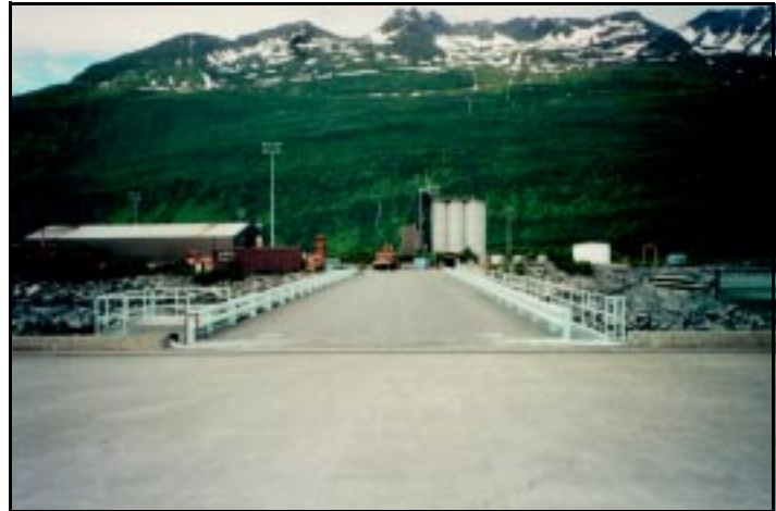
One of the Two Road Access to the Floating Dock
