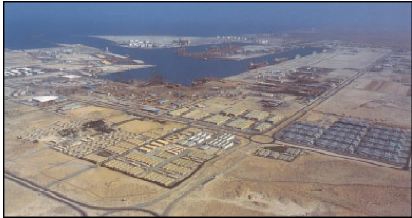
Offsite Marshaling (northward view)
