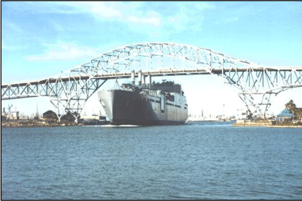
Corpus Christi Ship Channel and Harbor Entrance Bridge (U.S. 181) (LMSR USNS Sisler Accessing Harbor)
