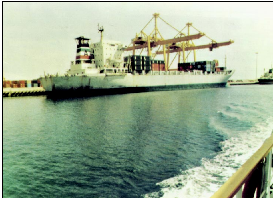
Container Terminal (southward view)
