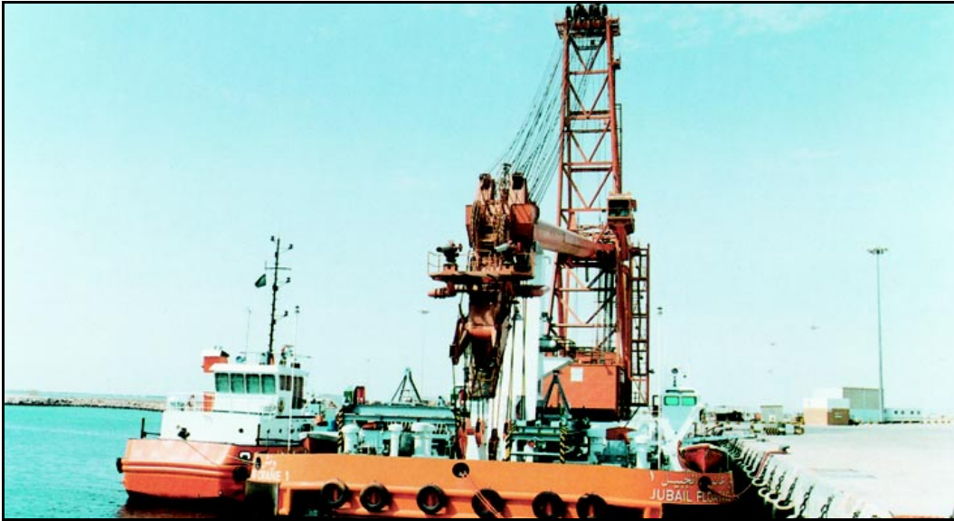
Floating Crane at the Port of Jubail
