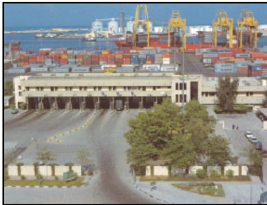
Gate to the Container Terminal, Berth 14-17 (northwest view)
