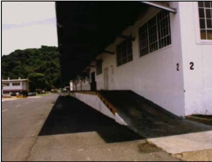
Building 2 - Main Warehouse (south dock)
