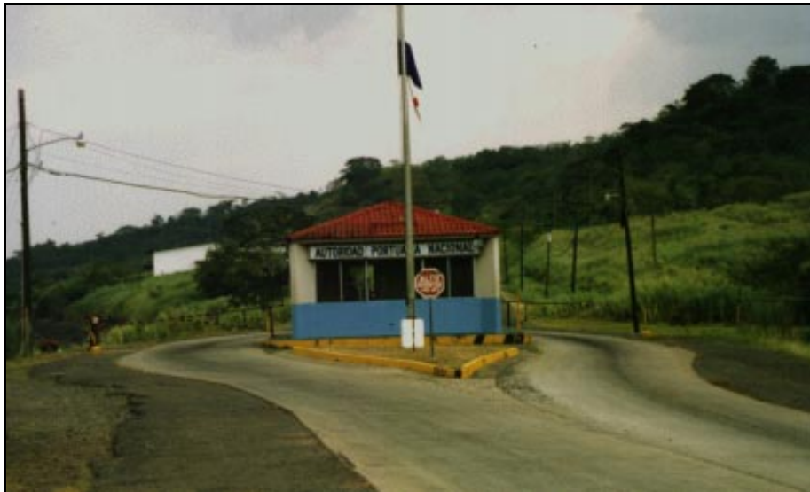
Gate at Port of Vacamonte
