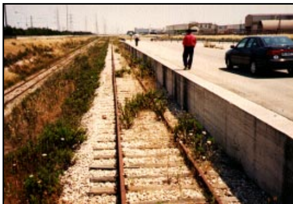
Side Ramp at Costa Morena Terminal
