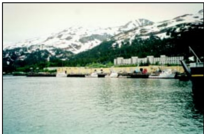
Alaska Railroad Marginal Wharf with Transit Shed
