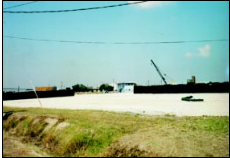
Open Staging Area
