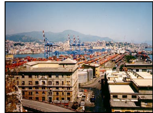
Sanita Container Terminal (on left) and Bettolo (on right)
