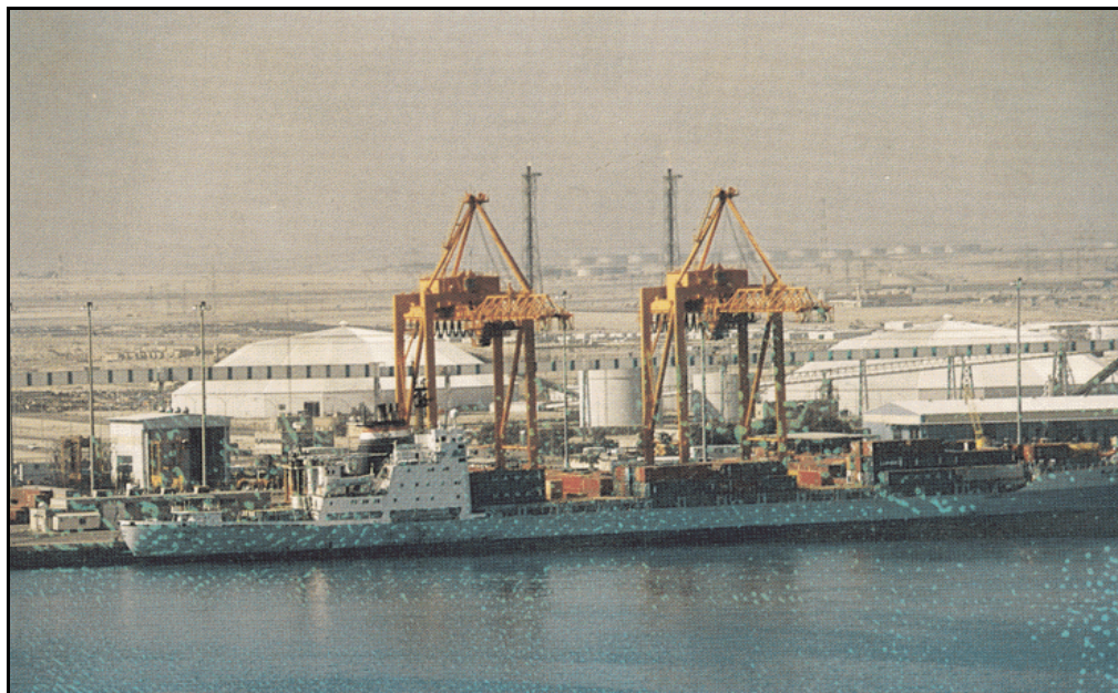
Berth 15 and 16 Container Cranes at Port of Shuaiba (westward view)
