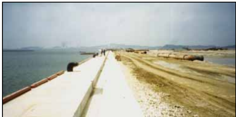
Construction of Southward Container Terminal
