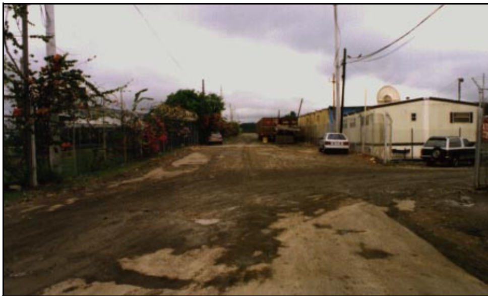
Access road to general cargo berth
