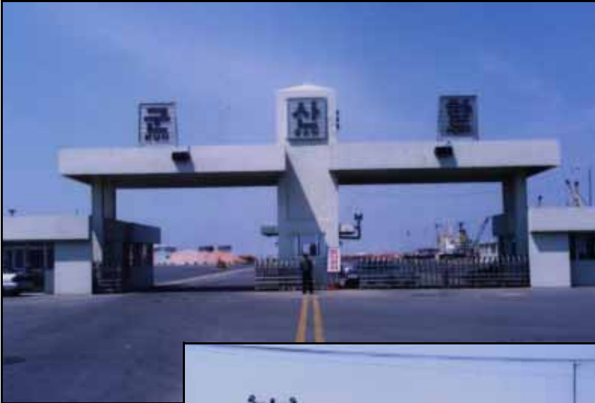
West Gate to Port of Kunsan
