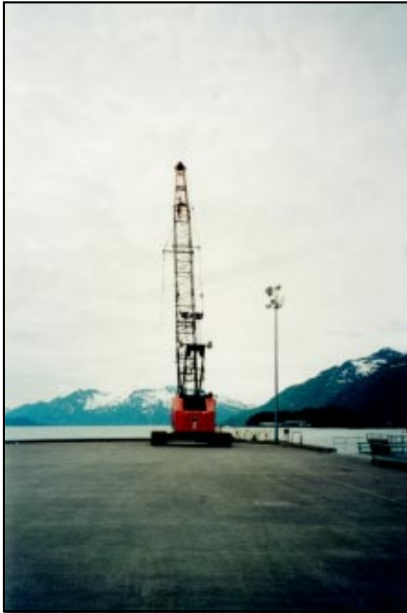
Manitowoc Tracked Mobile Crane
