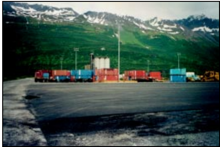
Paved Open Storage Area at the Container Terminal
