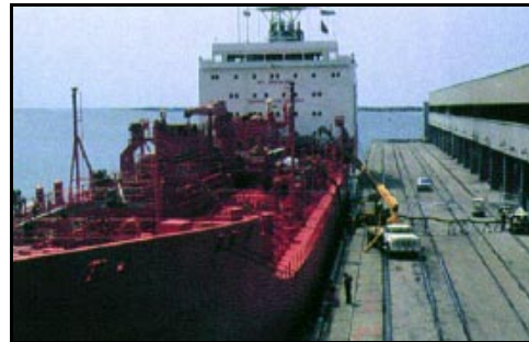
Apron Tracks at Berths 6 and 7
