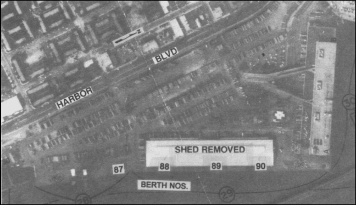
San Pedro Main Channel Terminal (Westward View)
