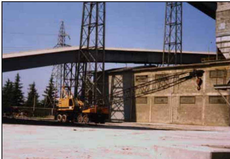
Mobile Crane Used at Port of Tonghae
