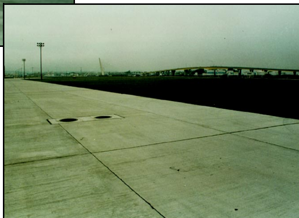
Open Staging at Kawaragi Pier 1
