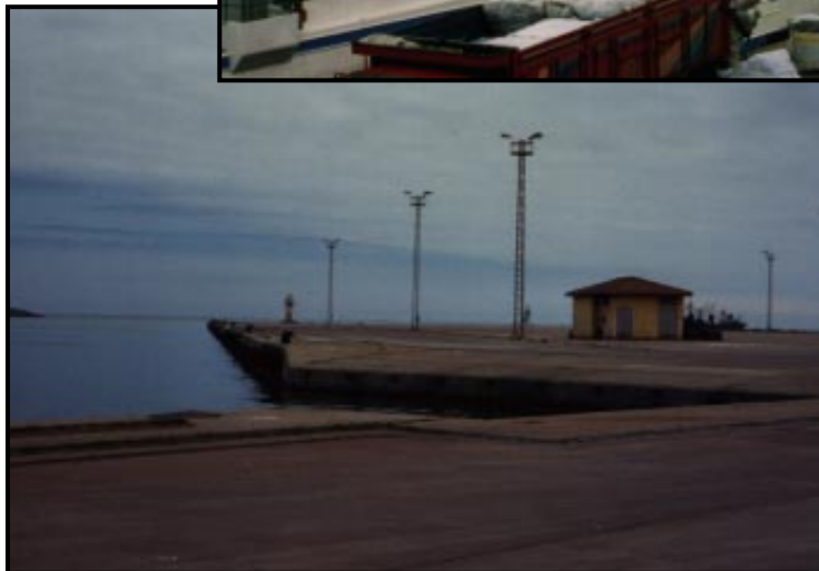
RORO Ramps seen from Berth 3
