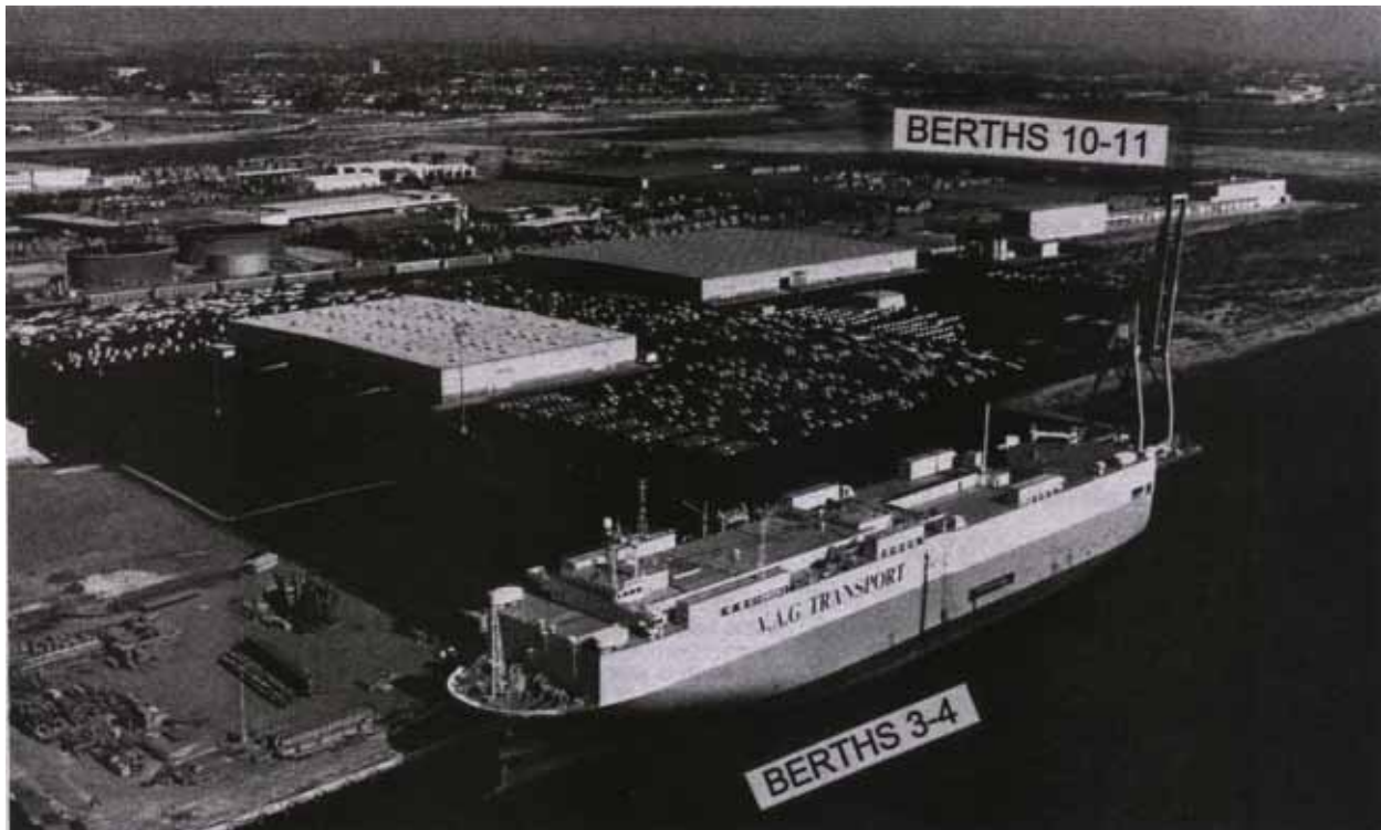
Figure 2. Aerial view of National City Terminal
