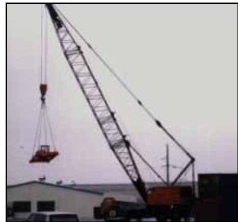
Mobile Crane Rigged for 20-foot Containers
