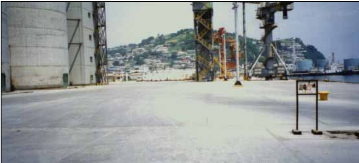
Open Area at South End of Pier 2 (northward view)
