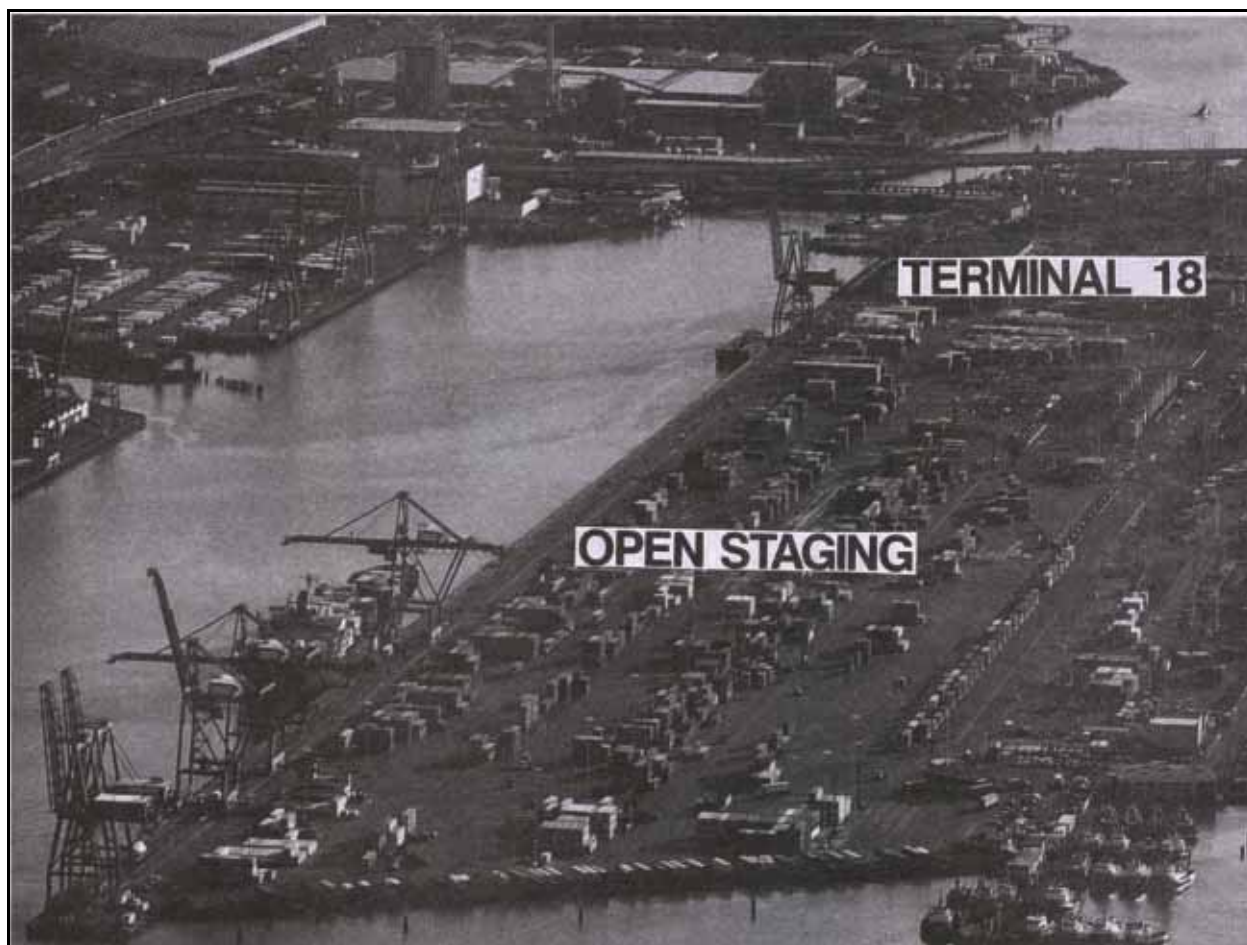
Terminal 18 Staging Area
