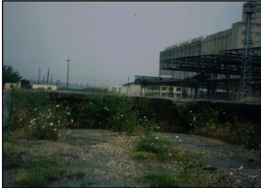
North-end Truck Ramp
