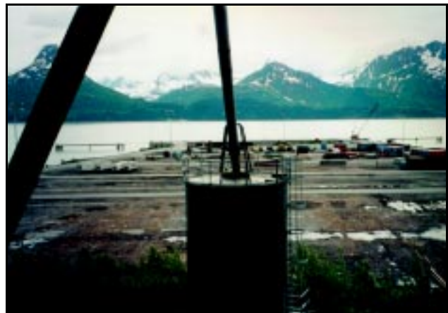
Open Storage Area at the Port of Valdez ( to be paved)
