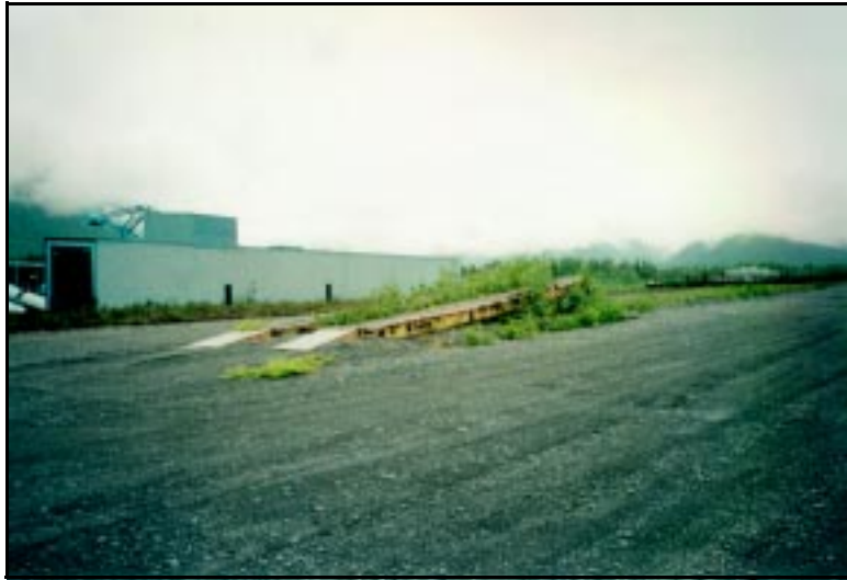
Fixed Rail End Ramp at Seward Railyard
