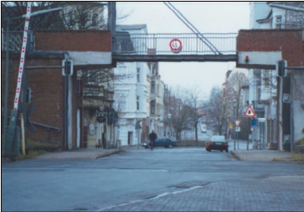
Highway and Rail Underpass
