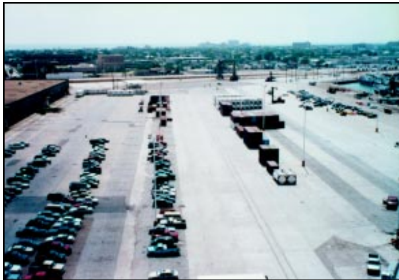
Open Staging Area at Pier 10
