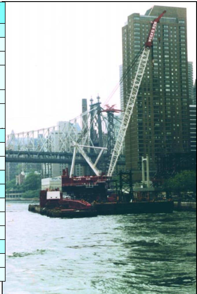
Weeks Marine Inc. Barge Crane
