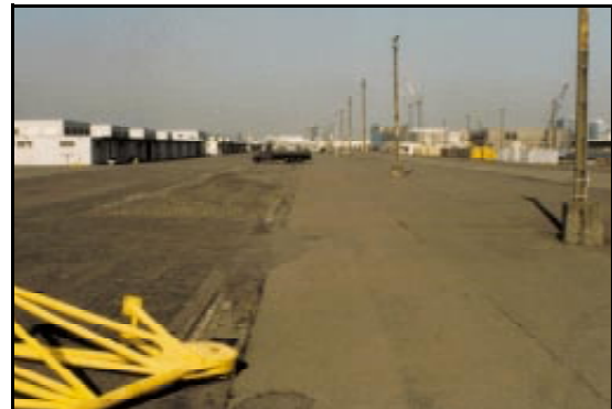
Open Staging at Berth H
