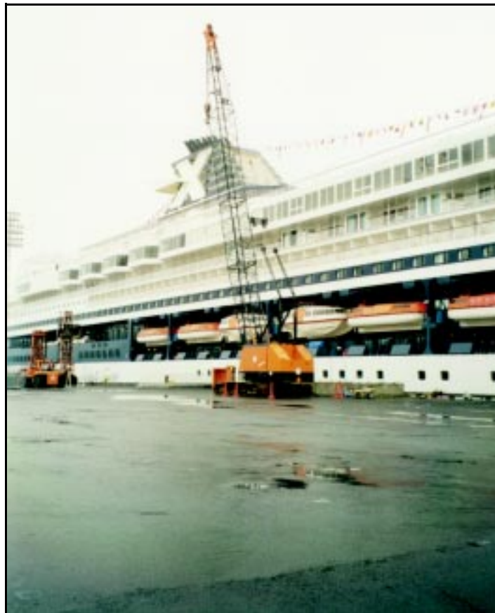
150-Ton Mobile Crawler Crane at ARRC Dock
