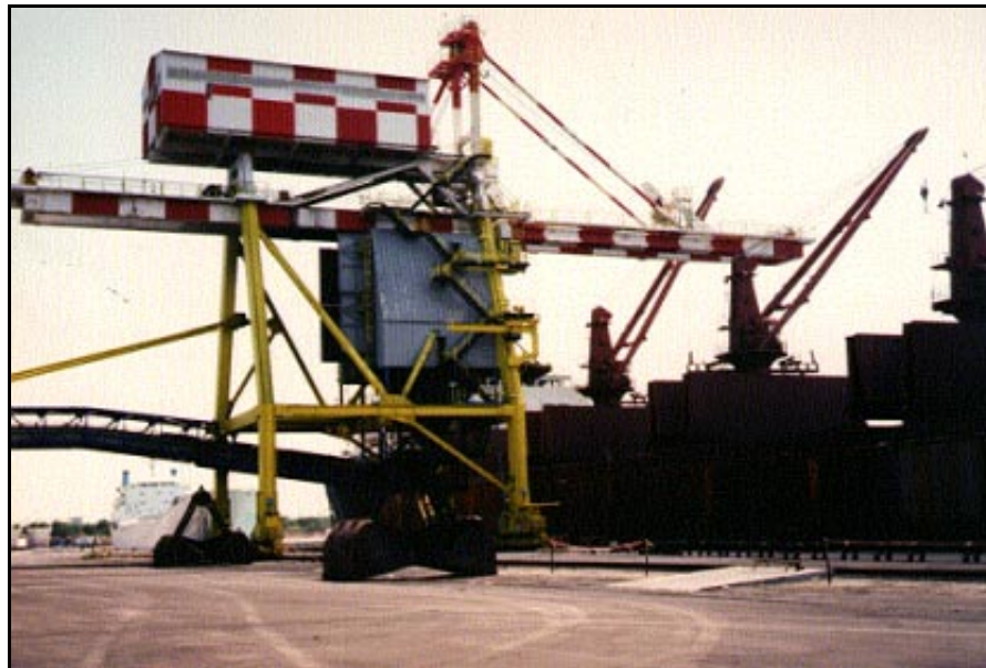
Port of Brindisi Costa Morena Terminal
