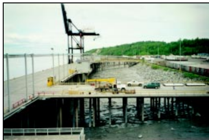
Access to Over-the-Water Wharf (port at low tide)
