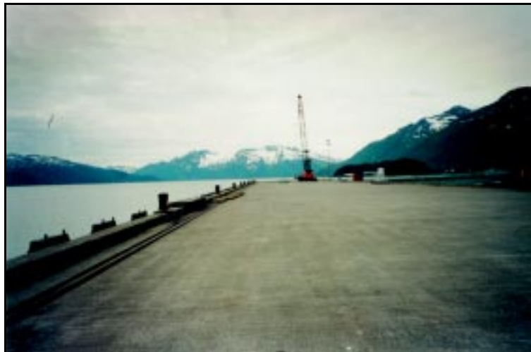
Container Terminal Wharf
