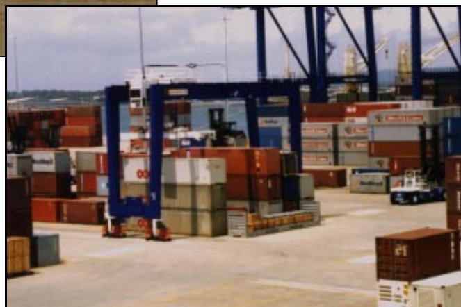
Container Cranes and Transtainer at Manzanillo
