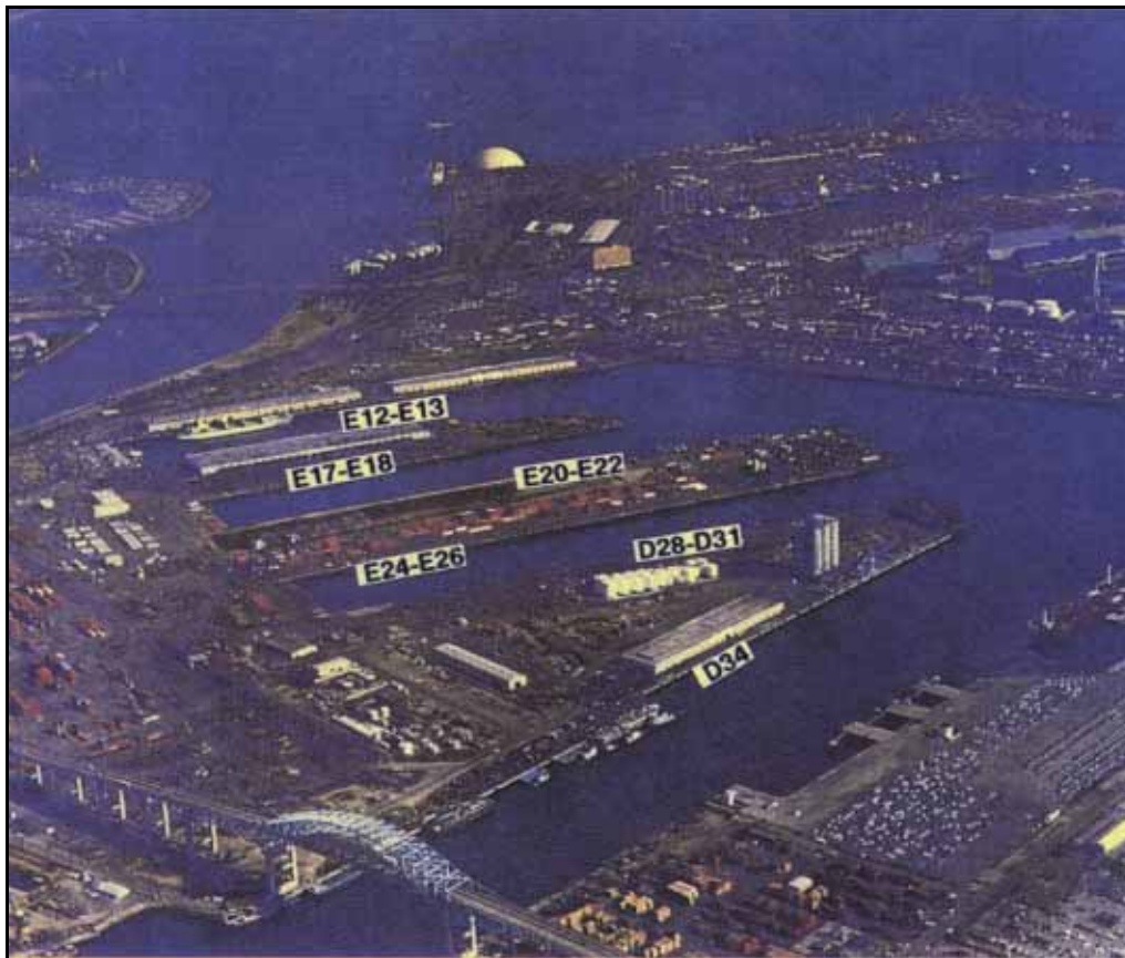
Piers D and E Terminal (Eastward View)
