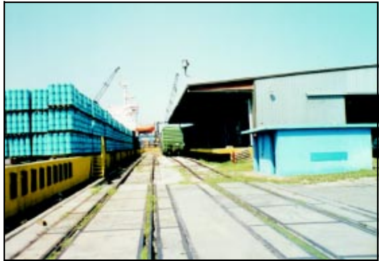
Fixed End Ramp Serving 700-Foot Long Double Tracks
