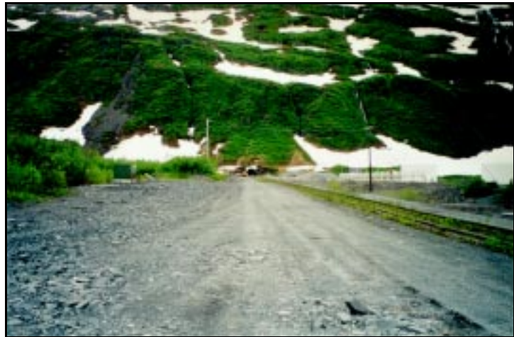
Anton Anderson Railroad Tunnel at Whittier
