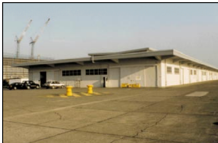
Transit Shed, Building 503
