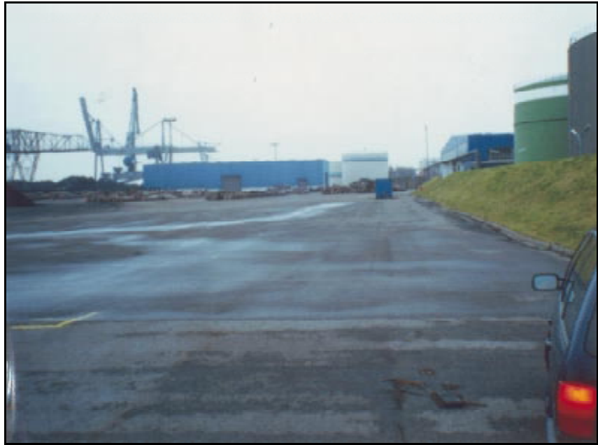
Open Staging Area
