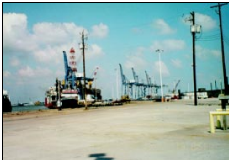
Pier 10 at the Port of Galveston
