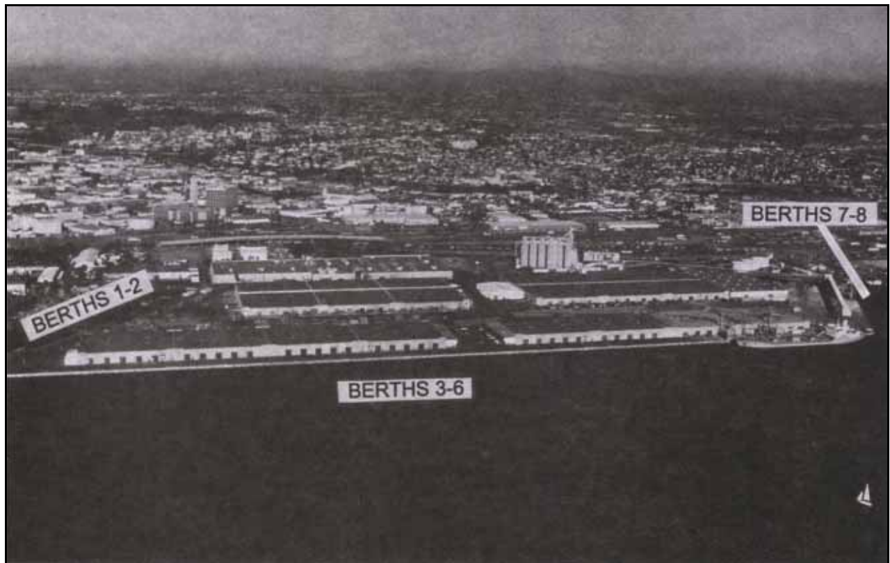
Figure 1. Aerial view of 10th Avenue Terminal
