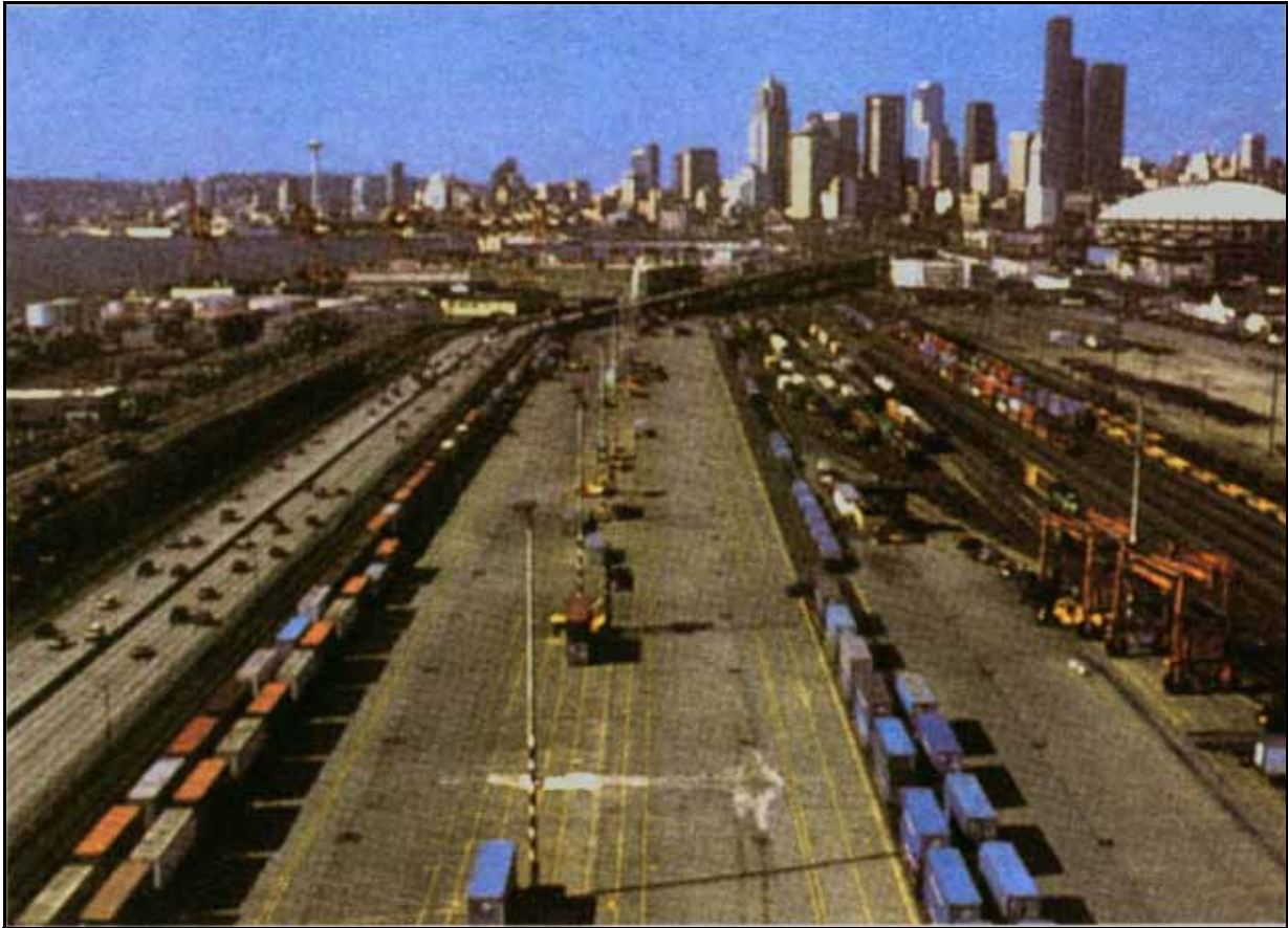
Burlington Northern Intermodal Railyard
