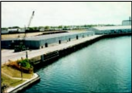
Berths 10 and 11 Turning Basin Terminal
