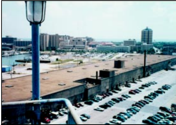
Covered Staging Area at Pier 10 Transit Shed
