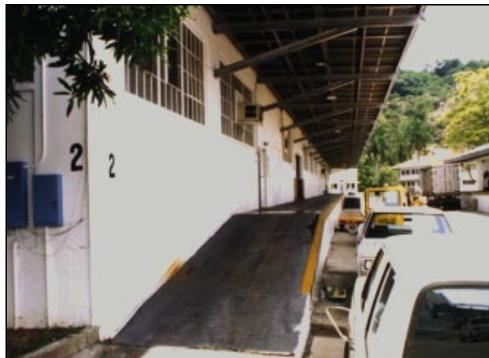
Building 2 - Main Warehouse (north dock)
