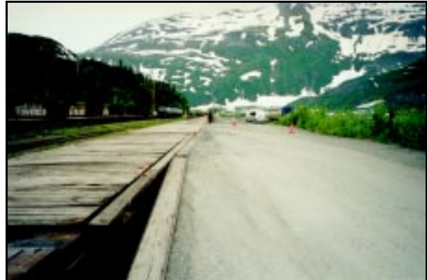
Close Tolerance Between Railcar and Side Ramp at the Port of Whittier
