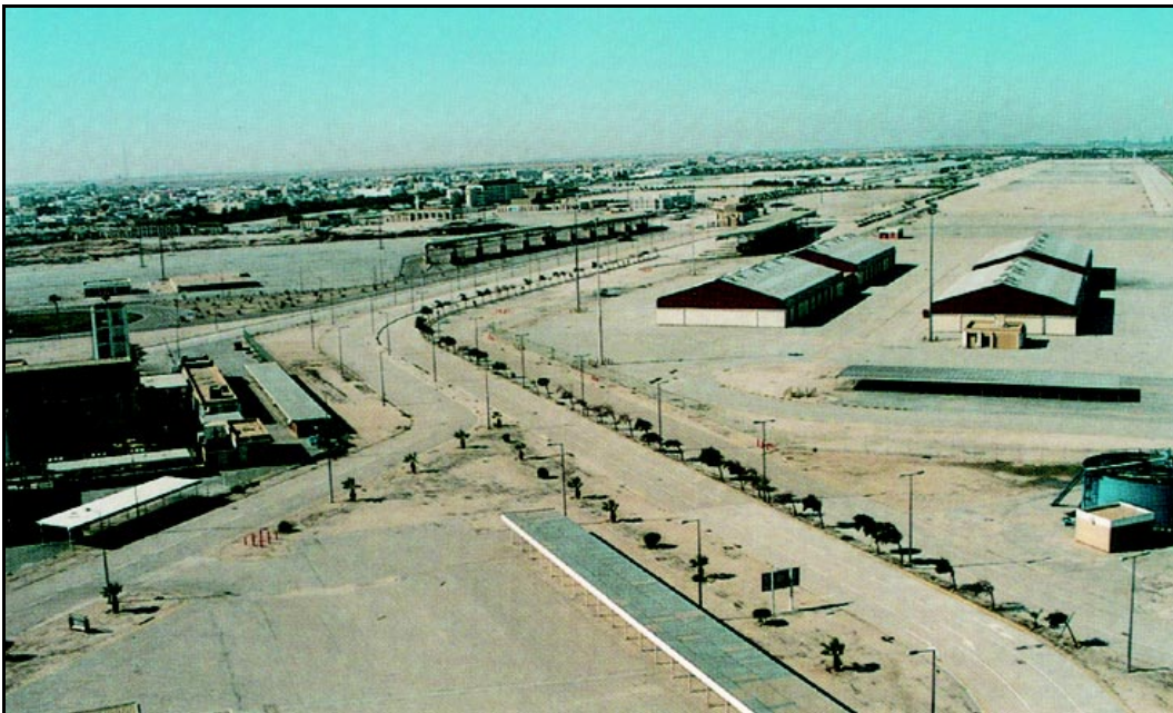
Open Staging at the Port of Jubail
