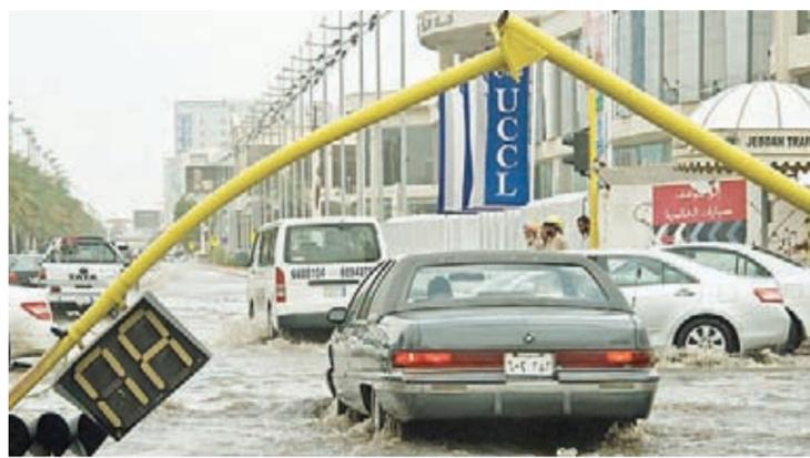
Like a triumphal arch, this traffic light, uprooted by the combination of rain loosening the foundations and high wind tearing at it, lies across a road in Jeddah. (AP)
