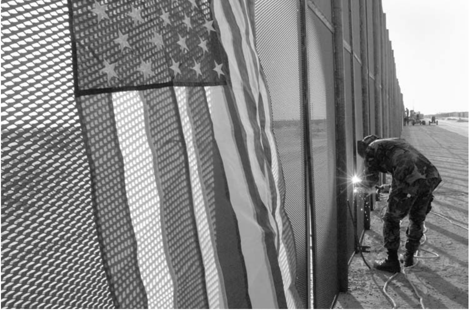
A U.S. Air Force serviceman welds together border-fence panels along the U.S.-Mexican border in Yuma, Arizona, April 24, 2007. (USAF Photo/Senior Airman John Hughel Jr.)
