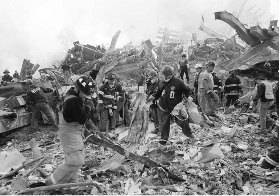
Firefighters and emergency personnel remove debris from the site of the World Trade Center towers on September 13, 2001. (AP/Wide World Photos)
