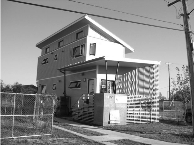
Figure 8.2. Global Green's demonstration house in Holy Cross. More sustainable houses and apartments are planned nearby. Photograph by the author.
