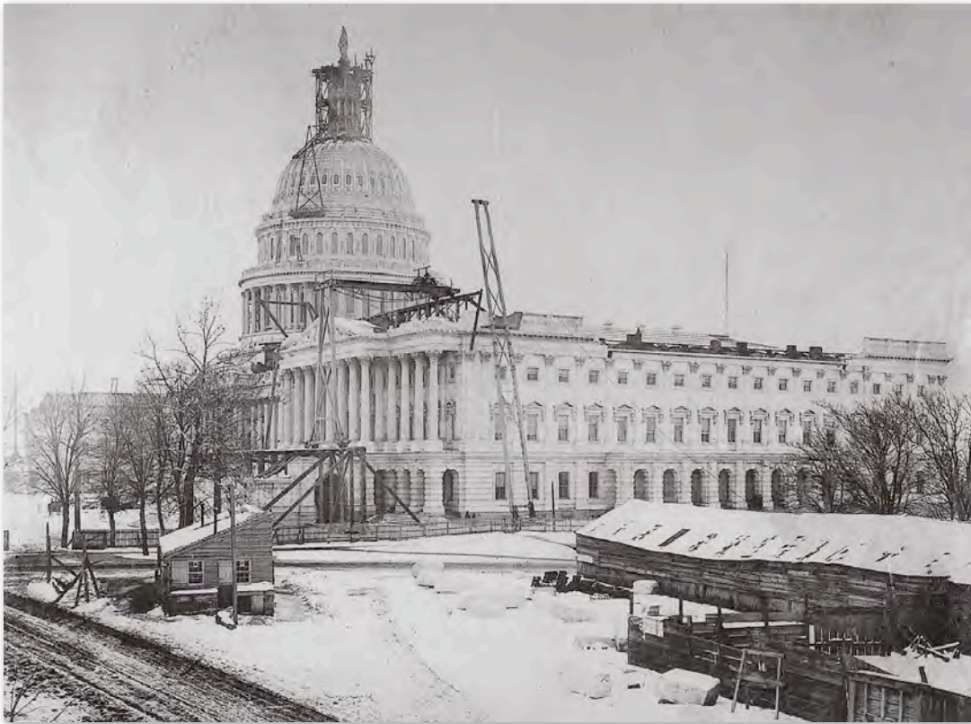
Soon after Freedom was mounted on top of the dome, the scaffold was removed. Capitol, looking Southwest, 1863.
