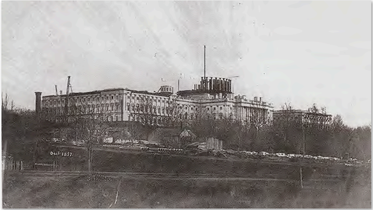
Dome construction, 1857 (top) and 1858 (below). Note the columns.
