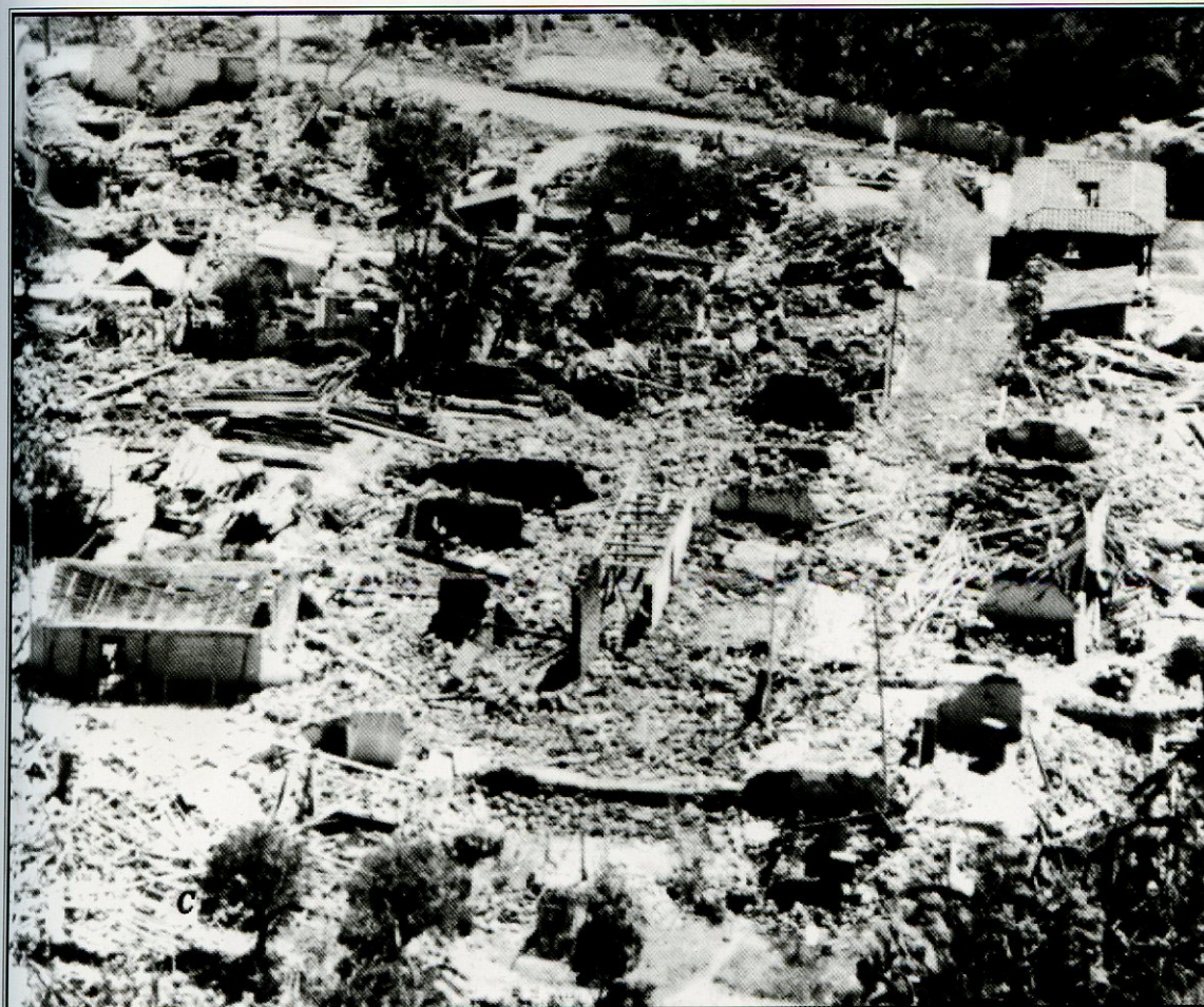
(Left) Devastated outer habs, Bal Prime.
