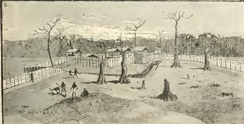
1. Exterior View of Fort Bodo ("Fort Peace") at Ikwiri, commanded by Lieutenant Stearns, U.S.A. 2. Stockade of the Enclosure, or "Boma," constructed of boards fixed between pairs of upright poles, and tied with ropes of vine.
