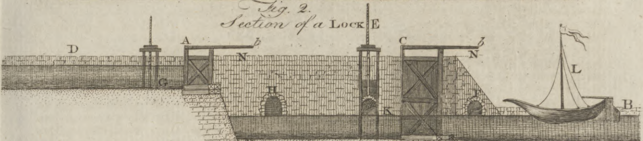
Fig. 3. Section of a Lock full of Water
