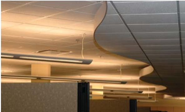
Modern Ceiling Detail
