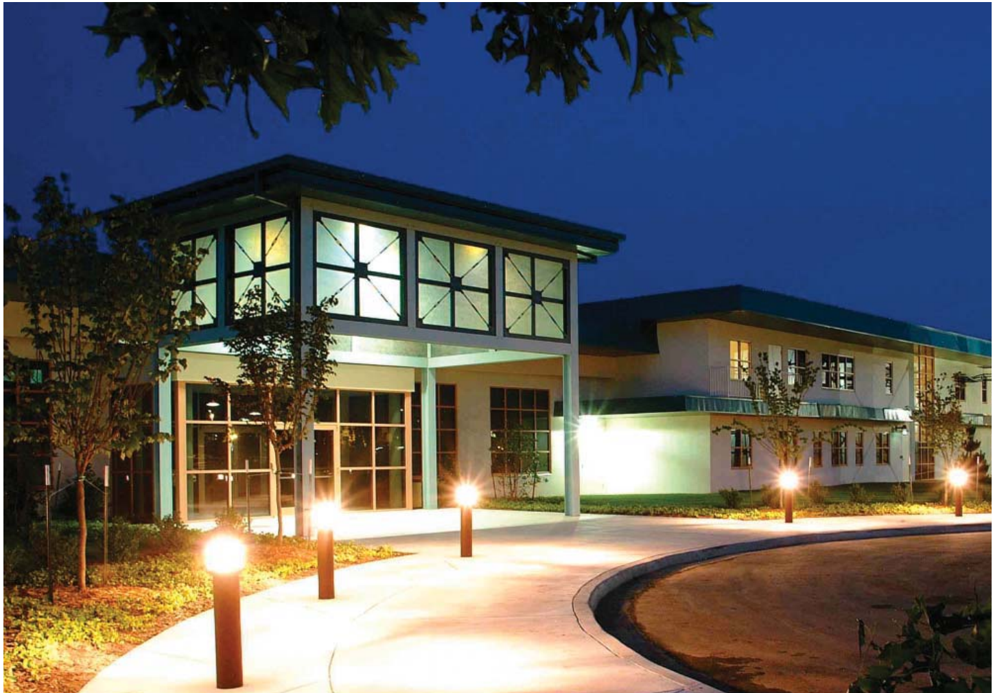
View of Renovation and New Entry Piece
