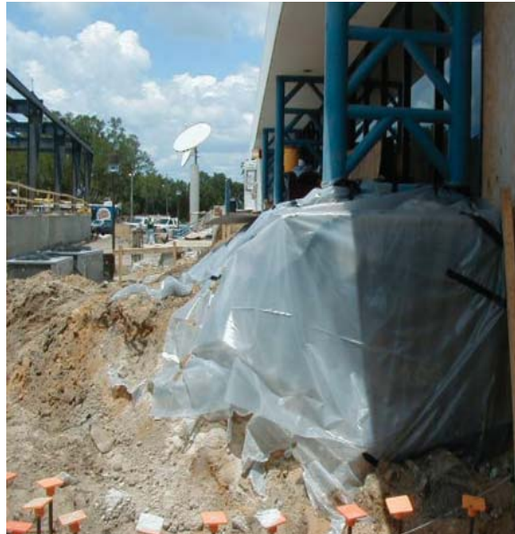
Construction Cox Radio Orlando
