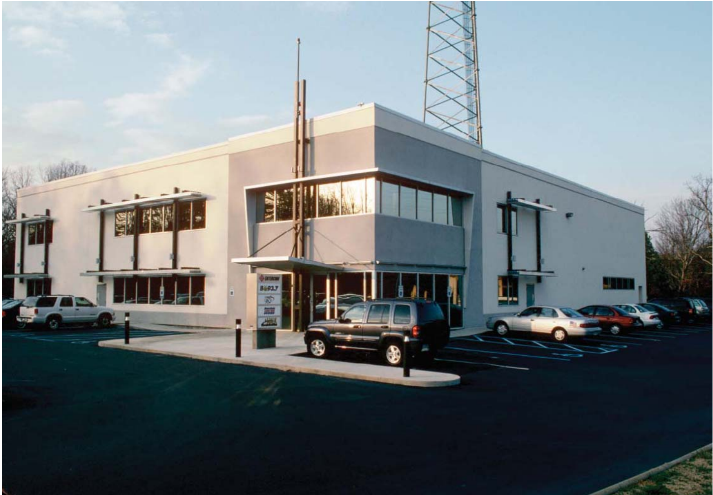
New Facility: Main Entry Renovation
