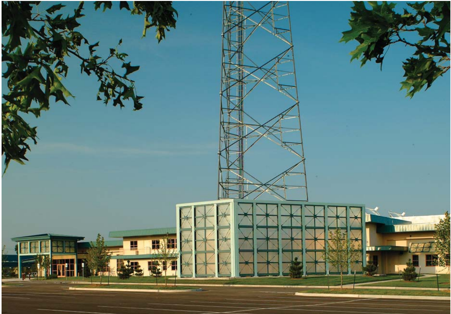
Station Addition Clear Channel Communications Tulsa
