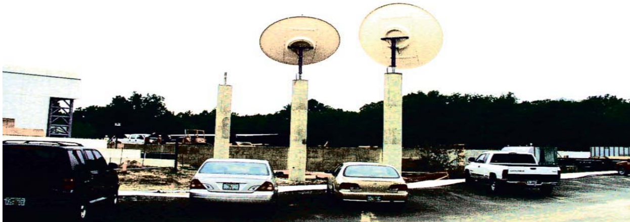
Construction Cox Radio Orlando
