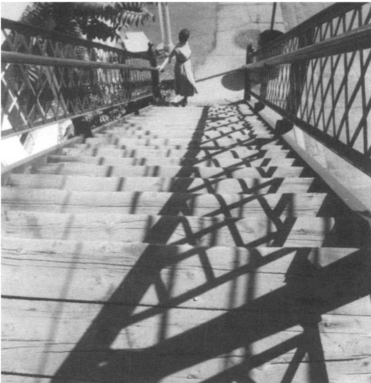
FIG. 2.3. Aurora climbing stairs of railroad bridge.
