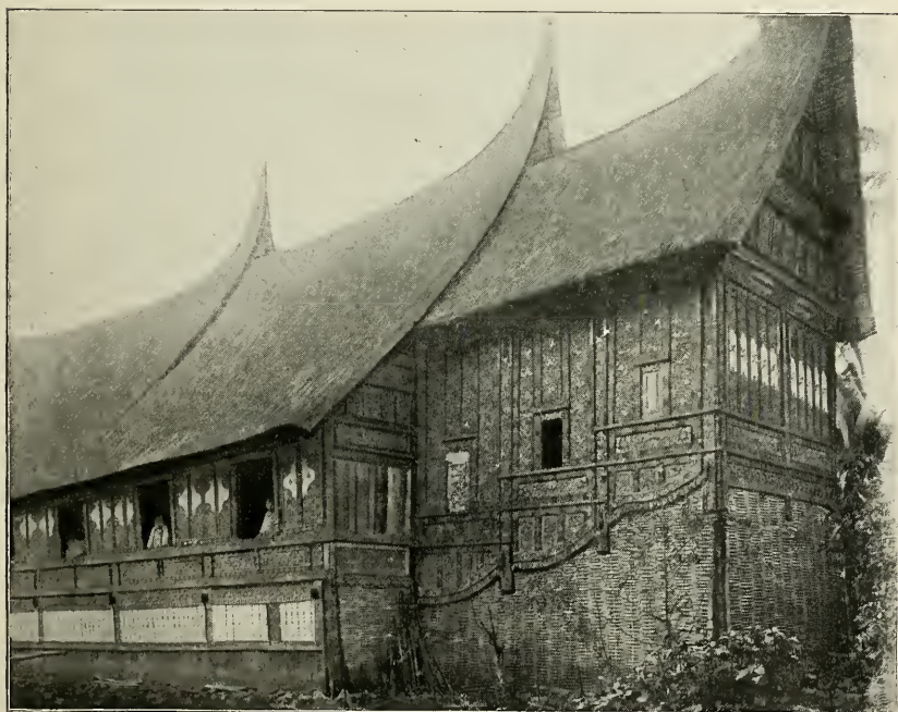
SUMATRAN DWELLING-HOUSE, SHOWING BAMBOO WICKERWORK AND ELABORATE CARVING AND PANELING
