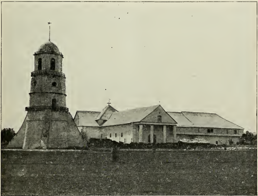
CHURCH, CONVENTO, AND WATCH TOWER — DUMAGUETE, NEGROS ISLAND
