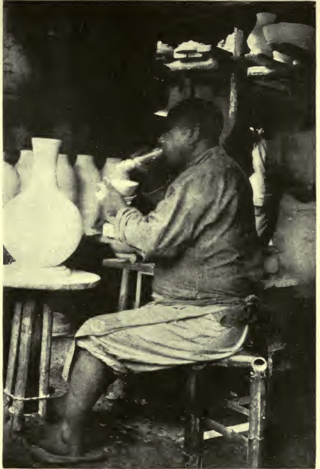
ONE METHOD OF APPLYING PORCELAIN GLAZE
