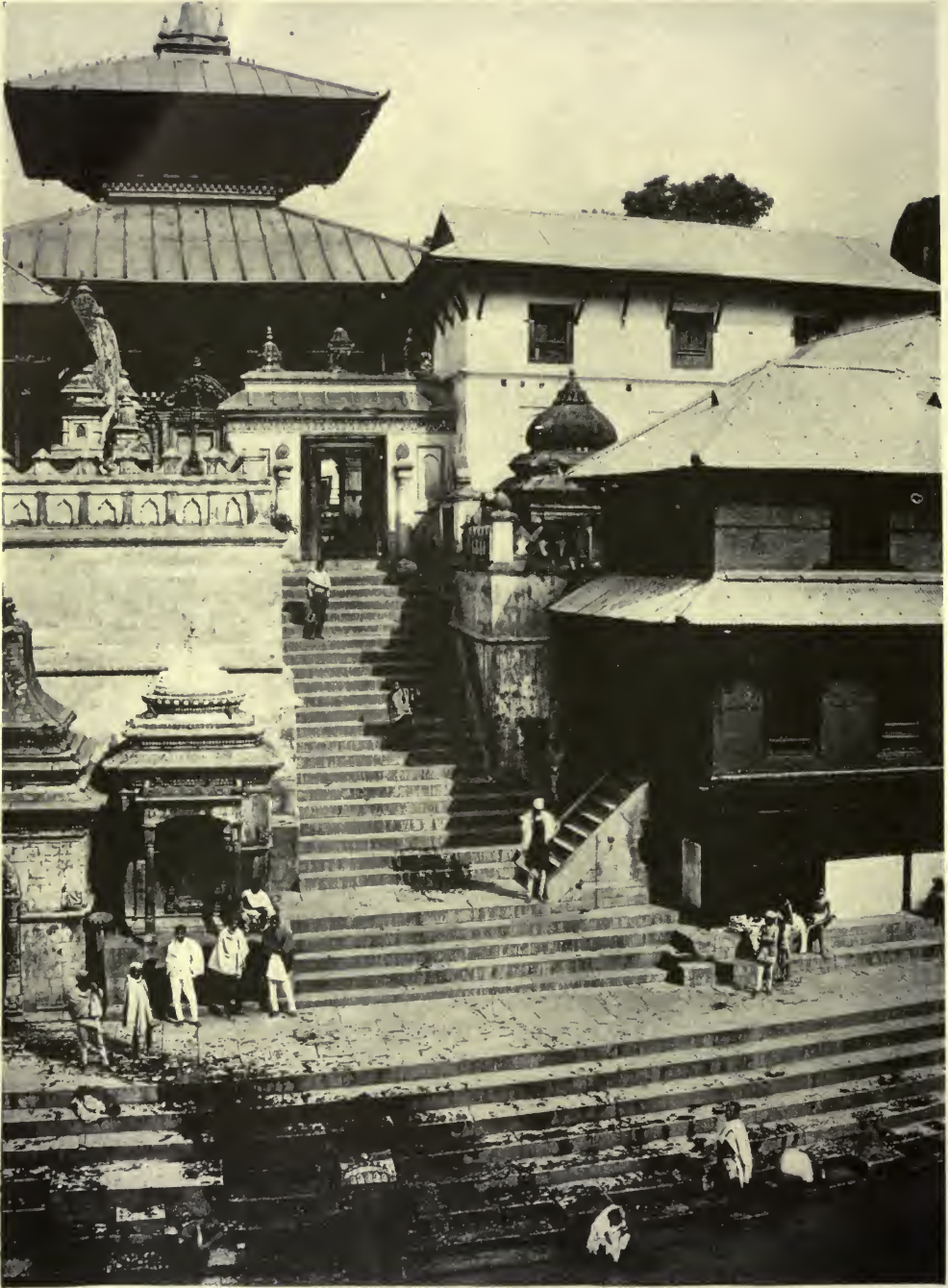
STEPS LEADING FROM THE HOLY BAGHMUTTI RIVER TO THE TEMPLE AT PASHPATI
