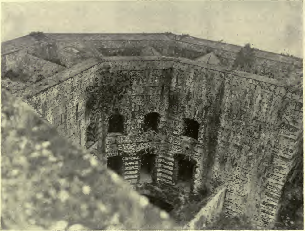
LOOKING DOWN INTO A SUNKEN COURT AT THE NORTHWEST CORNER OF CHRISTOPHE'S CITADEL
