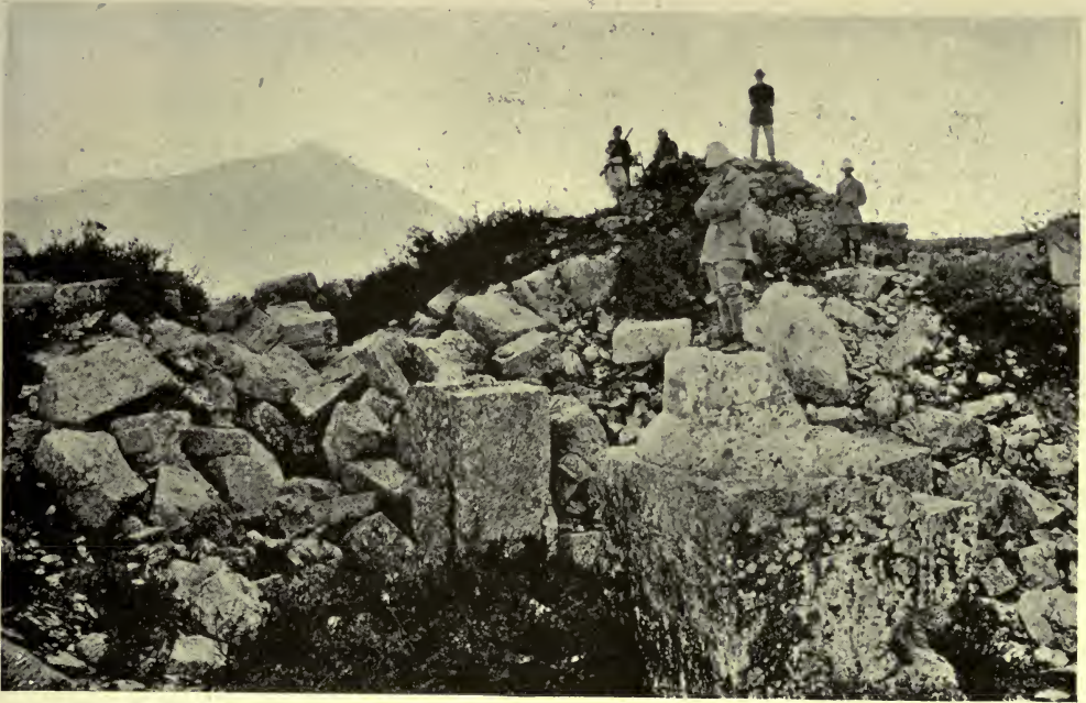
RUINS OF A CHURCH ON "JABEL SIMAN," PROBABLY THE BIRTHPLACE OF THE ORDER OF PILLAR SAINTS
