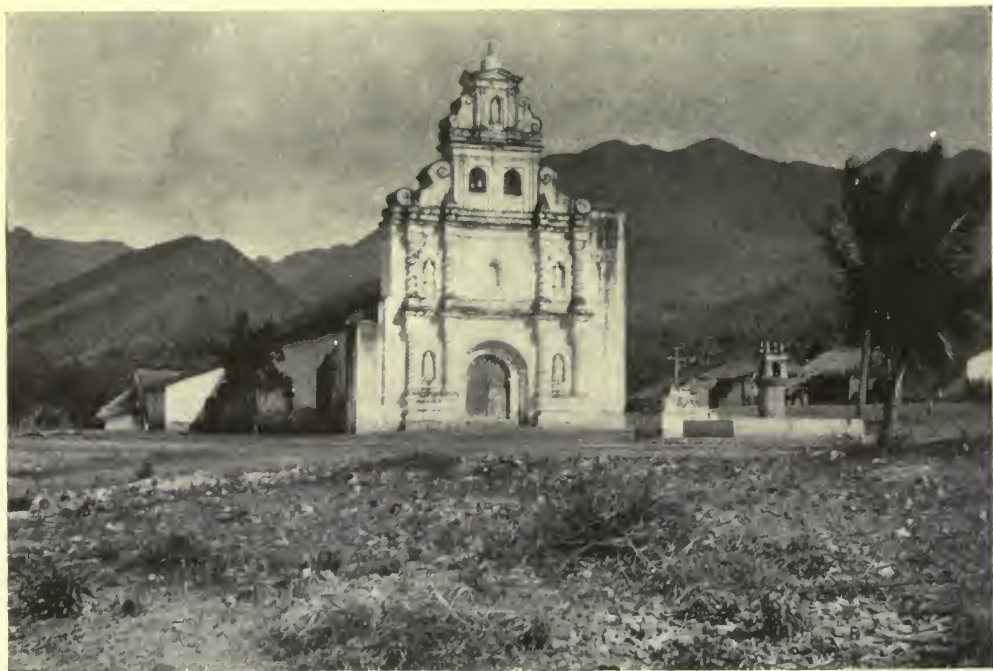
A CHURCH AT CAMOTAN, GUATEMALA, ON THE ROAD TO THE ANCIENT MAYAN CITY OF COPAN
