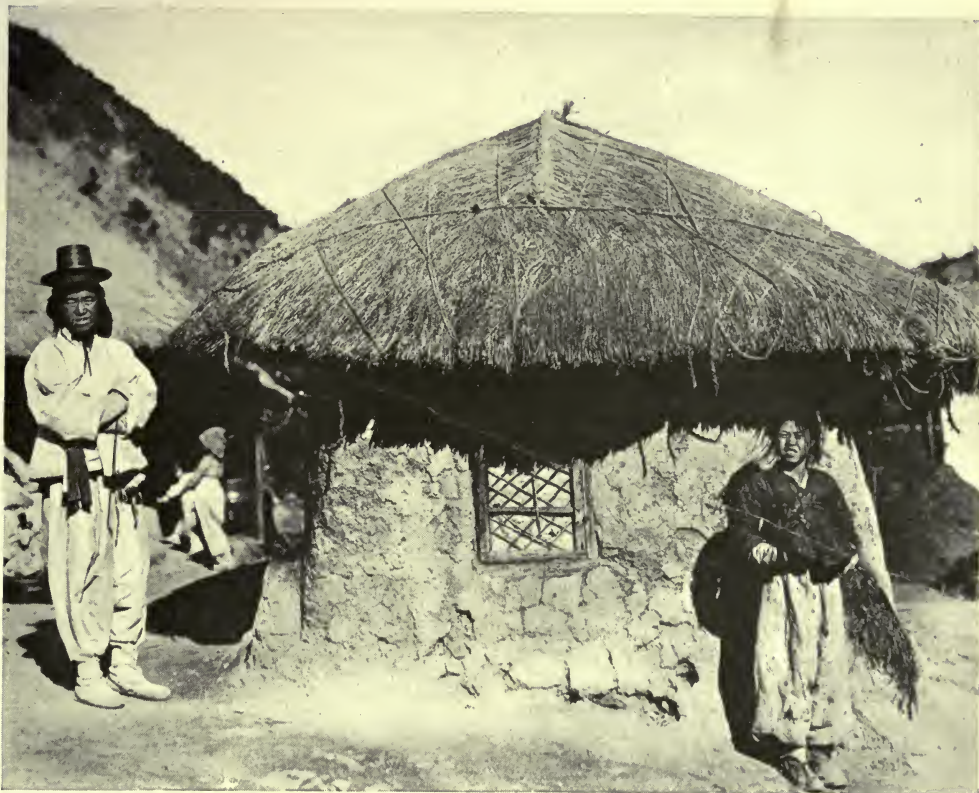
THE WALLS AND FLOOR OF THIS TYPICAL, NORTHERN KOREA HOUSE ARE MADE OF CLAY; THE THATCH IS OF RICE STRAW
