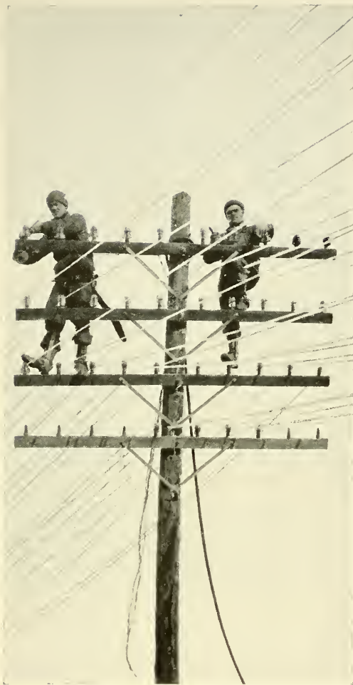
REPAIRING THE DAMAGE DONE BY SNOW AND SLEET
