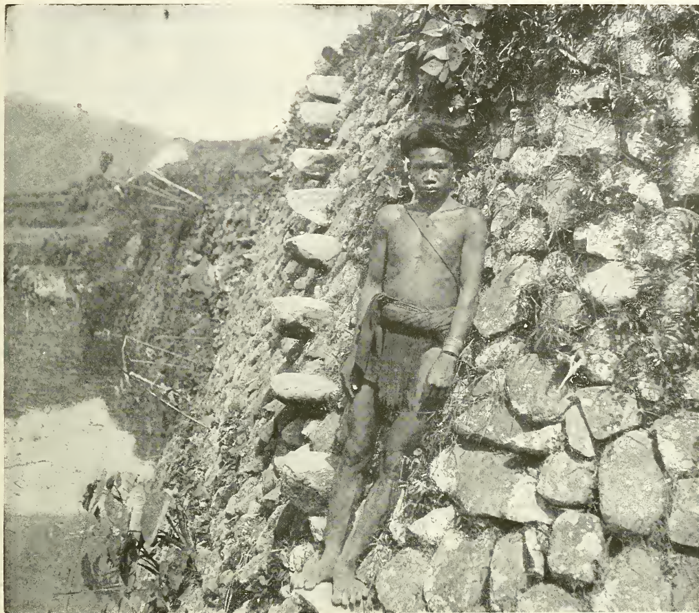
A TYPICAL IFUGAO RICE PADDY WALL, SHOWING STEPS USED IN ASCENDING TO TERRACES ABOVE (SEE PAGE 882)
