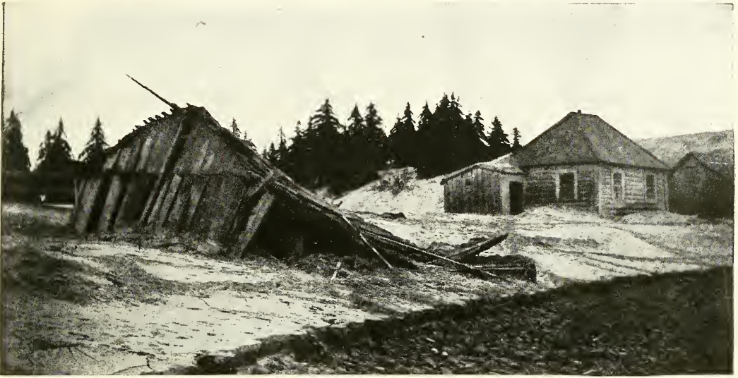
FRAME STRUCTURE, CRUSHED BY WEIGHT OF ASHES
