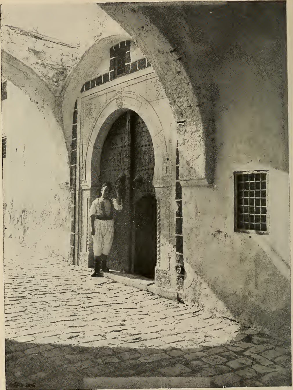
ENTRANCE TO ARAB HOUSE: TUNIS
