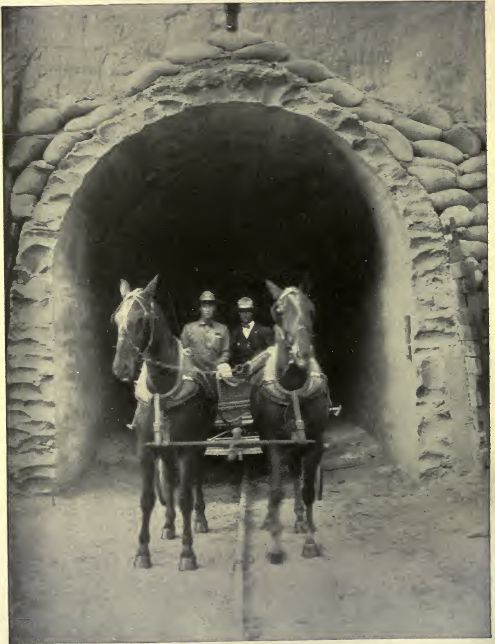
ONE OF THE AQUEDUCT TUNNELS
