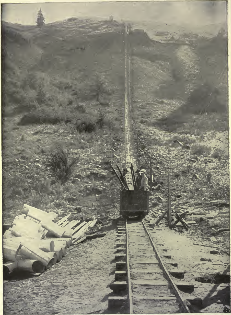
TRAMWAY IN THE TIETON CANYON AT CAMP NO. 1: YAKIMA PROJECT, WASHINGTON
