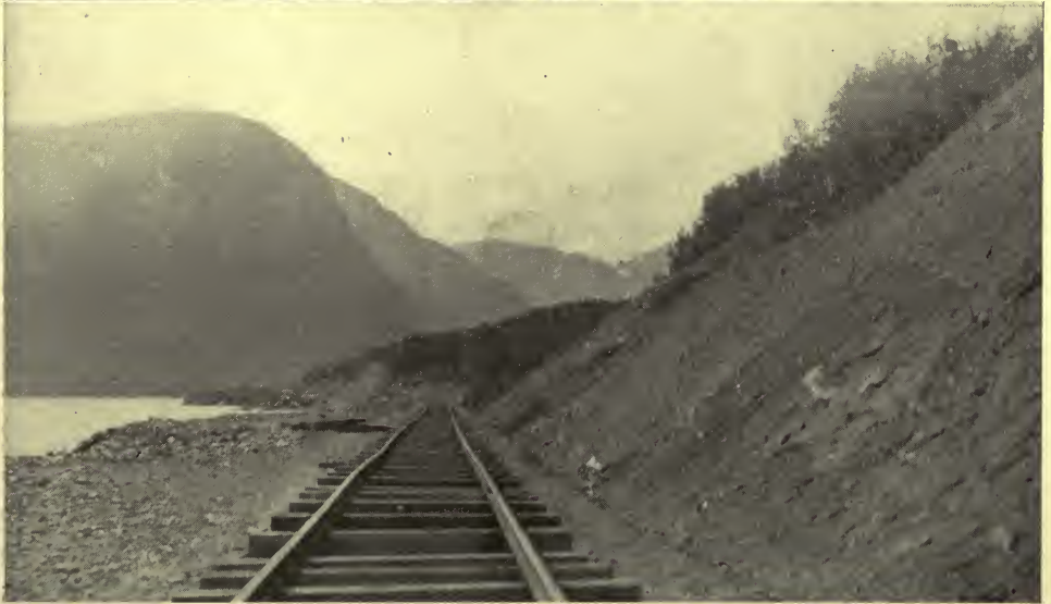
A SHARP CURVE IN THE RAILWAY AT ABERCROMBIE RAPIDS: A NARROW SHELF BLASTED OUT FOR THE ROAD
