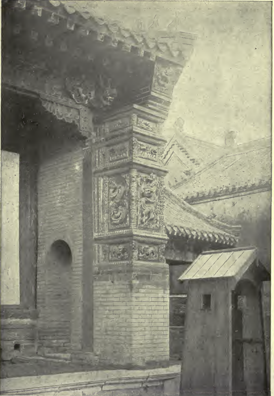
DETAIL OF GATE-HOUSE OF IMPERIAL PALACE: GREEN FAIENCE DRAGON PANELS ON BRICK COLUMNS (SEE PAGE 305)
