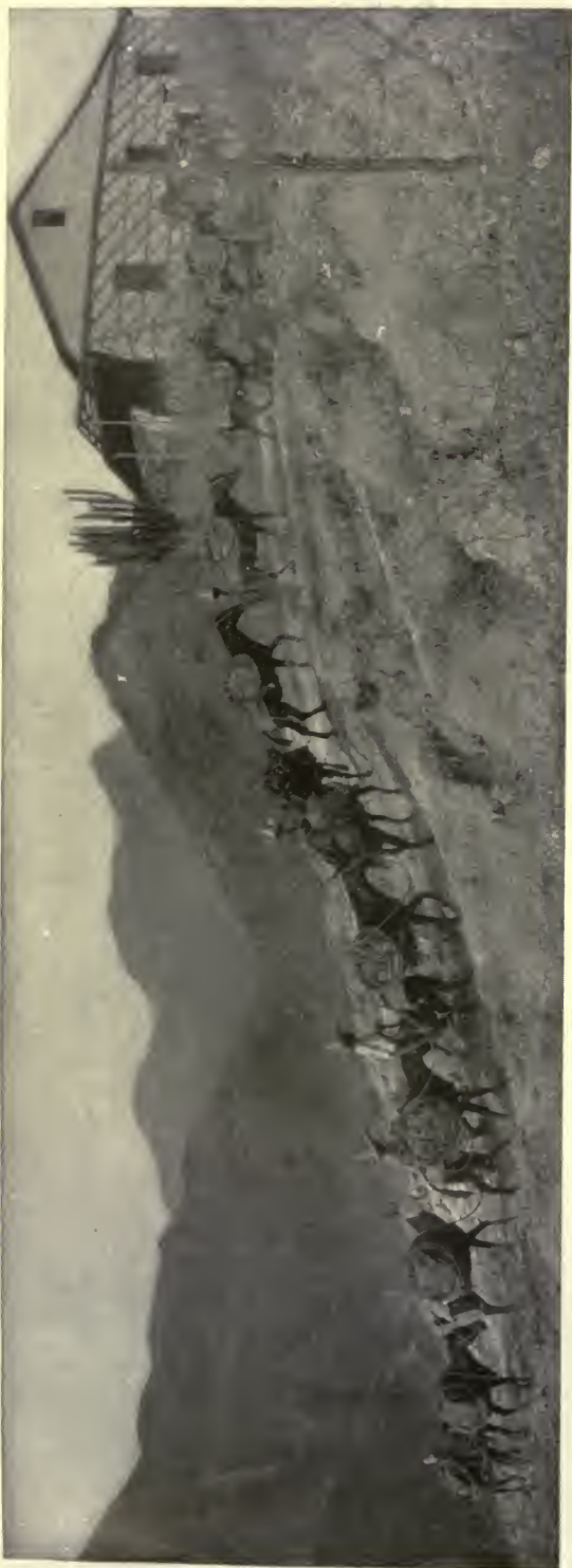
PICTURE 10. CARRYING 2,300 FEET OF \frac{7}{8} STEEL AERIAL TRAMWAY CABLE ON 12 MULES (SEE PAGE 990)
