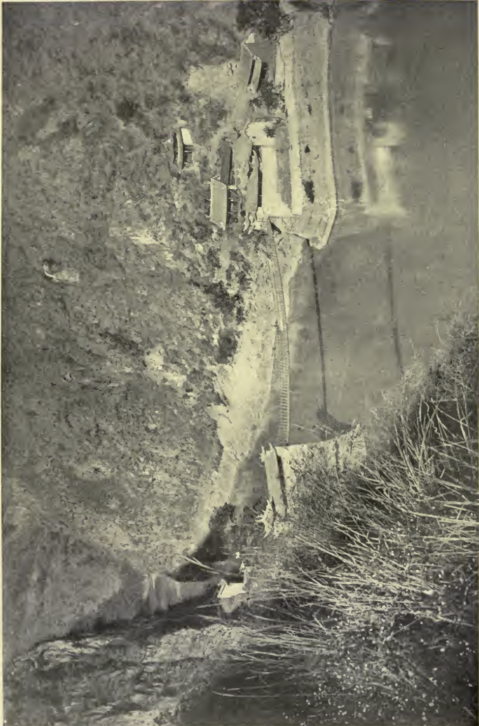
SUSPENSION CHAIN BRIDGE ON THE MEKONG RIVER, ON THE MAIN TRADE ROUTE FROM UPPER BURMA TO YUNNAN It is formed of 12 iron chains and plank roadway 8 feet wide. Breadth of span, 70 yards
