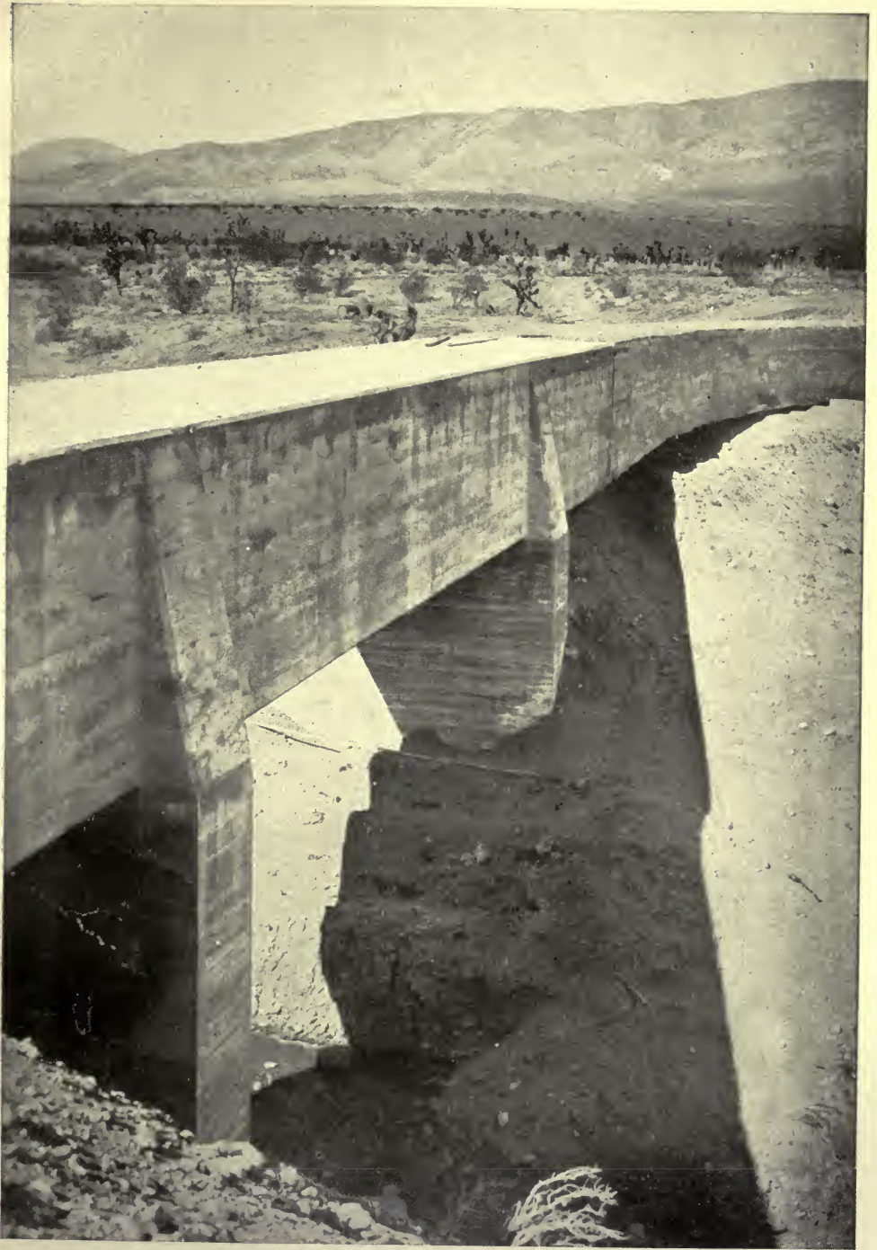
THE AQUEDUCT SPANS SMALL DESERT WASHES BY RECTANGULAR CONCRETE CULVERTS
