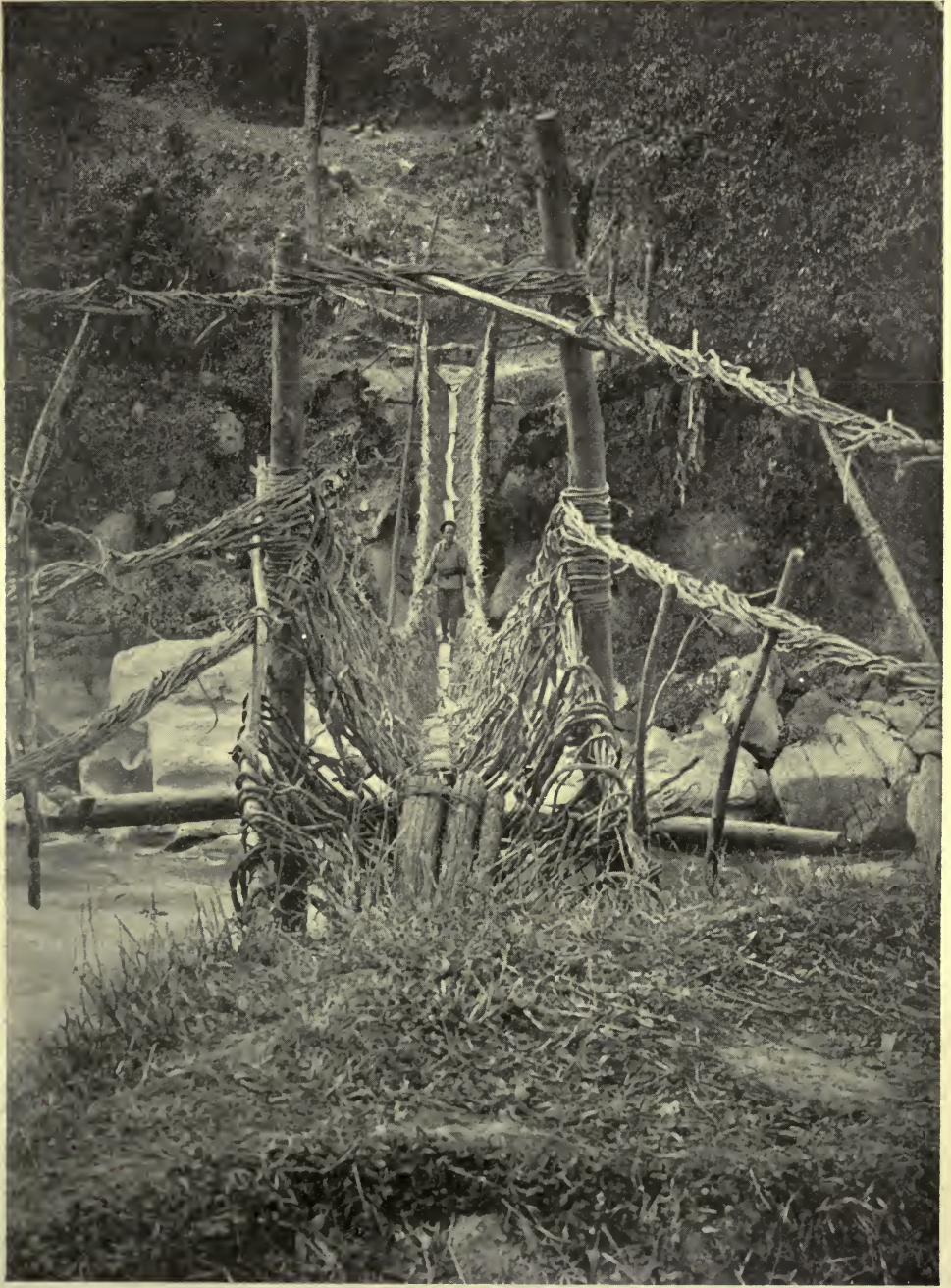
ANOTHER TYPE OF LIANA BRIDGE IN THE LAND OF THE CROSSBOW, SHOWING APPROACHES AND FASTENINGS
