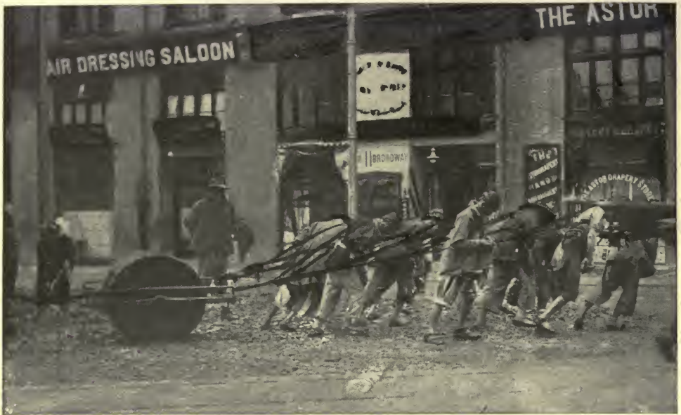
A STEAM ROLLER IN THE AMERICAN SETTLEMENT AT SHANGHAI
