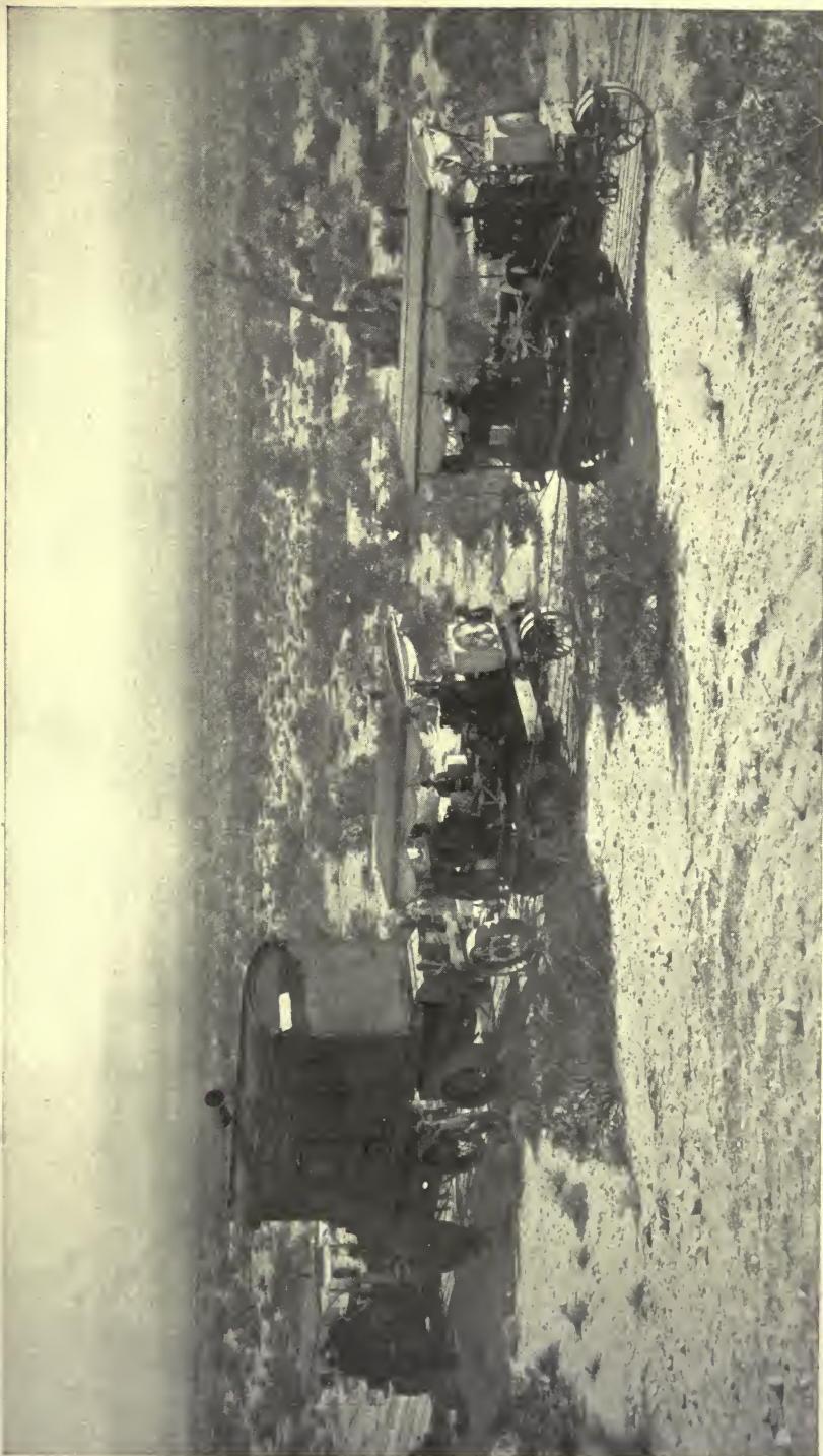
TWO CATERPILLAR TRACTION ENGINES COUPLED TOGETHER AND HAULING ONE OF THE BIG POWER-SHOVELS INTO THE DESERT, WHERE IT IS TO BE PLACED AT TRENCH EXCAVATION
