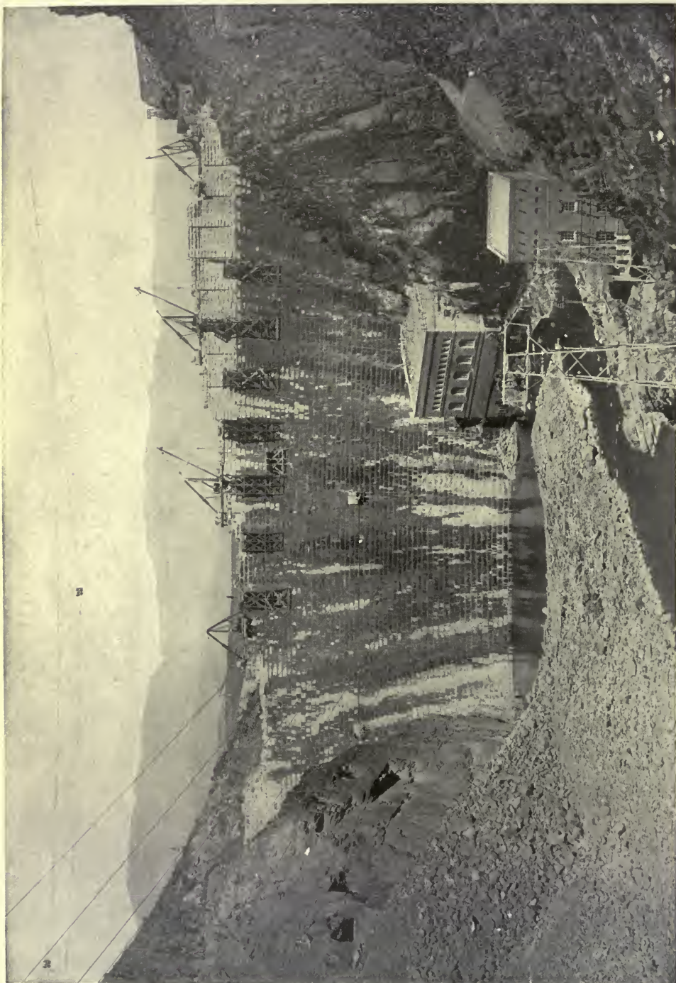
THE ROOSEVELT DAM : TYPE RUBBLE MASONRY ARCH GRAVITY (SEE PAGE 360)
