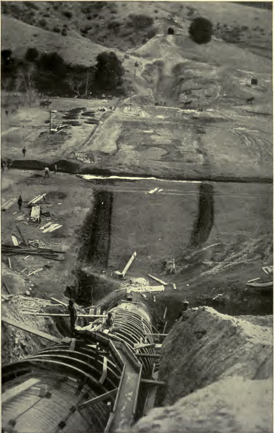
BUILDING AN INVERTED SIPHON ACROSS WHITNEY CANYON TO CARRY THE WATER DOWN ONE SIDE AND UP THE OTHER (SEE PAGE 574)
