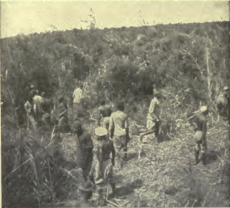
SUDD-CLEARING STEAMER TEARING OUT THE OBSTRUCTION WITH STEEL CABLES THE TOP OF A SUDD GROWTH REMOVED AND READY TO BE PULLED TO PIECES TO CLEAR THE CHANNEL
