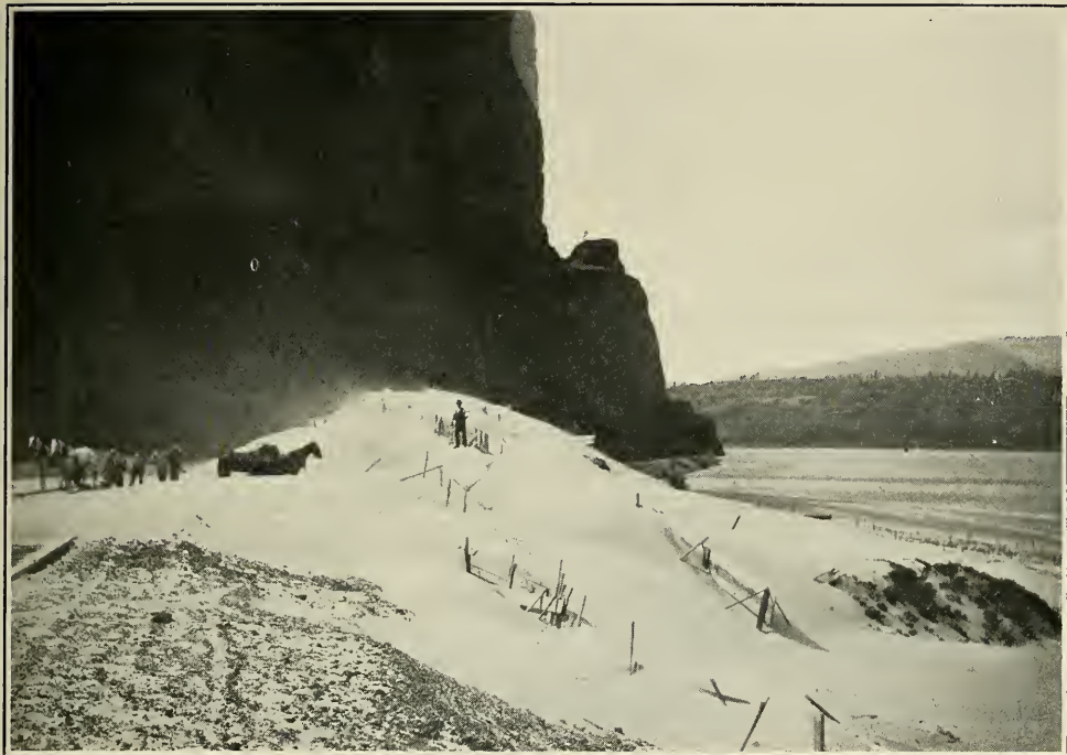
Sand Dune Encroaching on Railroad, Near The Dalles, Oreg.
