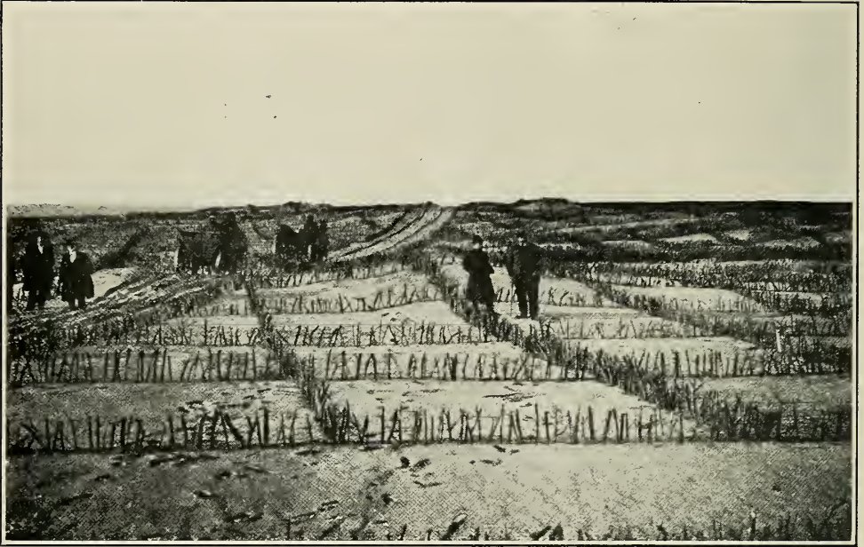
Sand Dunes Controlled by a Covering of Sand Hedges, on the Kurische Nehrung, Northeastern Prussia
