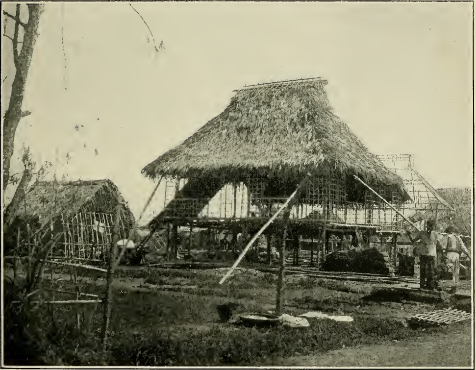
Nipa House Under Construction
