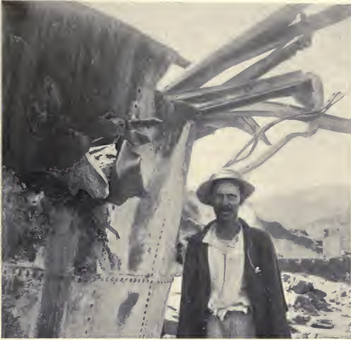
St Pierre. — Near view of one of the holes. The material of the tanks is quarter-inch boiler iron (see page 425)
