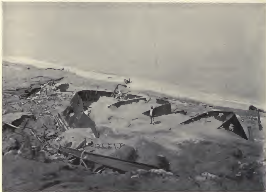
St Pierre. Ruins of the Great Distillery in the Fort Quarter of the City, Showing Holes in the Iron Tanks due to Volcanic Bombardment
