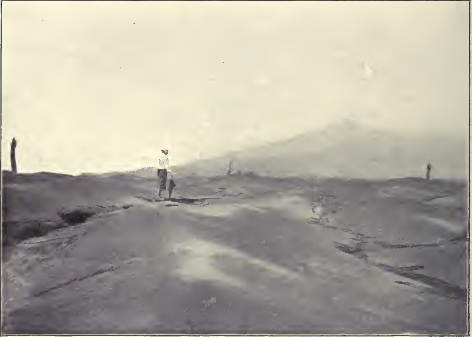
Richmond Estate, St Vincent, May 25, 1902
