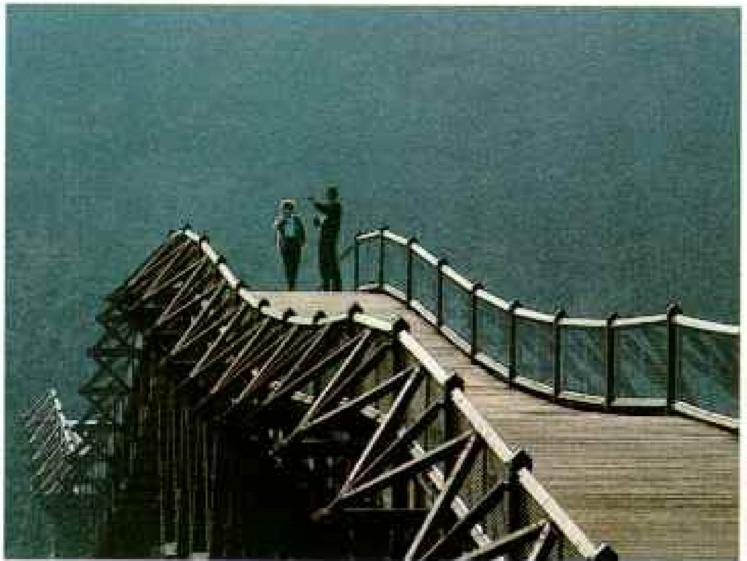
At Essing, planks bonded by glue form a footbridge that undulates like a wave. Bridges in the Altmühl region were architect-designed, and each is different. Seven of the lockhouses built by King Ludwig’s architect were preserved.
