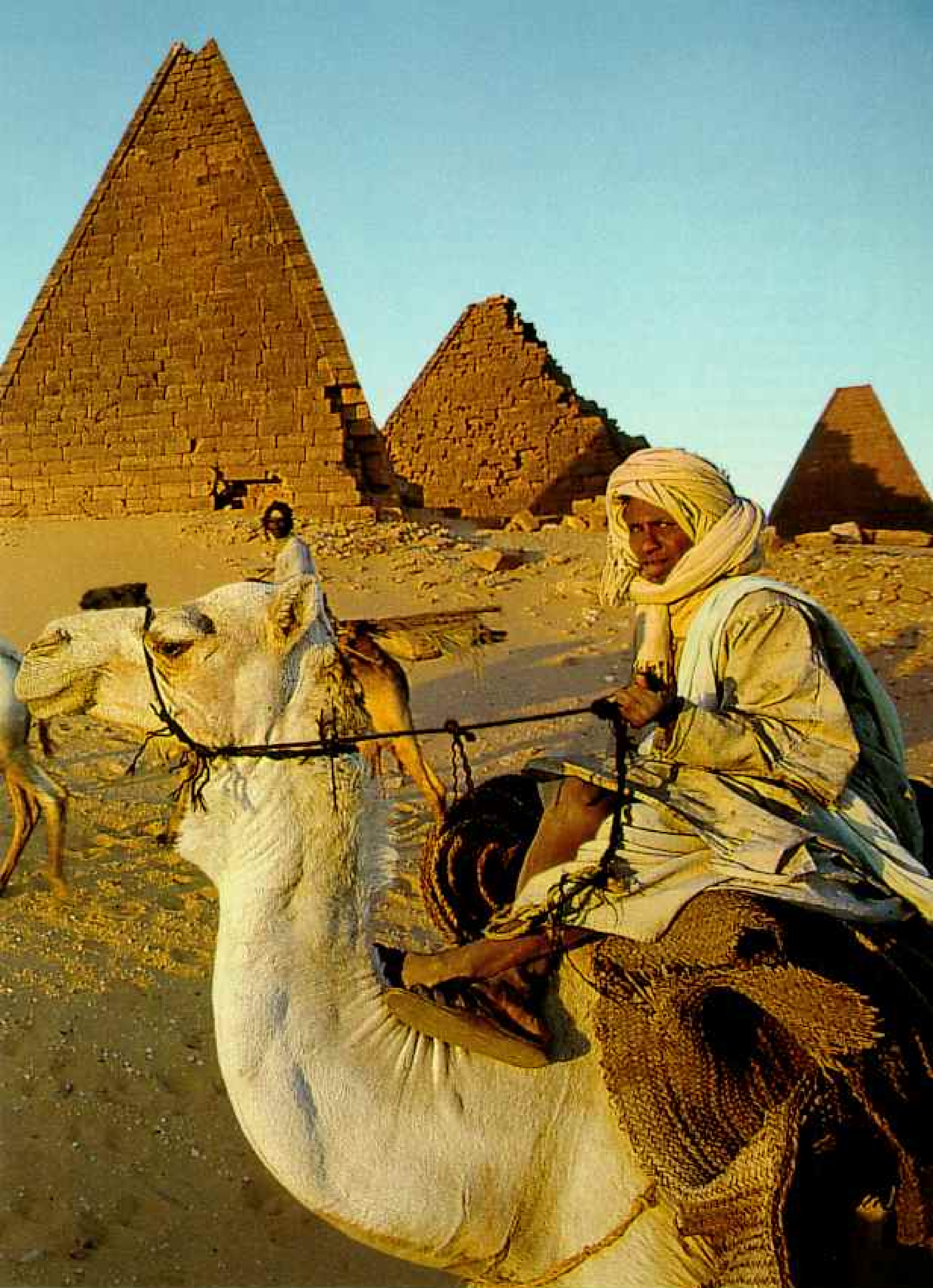
prepared rock-cut burial chambers and capped them with steep-walled pyramids. The stone blocks were raised by a shadoof, a seesaw lift of Egyptian design.
